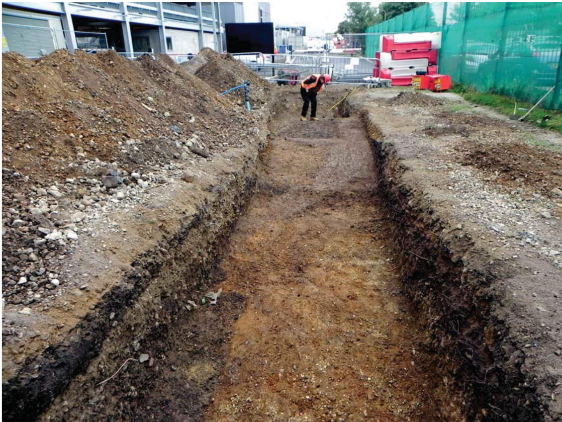
Fig 5 Trench 1, looking south
