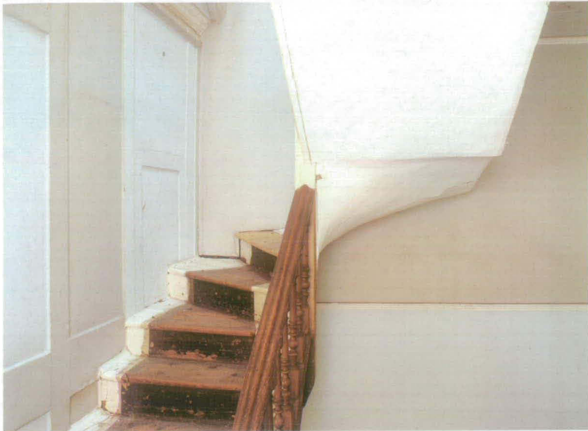
Fig 32 Dog-leg staircase between 2F1 and 3F1, indicating the probable original width of the service stair compartment; looking west from 2F1.
