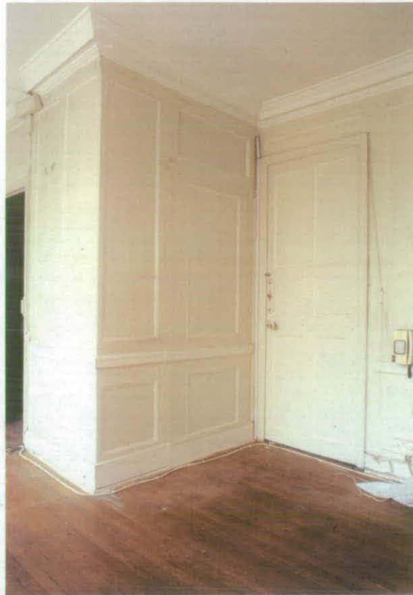
Fig 34 Plain panelling [52] facing 2F2; looking north-west. Room 2F2 was originally divided into two rooms, each entered from 2F1 by a separate door, that to the east being sealed shut when the rooms were later thrown together. Another door to room 2F5 to the north is probably a later insertion
