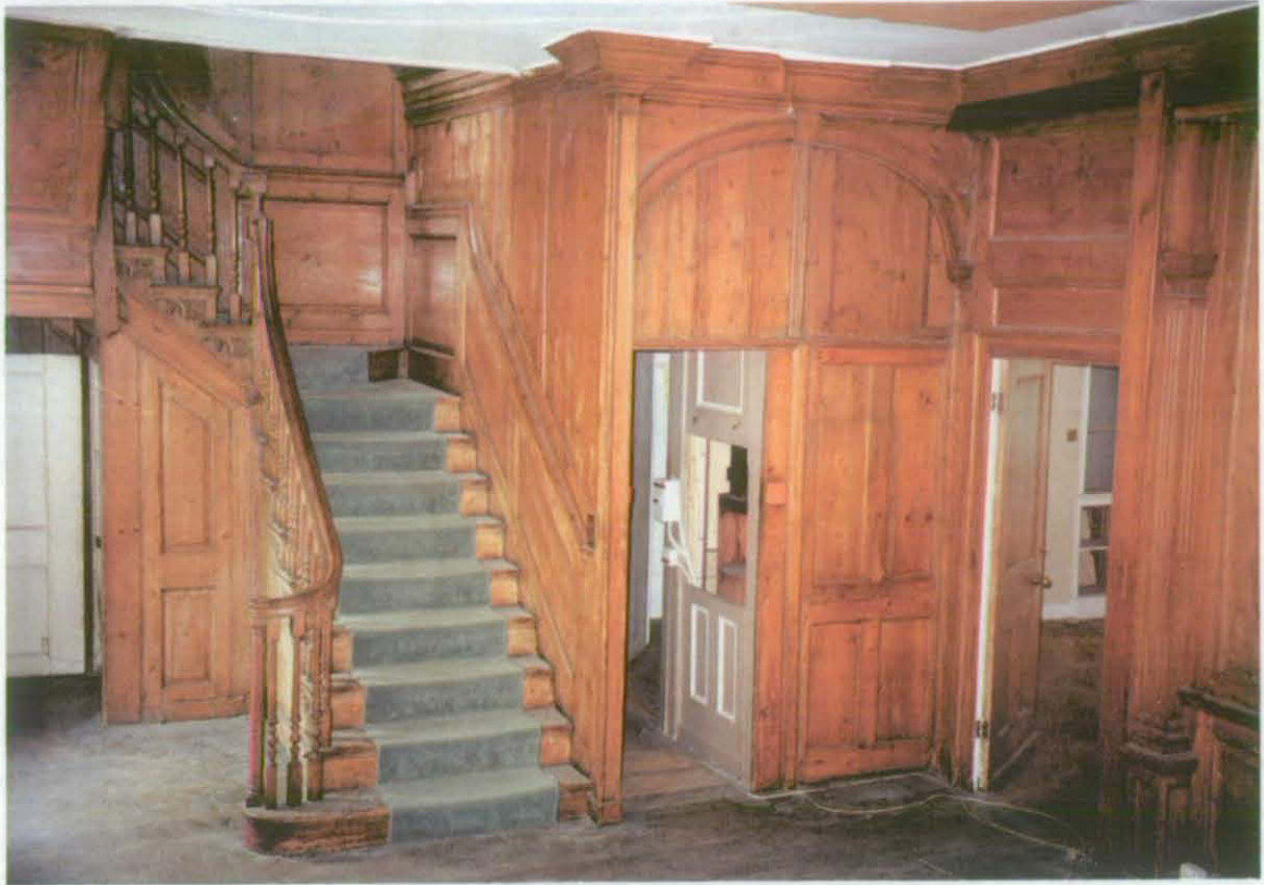
Fig 28 Principal staircase, between G1 and 1F1; looking west
