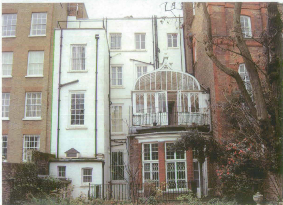
Fig 25 North (rear) front of the house; looking south (A J Browne, Architects)
