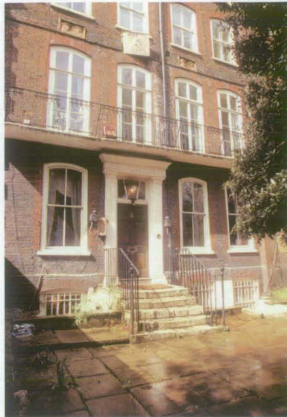
Fig 24 Detail of the south front of house, including garden, door steps and door case, basement area, windows and 1st-floor balcony; looking north-east
