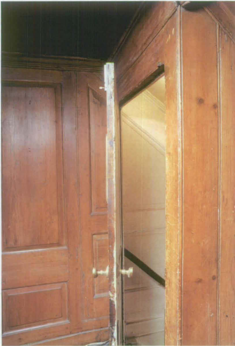
Fig 30 Continuous high quality panelling [10] under the principal staircase on the ground floor, originally intended to be seen and later partially masked by the insertion of a door and staircase down to the basement (the door is ajar to show the panelling); looking north-west
