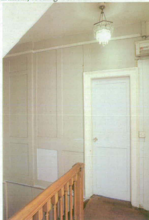
Fig 33 Plain panelling [49] on the south face of chimney breast [25], visible in the north wall of 2F1, and offset panelling [50] and inconsistent door frame [51] to its east, the latter probably inserted later when the service stair compartment was enlarged; looking north-west
