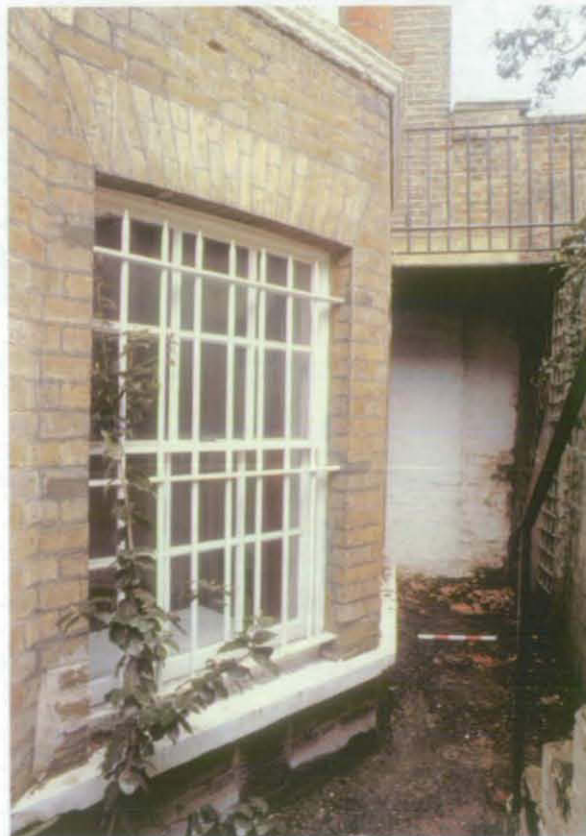
Fig 27 Brick wall [31] running south to north at the north west corner of the rear basement area, B8 (above the scale rod), looking west. The canted bay windows of the rear west wing and its ground-floor bridge to the garden are also shown
