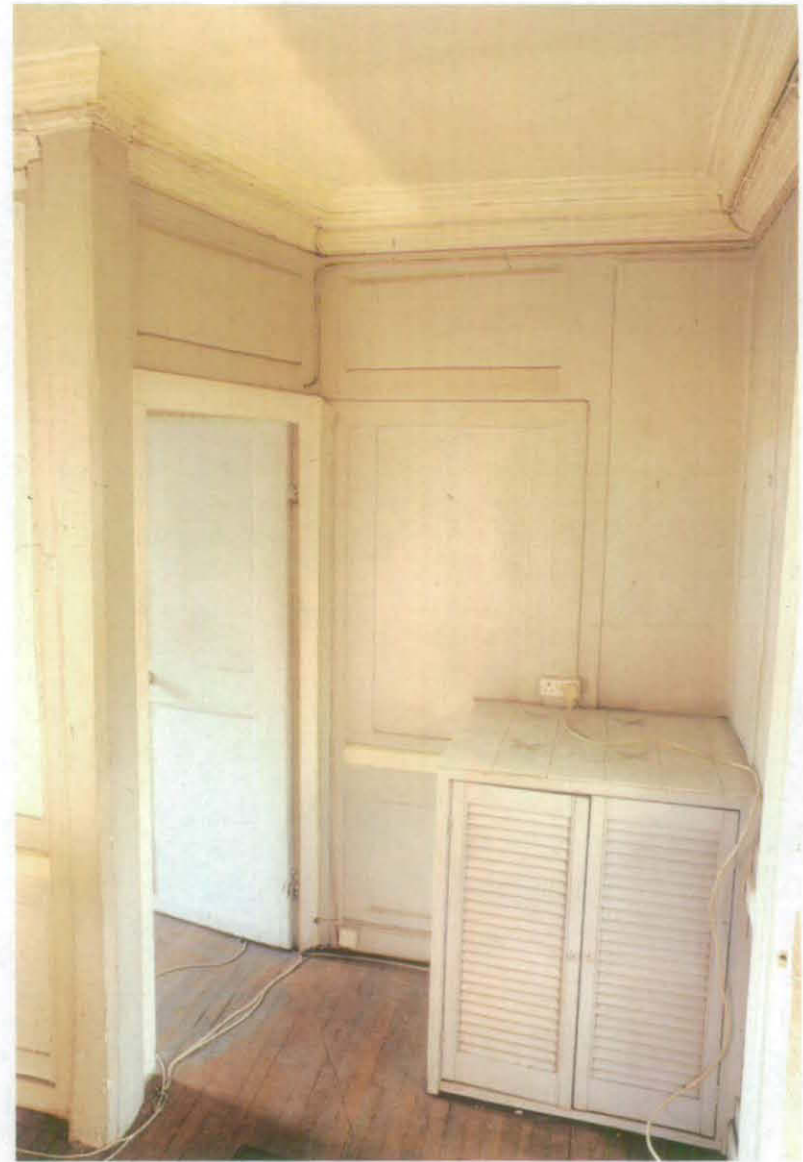
Fig 31 Consistent plain panelling and door frames [52] around the east and south sides of 2F1; looking east
