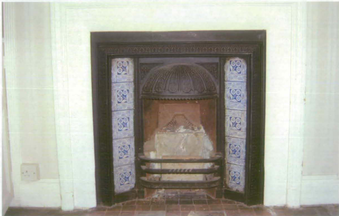
Fig 43 Ceramic fire surround and cast-iron grate in B5; looking west (A J Browne, Architects)
