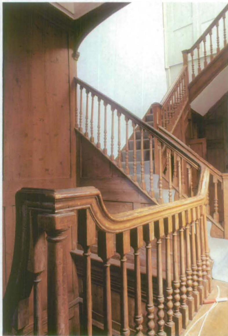
Fig 38: Head of principal staircase on 1F1, and enlarged service stair beyond, rising from 1F2 to 2F1, the latter rearranged as an open-well newel staircase similar to the former; looking north
