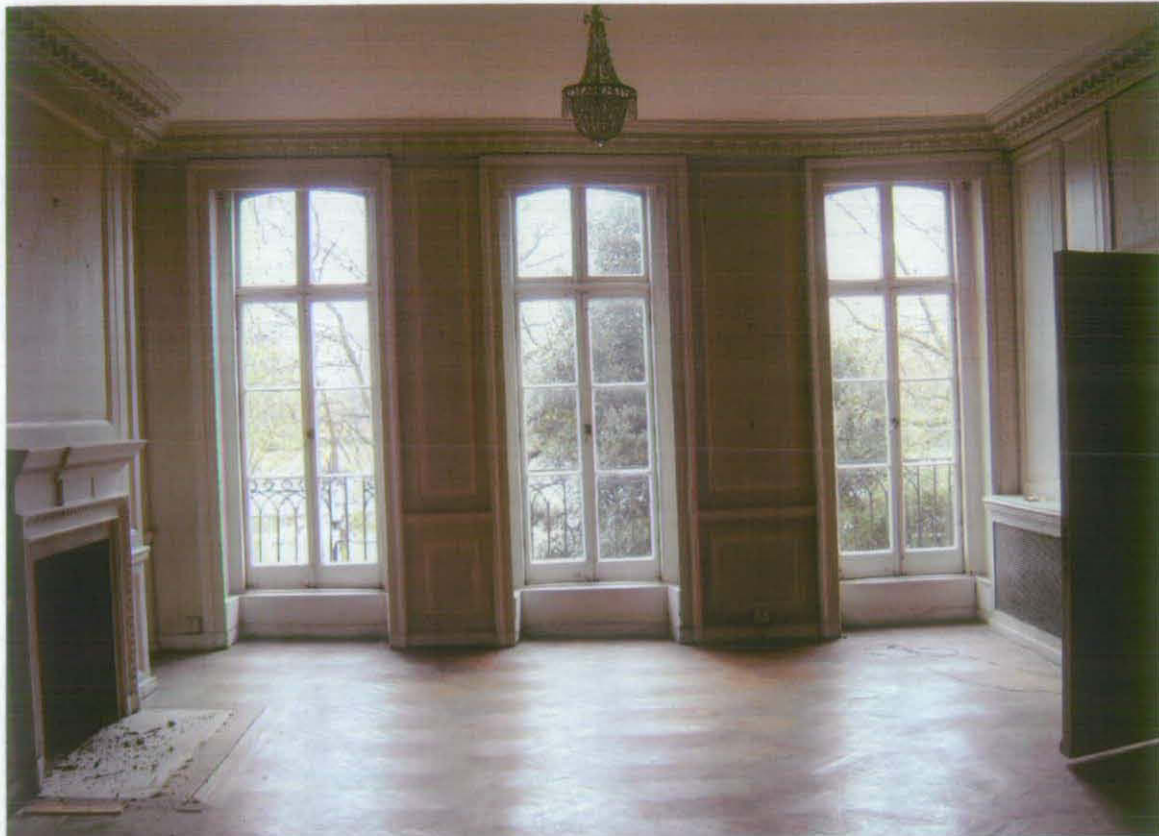
Fig 40 Southern half of 1F6, showing one of two chimney breasts and fireplaces in this room, and highly decorated cornice; looking south (A J Browne, Architects)
