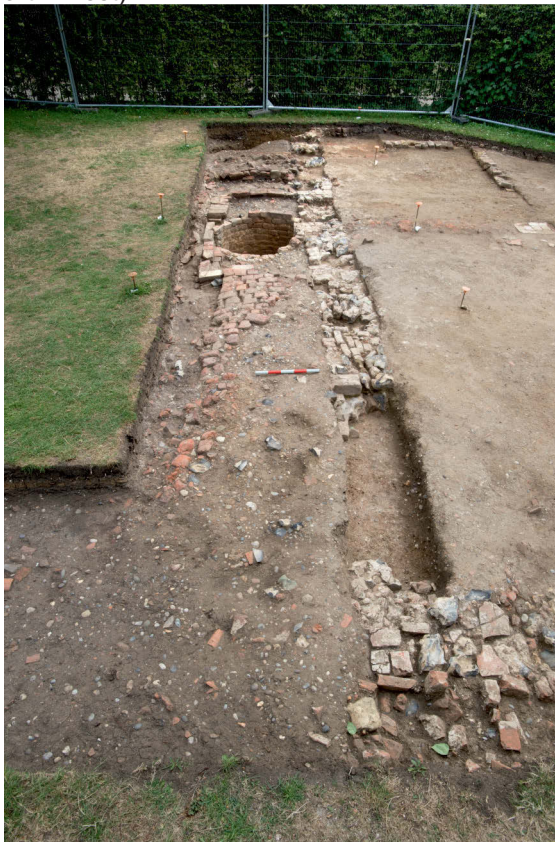
Fig 10 Area B: Remains of poorly constructed ancillary structures built against the external east wall [107] of Headstone cottages (looking south)
