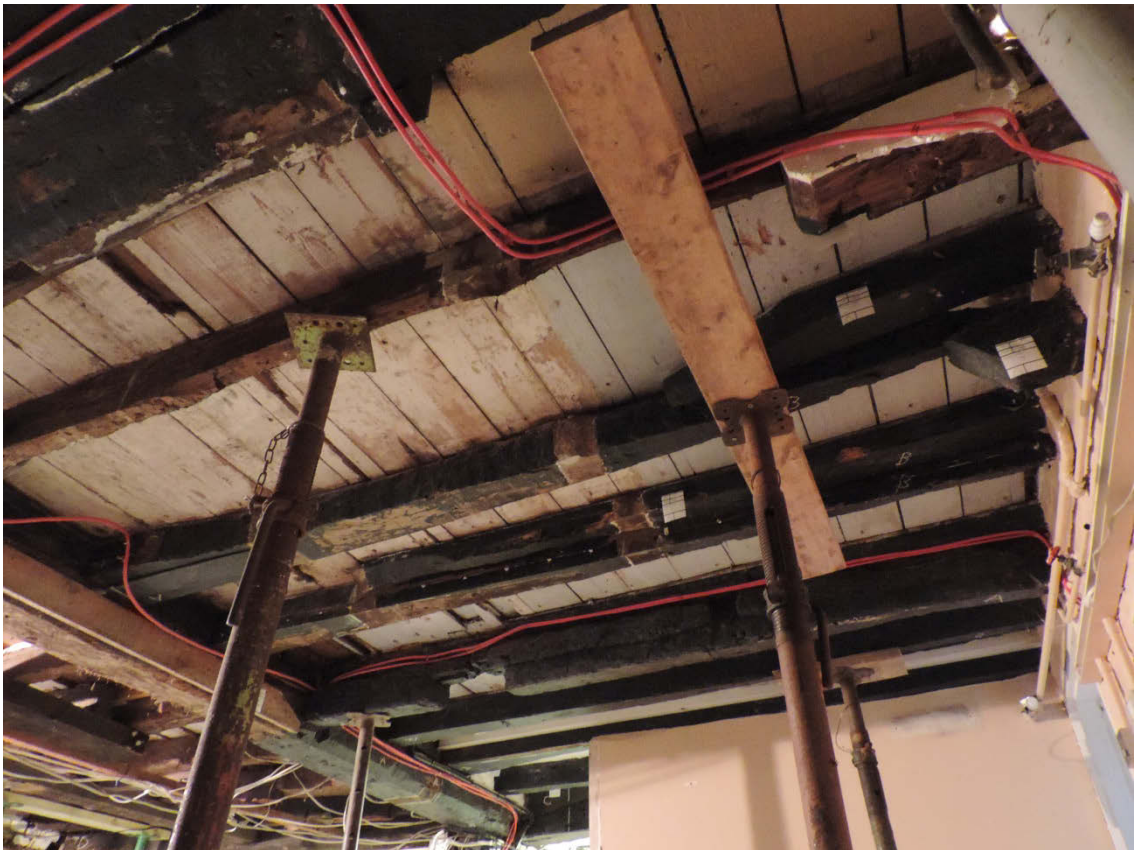
Fig 11 Timber doubling beam [47], looking north-east. Third joist from the top.
