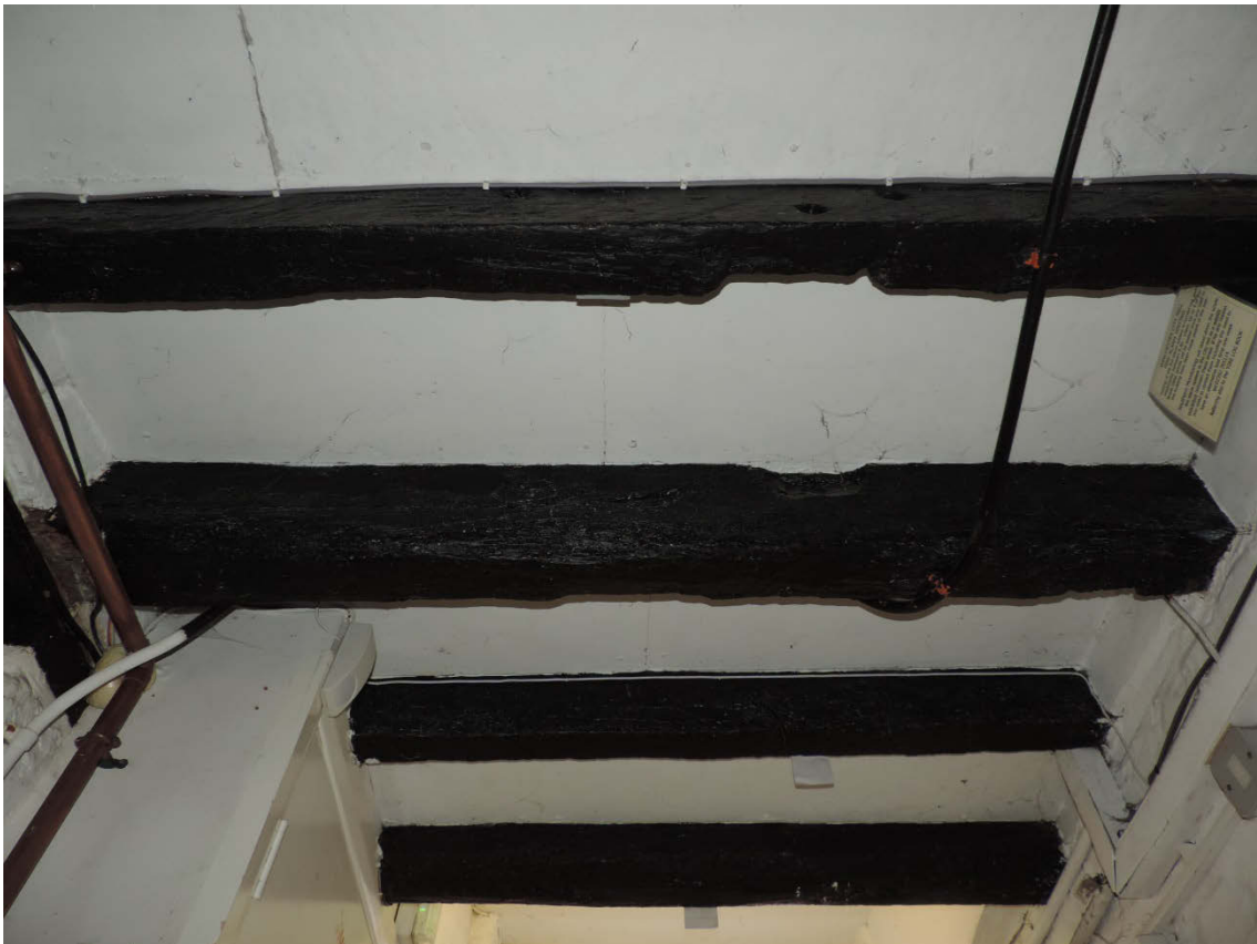
Fig 5 Timber [03], second from top, facing east
