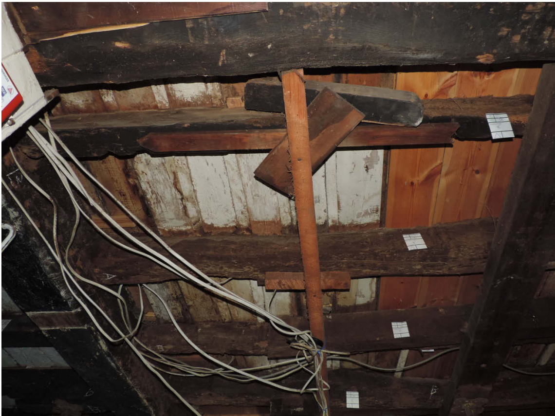
Fig 7 Timber [51], third labelled timber from the bottom, facing west
