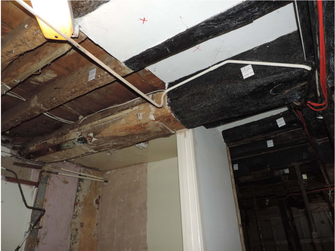
Fig 16 Timber [105], looking south-west, the timber with the most potential for a successful dendrochronology date. Sap wood can be observed near where the unpainted and painted portions of the timber meet.
