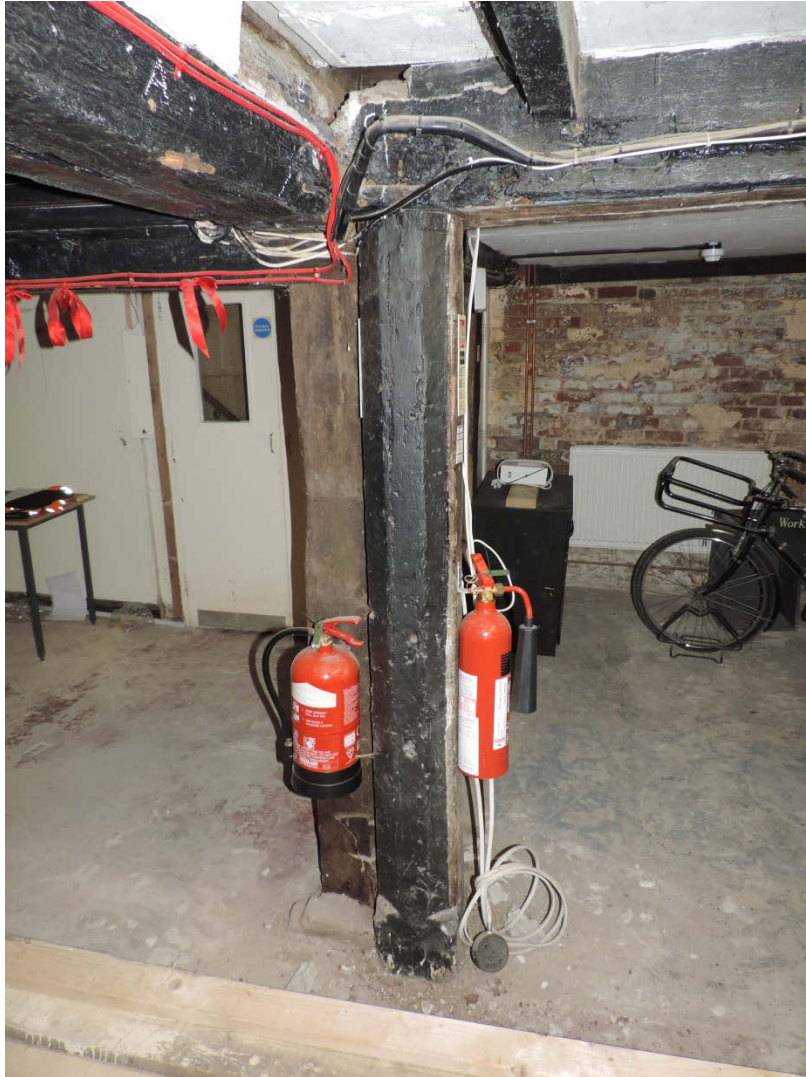
Fig 3 Timber post [200], likely a reused crown post.
