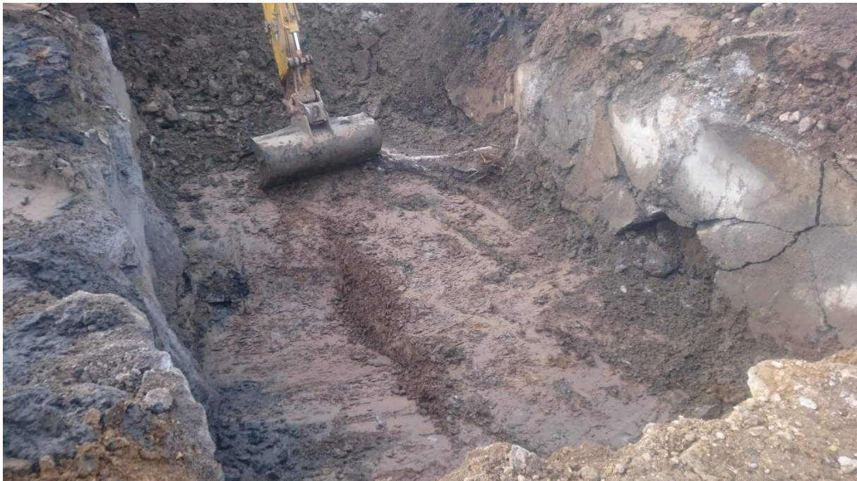
Photo 3 London clay observed at the base of the diesel tanks in the south-eastern part of the site.
