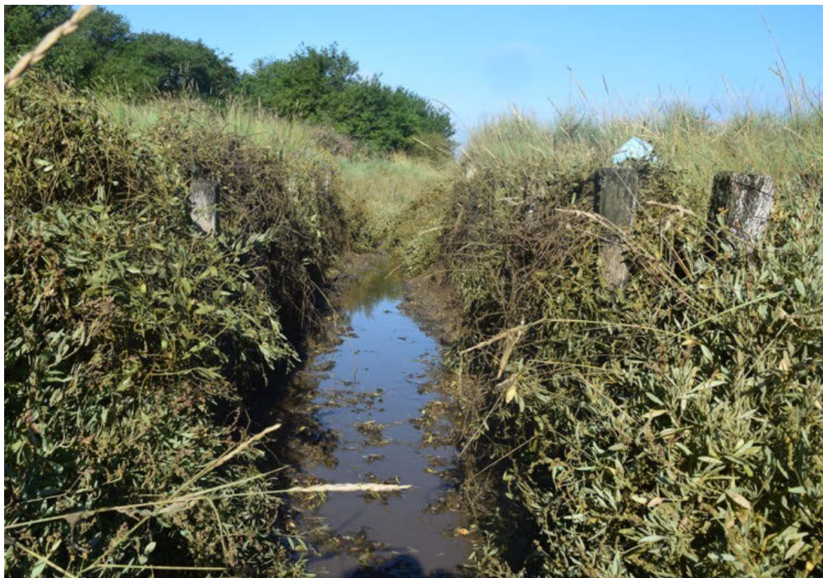
Drainage channel on southern side of oyster pits
