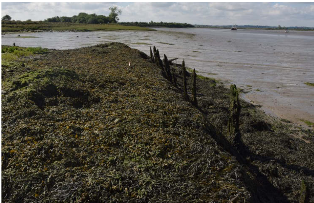
Wharf looking south-west showing timber revetments along western side
