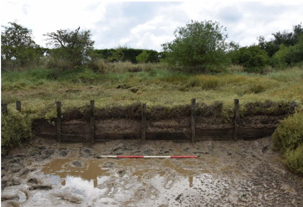
Southern end of north-eastern oyster pit showing timber revetments
