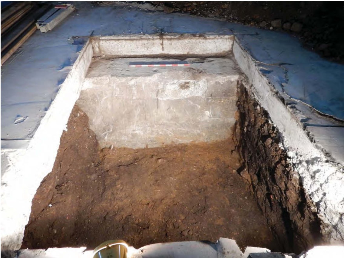
Fig 5 Reinforced concrete floor beam in Trench 4, looking SW (1m scale)
