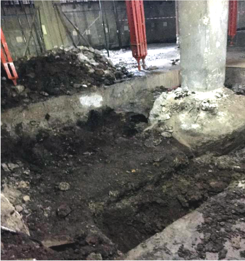
Fig 3 General view of lift pit excavation (WT Partnership)
