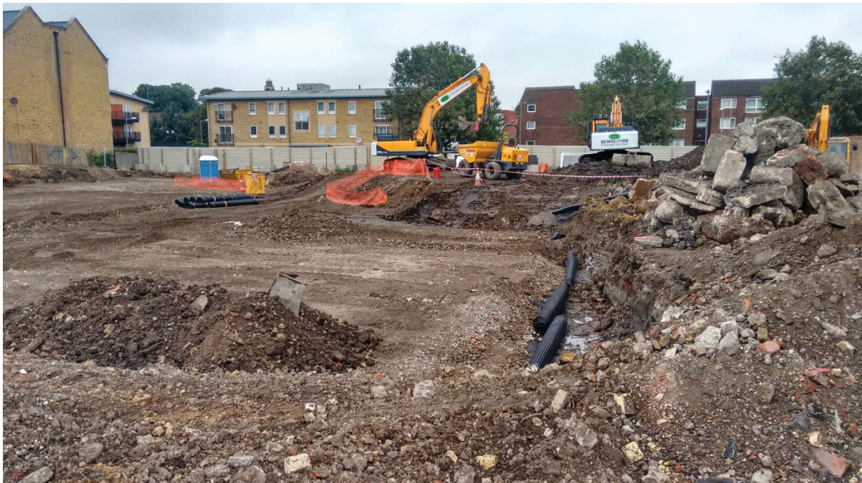
Photo 1. The bulk level reduction in progress, looking east
