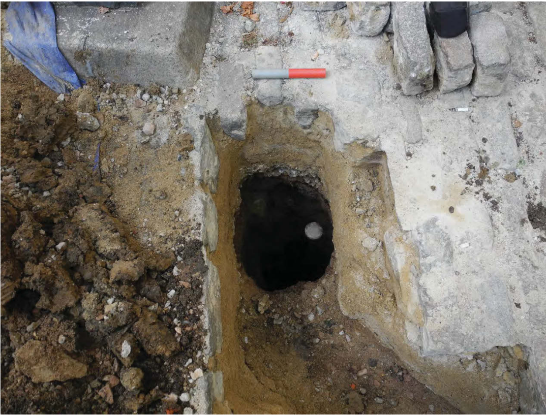
TP08 looking north, stone block is just visible in northwest corner of trial pit
