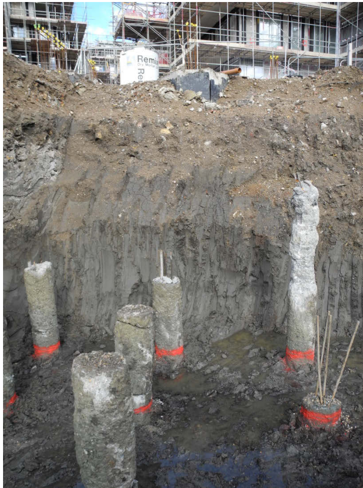
Photo 2: Plot B showing typical depth of alluvial clays found in this area.
