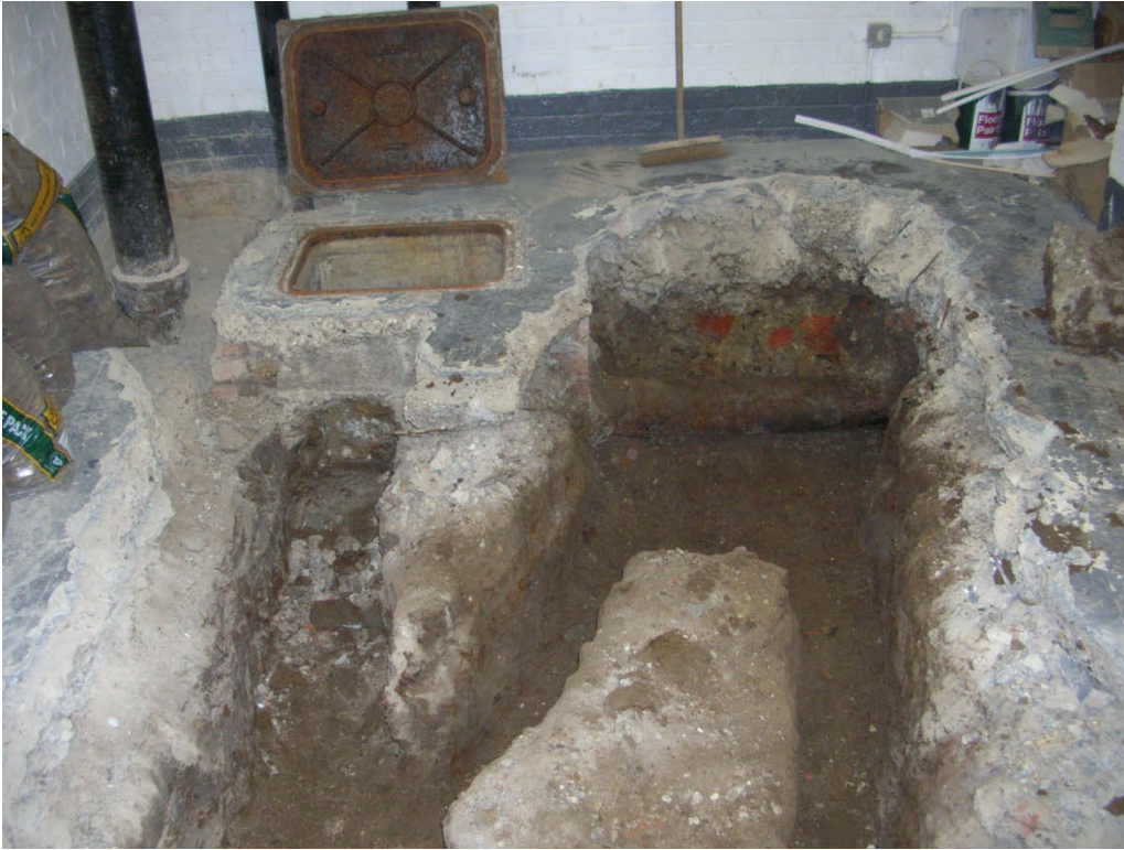
Photo; Trenches 3 and 4 and the new chamber looking north
