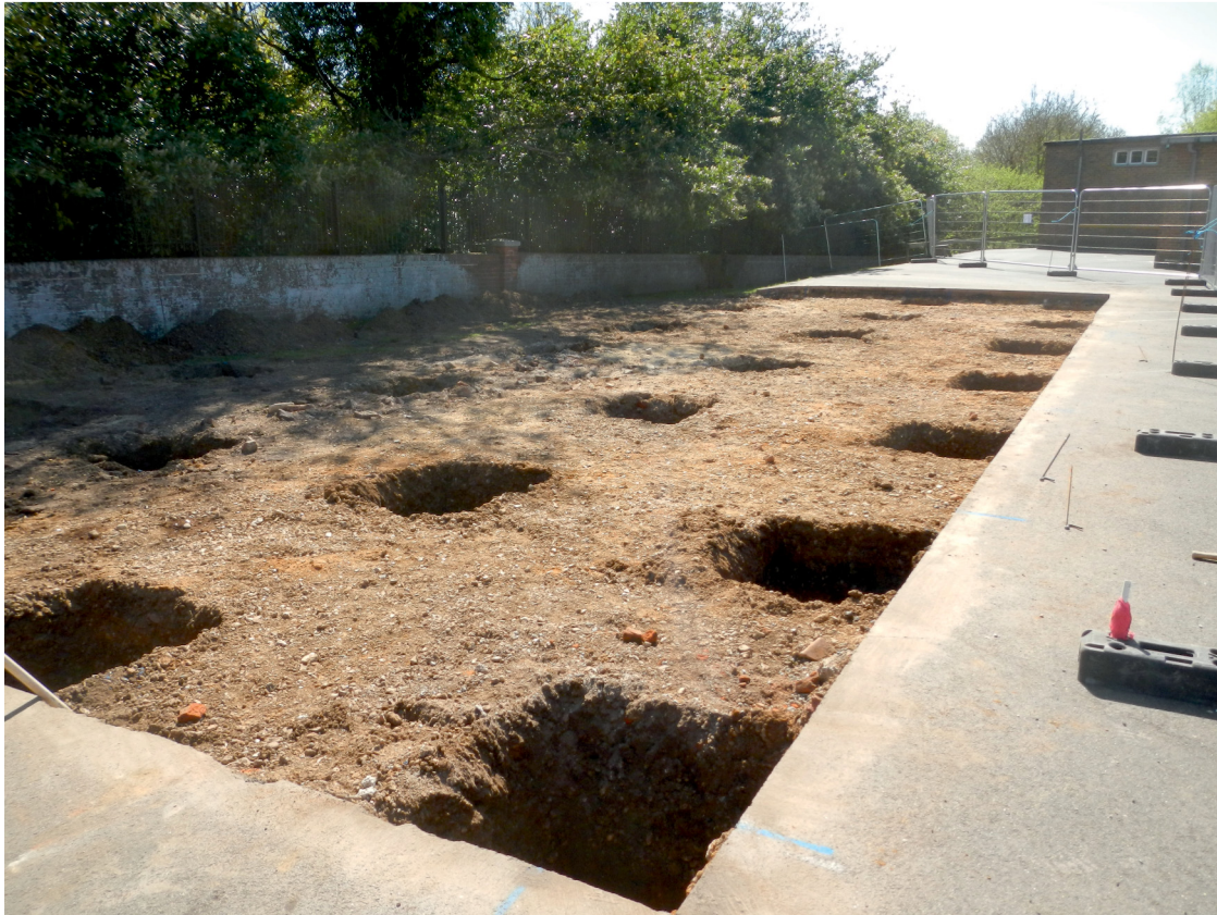
Fig 3 General view of the site post excavation; facing SE
