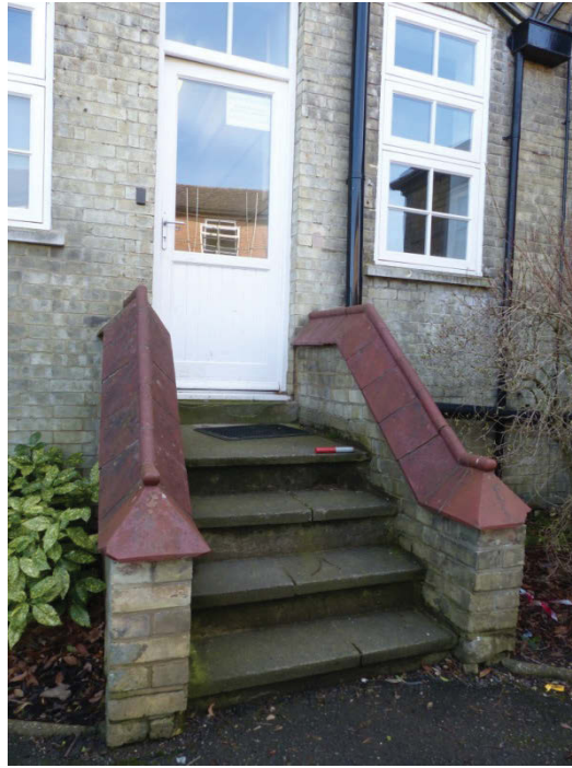
Fig 29 The steps on the eastern side of the north façade (Phase 2)
