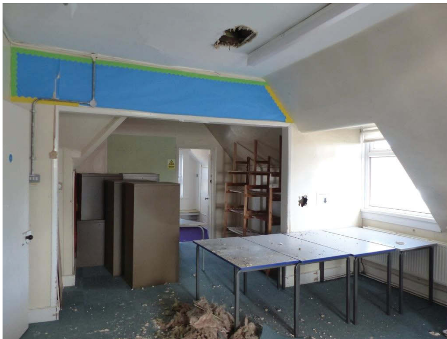
Fig 101 Room 2F3 looking south
