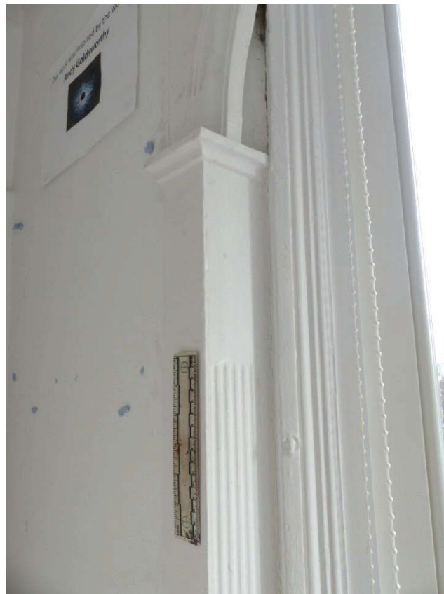
Fig 91 A detail of the fluted jambs and the impost of the Tudor arch, room 1F4, looking south-east
