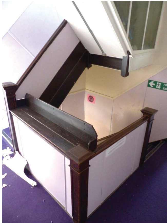
Fig 75 The staircase on the 1 st floor landing, looking north-west
