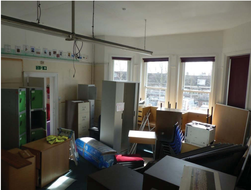
Fig 62 Room G2 looking south-east
