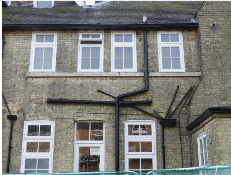
Fig 31 The north facing façade of the Phase 2 extension, looking south.
