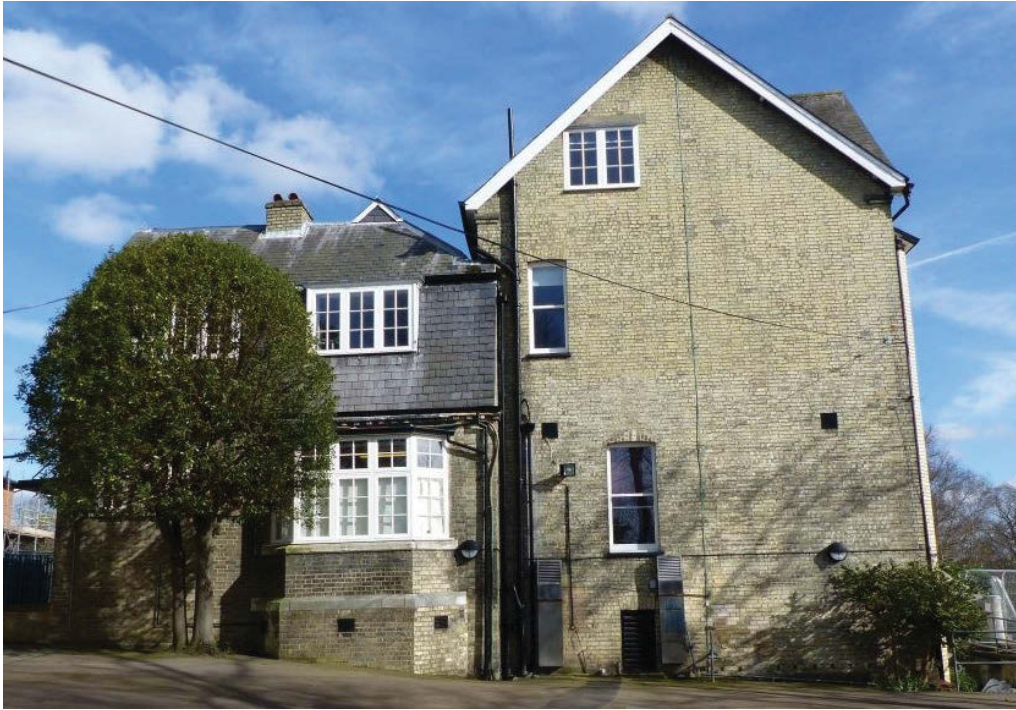
Fig 36 The west façade, looking east
