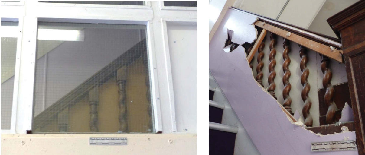
Fig 73 Twisted balusters, left on the ground floor behind a modern glazed partition, right on the 1 st floor leading up to the 2 nd floor level
