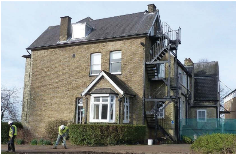
Fig 22 The east façade, looking west
