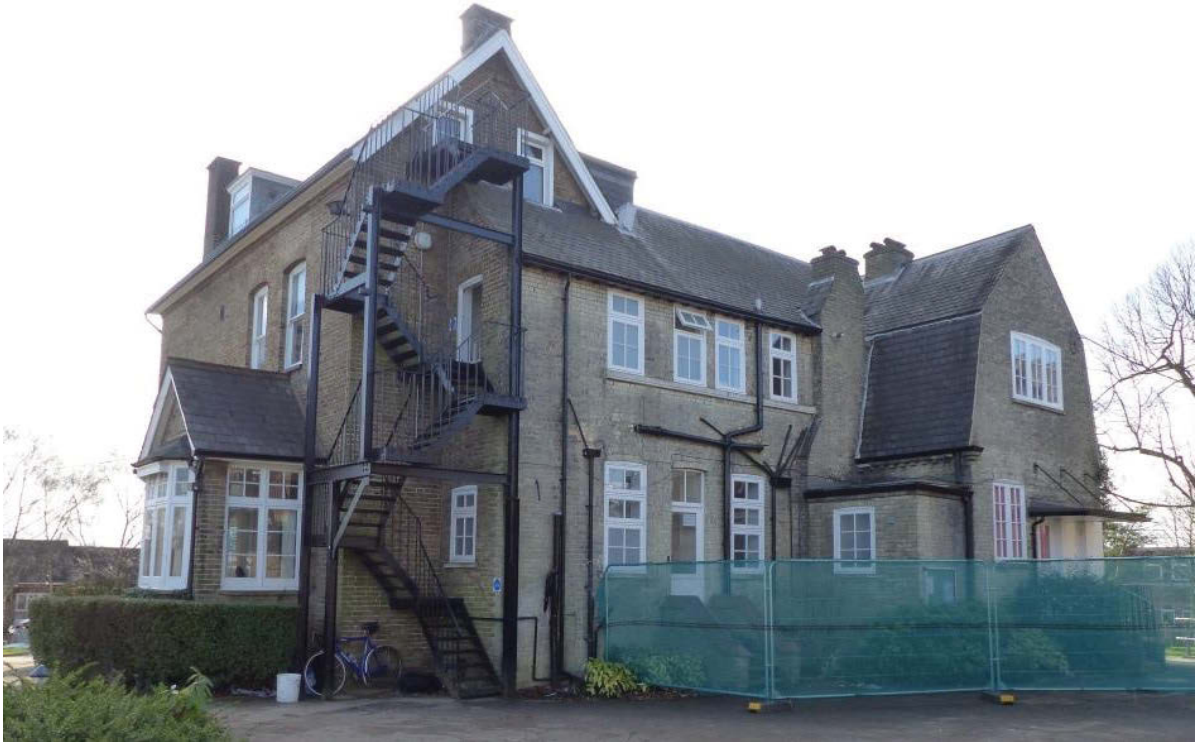
Fig 26 The east and north facades, looking south west.
