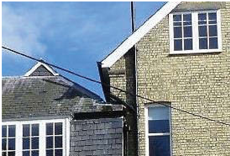
Fig 37 A detail from a photograph of the west façade, note the fragment of cornice below the bargeboard and roof eaves in the centre of the photograph. Note also the gablet of the Phase 2 roof on the left
