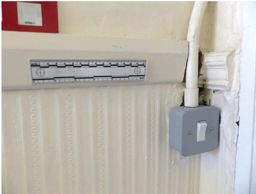
Fig 70 The textured wallpaper and two of the three types of dado rail in corridor G7
