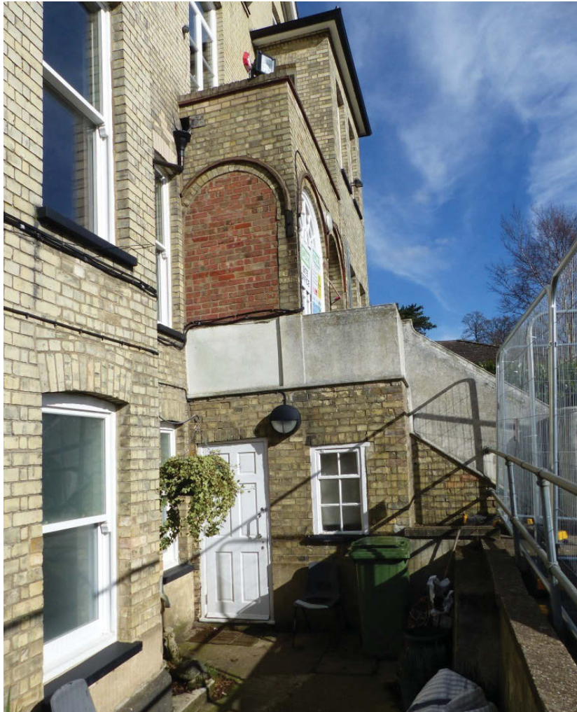
Fig 17 The porch viewed from basement level, looking east
