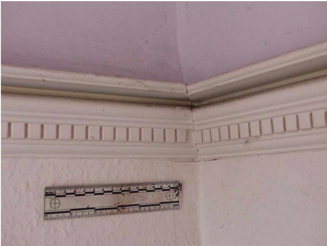
Fig 83 The picture rail in room 1F2, looking north-east
