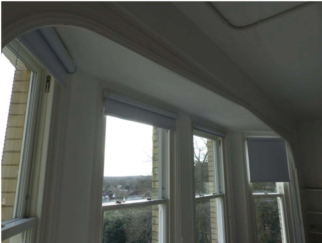
Fig 90 The timber, Tudor arch in front of the bay window, looking south-west
