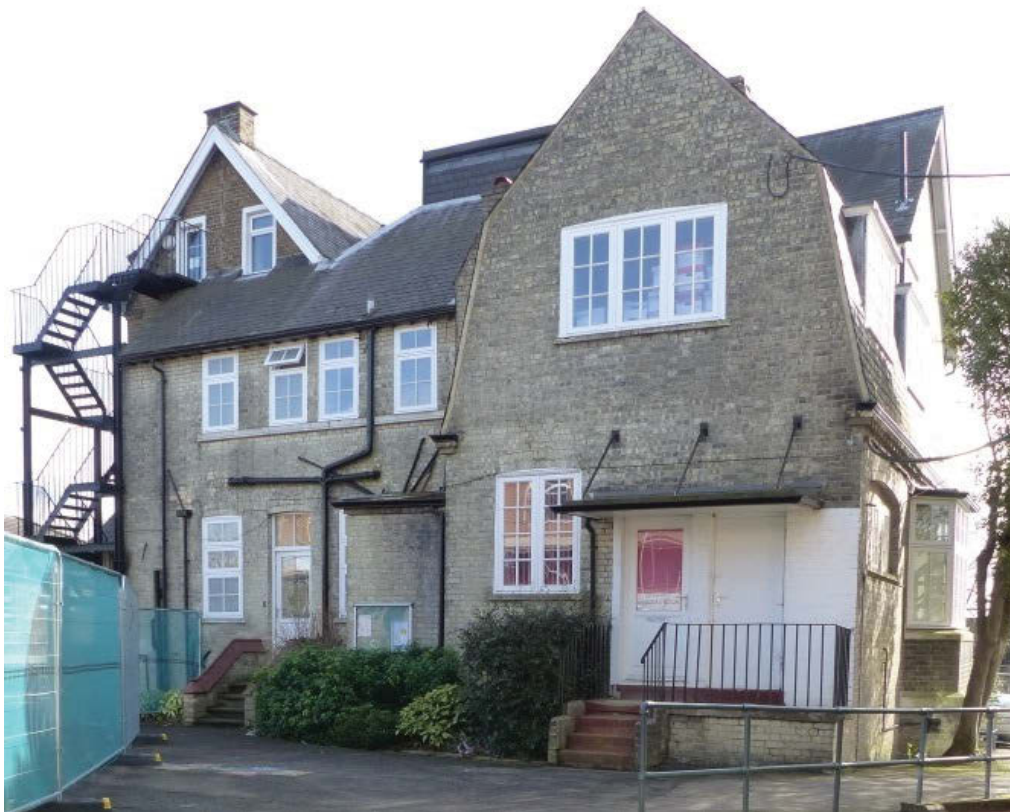
Fig 28 The north façade, looking south-east
