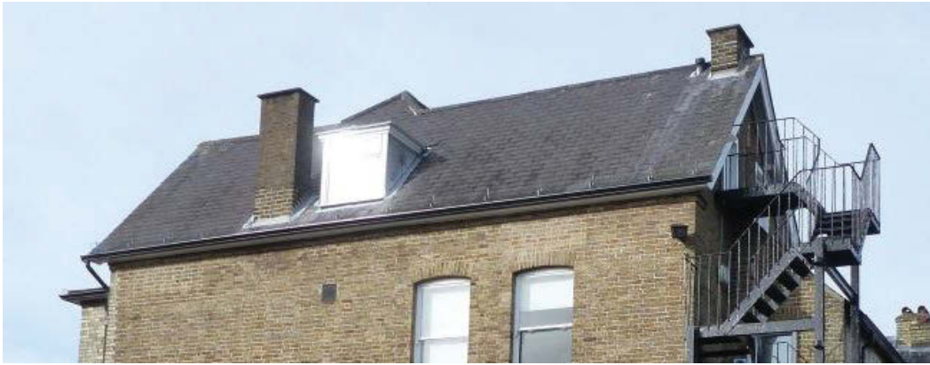
Fig 42 The Phase 1 north-south roof, looking west
