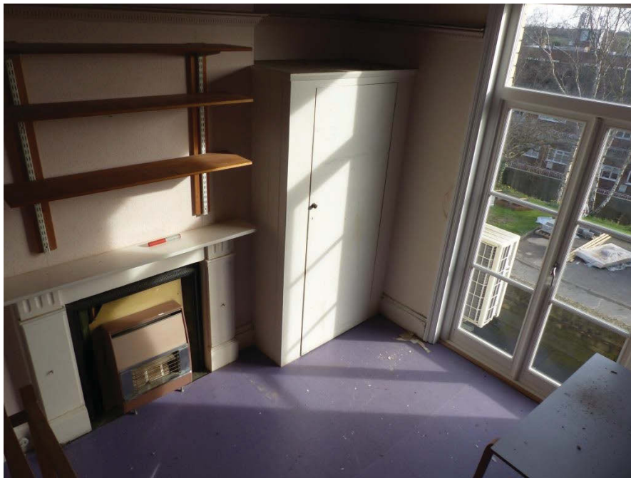
Fig 81 Room 1F2 looking south-east
