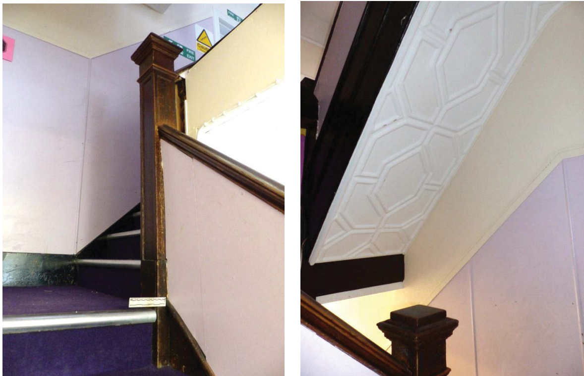
Fig 74 The flight from ground to 1 st floor. Left, a less decorated newel post looking north-west. Right, decorative plaster work on the ceiling above the stairs
