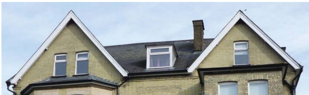
Fig 41 The two south-facing gables looking north. The larger example on the left is the gabled dormer. That on the right is the smaller gable end of the north-south roof.
