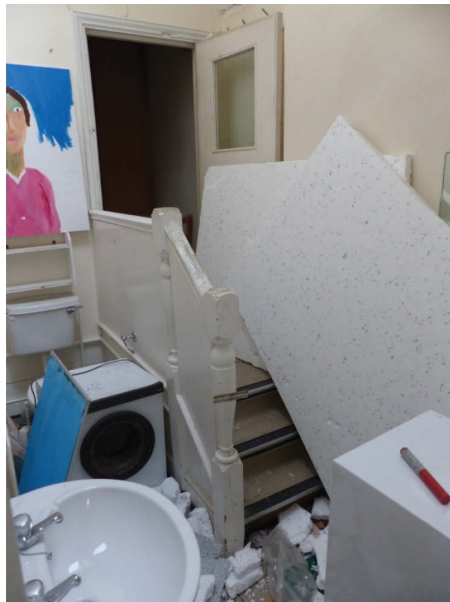
Fig 92 Room 1F9, looking east
