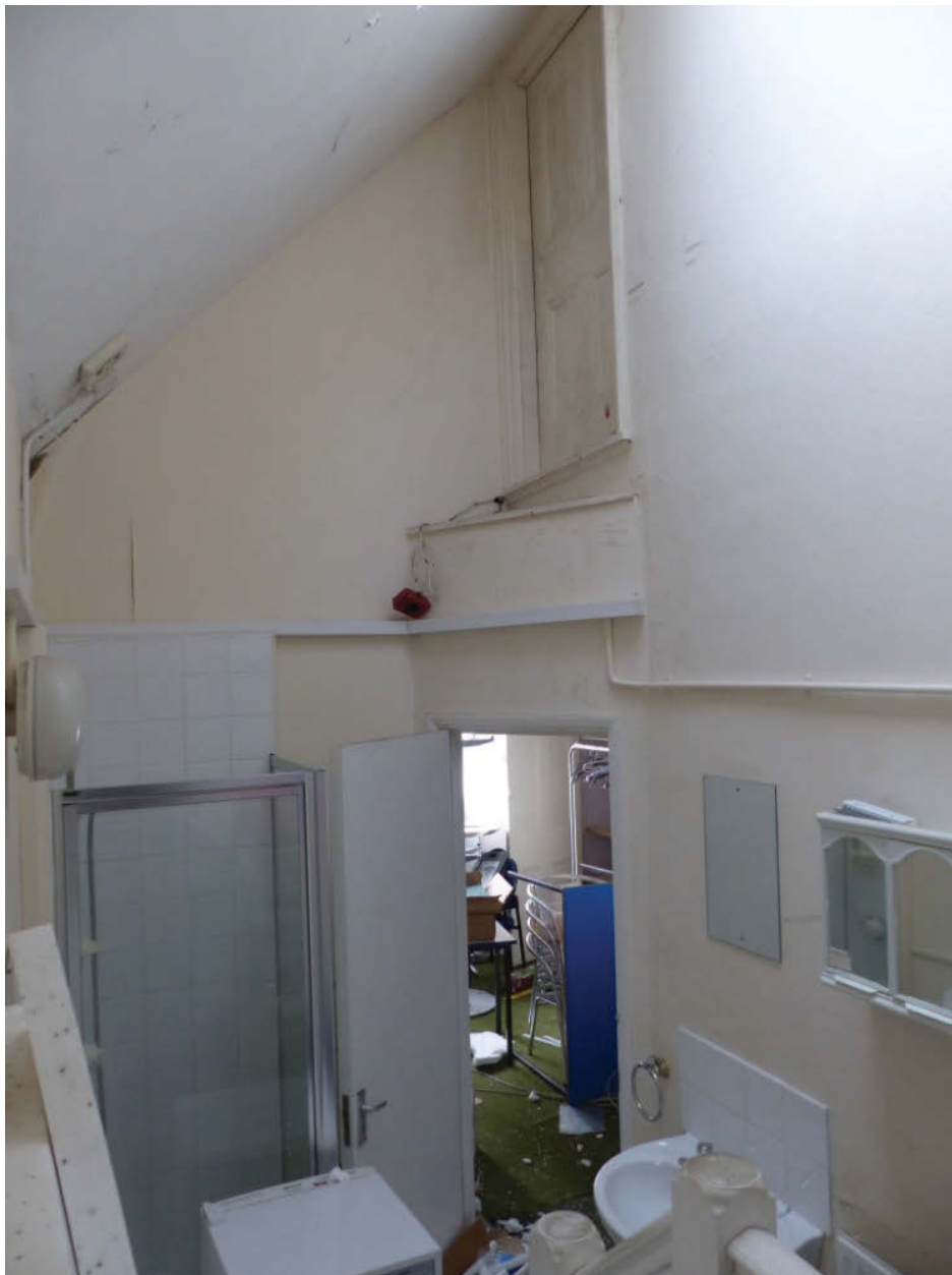
Fig 93 Room 1F9, looking west
