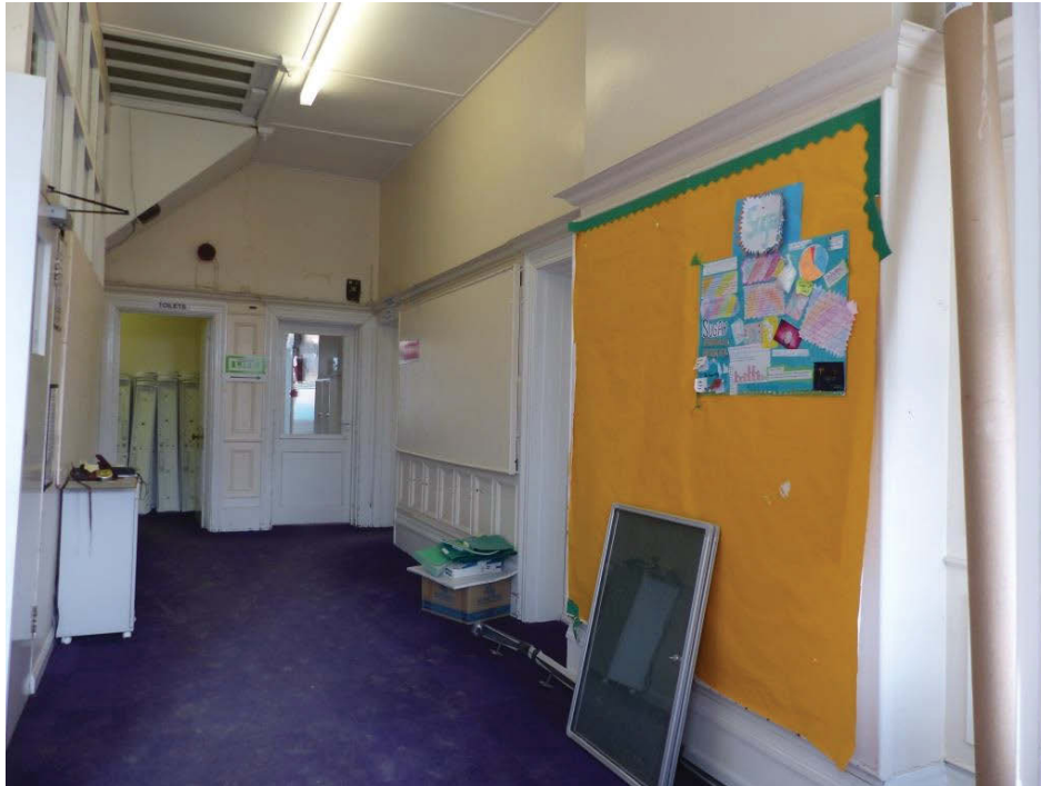
Fig 55 Room G1, looking north. The chimney breast is on the right with the adjacent disused doorway
