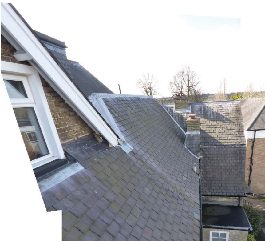
Fig 43 A composite photographs of two images, showing three phases of roof. The Phase 1 gable and part of the ridge can be seen on the left. In the centre is the double pitch Phase 2 roof. On the right is the Phase 3 gambrel roof.
