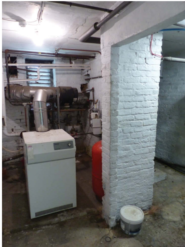
Fig 50 Room B5, looking north-west
