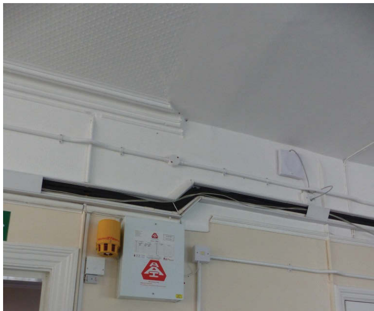
Fig 86 the end of the decorative scheme indicating the site of a removed partition wall, room 1F3, looking north-west
