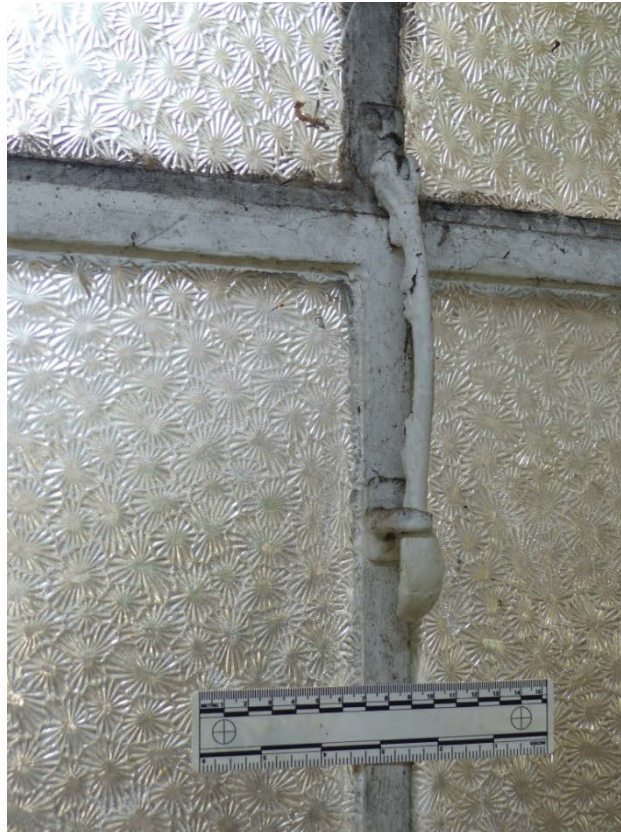
Fig 46 Ironmongery of the east window in room B1 looking south-east
