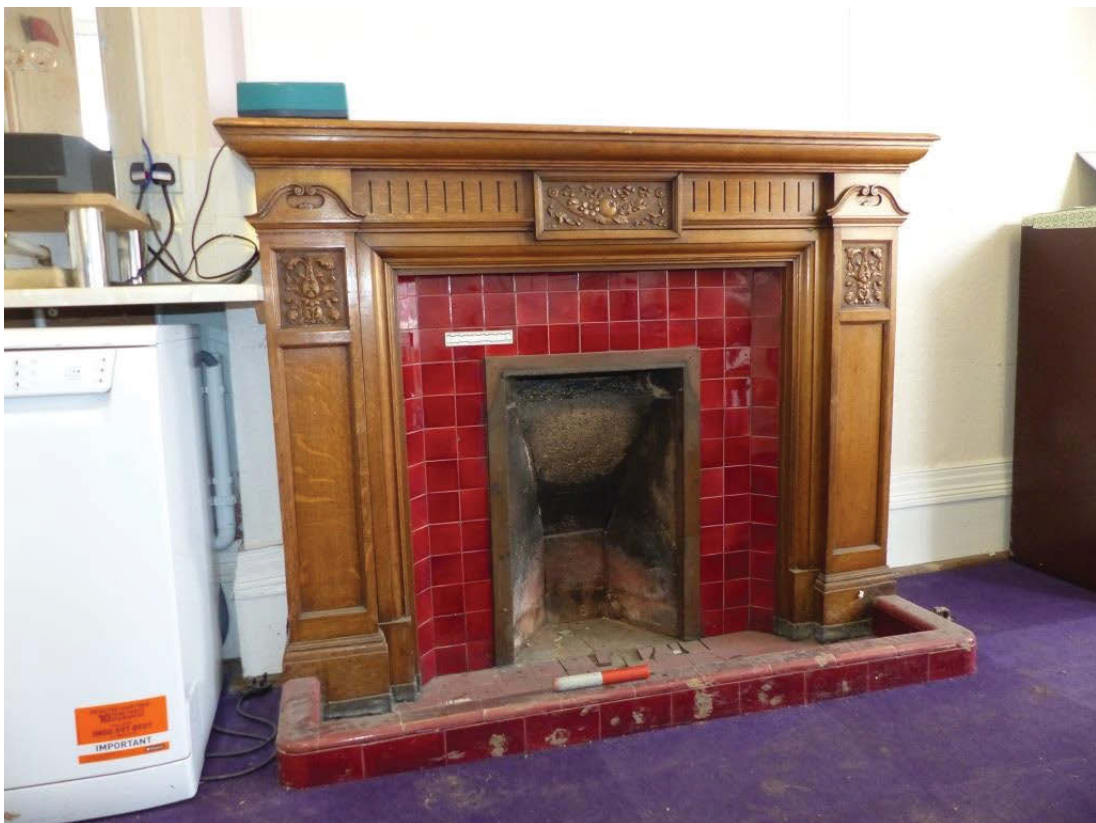
Fig 60 Fireplace in room G4, looking north
