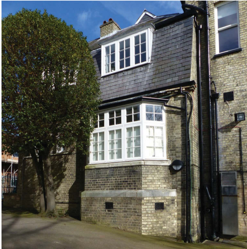
Fig 38 The bay window of the Phase 3 extension, looking north-east
