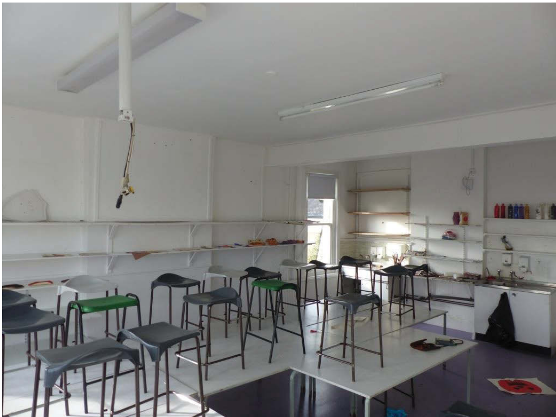
Fig 89 Room 1F4, looking north-west. Note the two chimney breasts, while the boxed-in modern RSJ can be seen in the ceiling running from the centre to the right of the photograph
