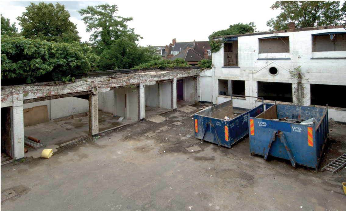
Fig 6 View to southeast of garage block at southeastern corner of site
