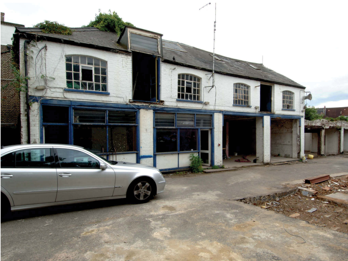
Fig 5 View to east of two-storey building on east side of site
