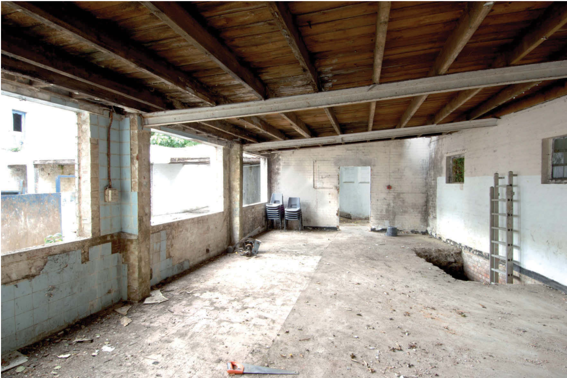
Fig 12 Internal view to south of building on west side of site
