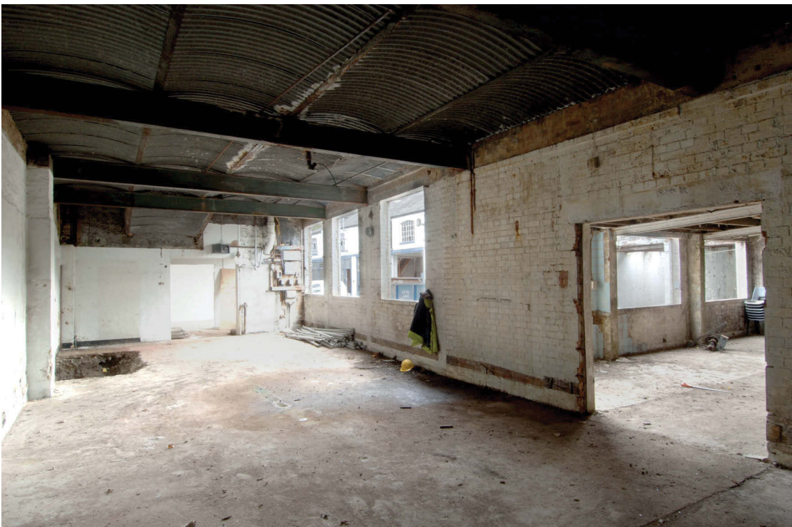
Fig 11 Internal view to north of building at western side of site with arched corrugated iron sheet ceiling
