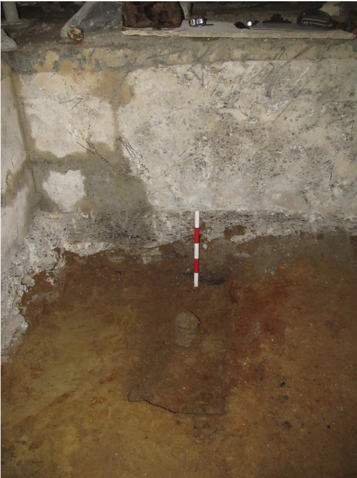
Fig 7 Looking east, showing excavated cut [3] with remnant of concrete core
