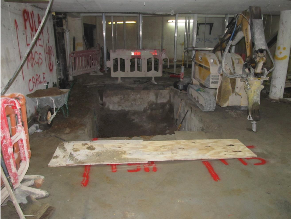
Fig 5 Looking north, showing location of excavation trench within basement
