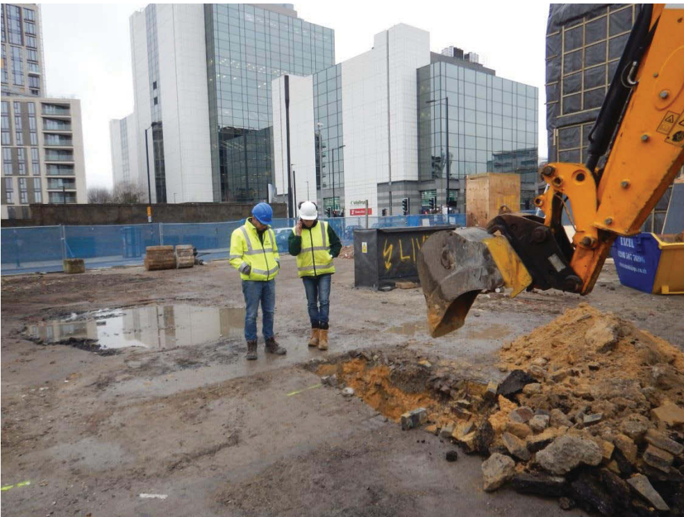
Excavation of trench containing gas main, looking southwest
