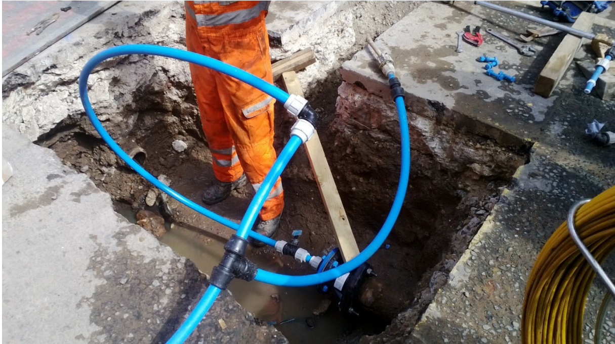
Fig 3 Launch/receptor pit
