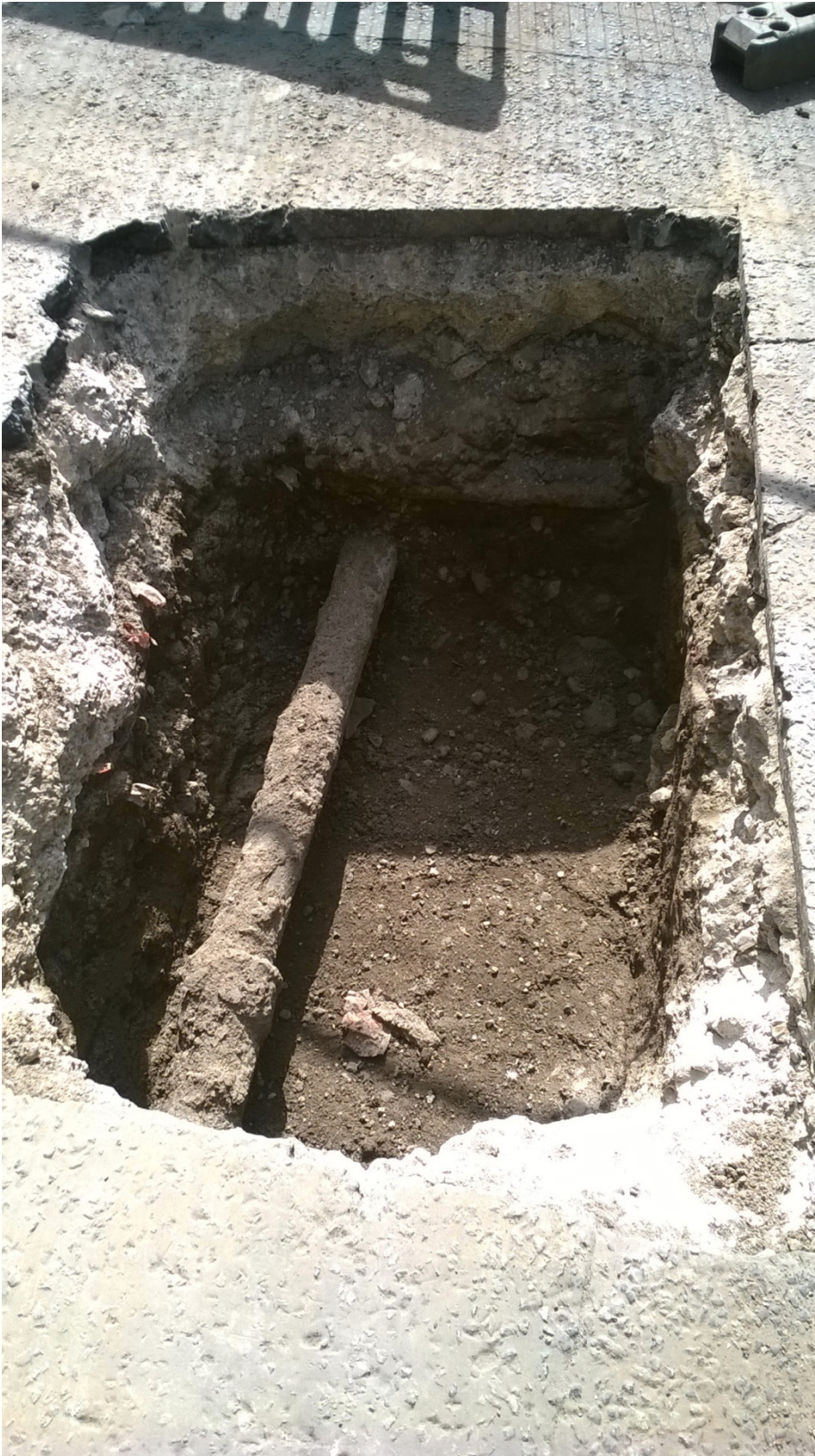
Fig 4 Pit at junction with Wigmore Street
