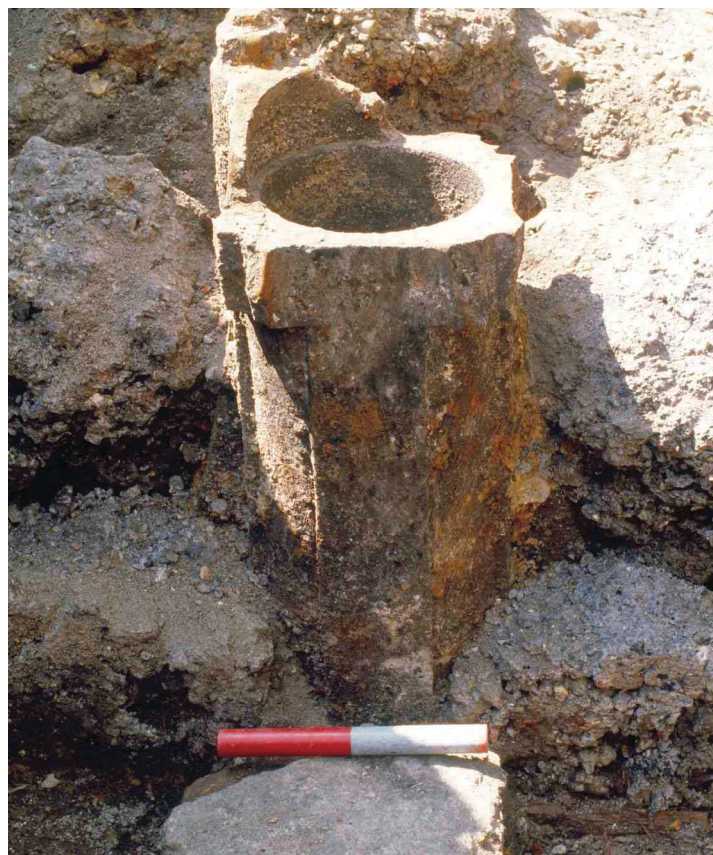
Fig 21 Iron column [44], set in concrete
