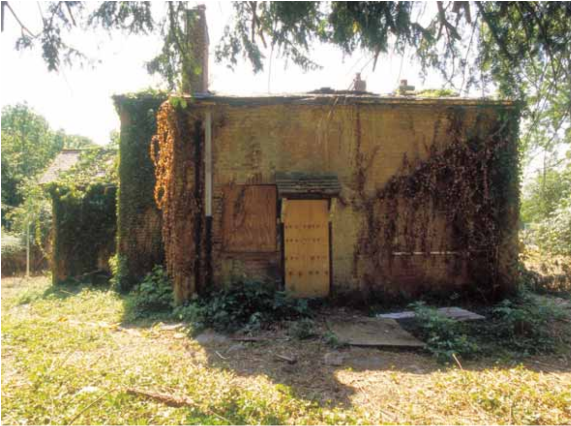
Fig 18 Looking south at the north front of the farmhouse
