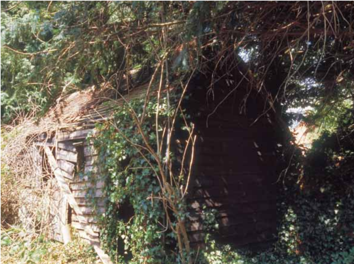
Fig 22 Exterior of the stable shed, looking west
