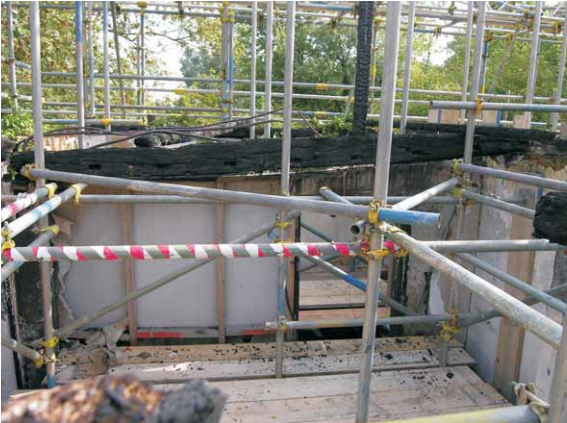
Fig 30 Tie-beam and post over IF1, looking east
