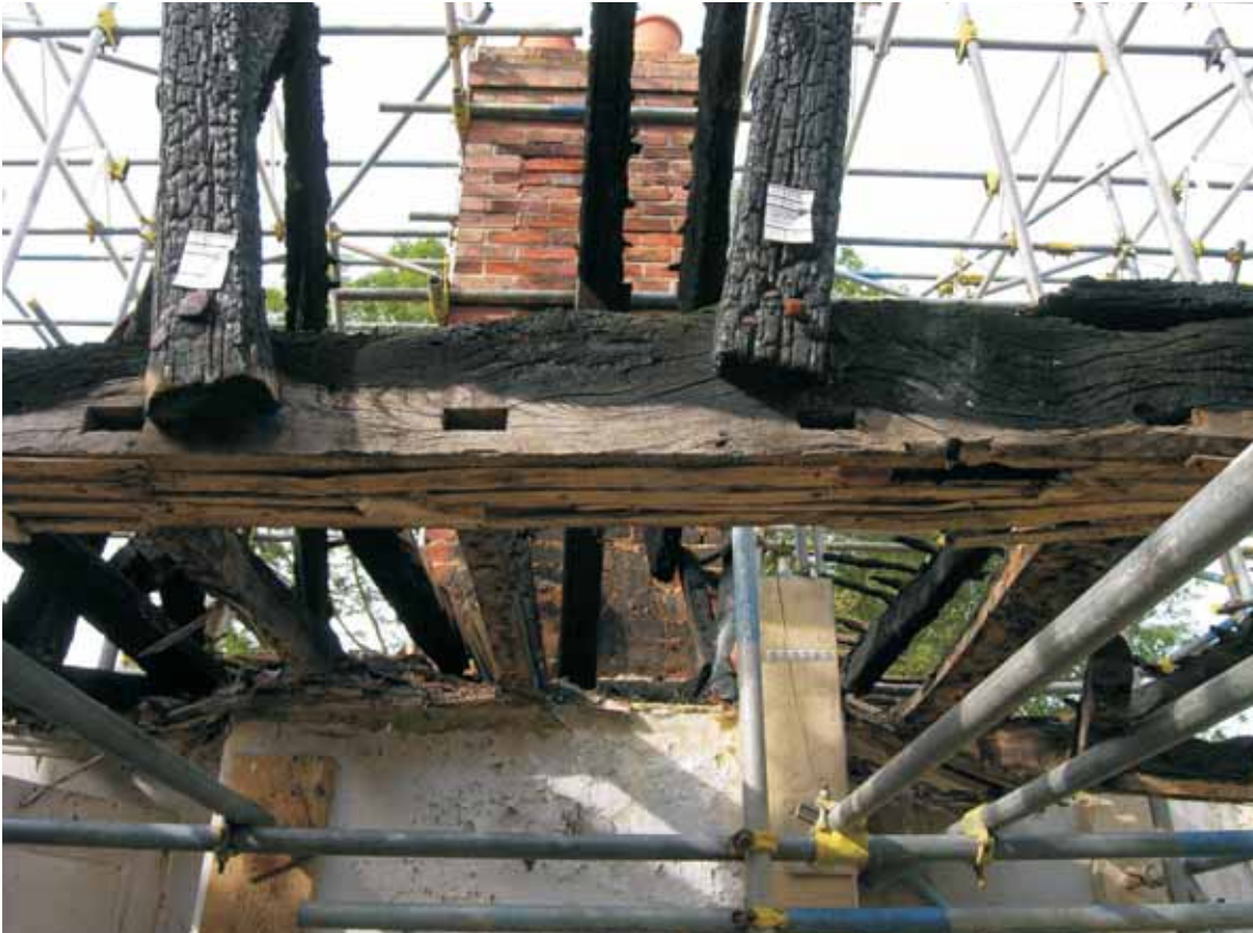
Fig 28 Tie-beam of surviving roof truss over IF4, looking west
