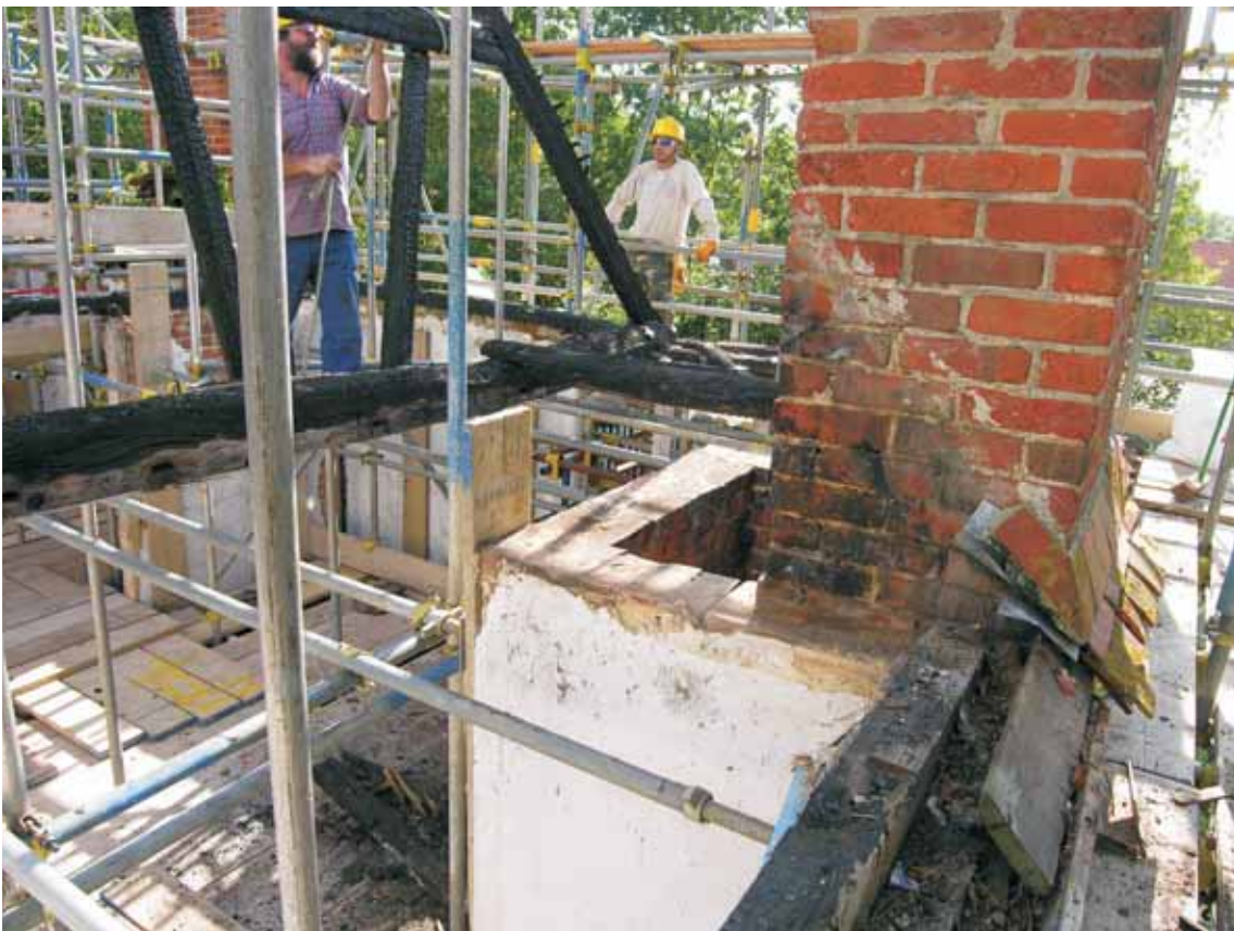
Fig 29 Chimney breast projecting into IF4, looking south-east
