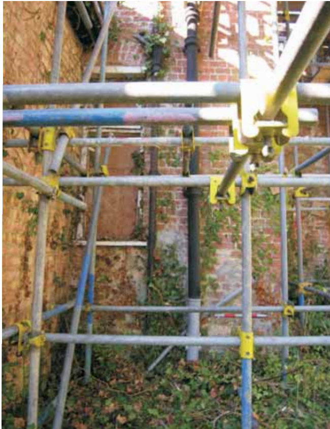
Fig 40 External face of east wall of G8, looking west
