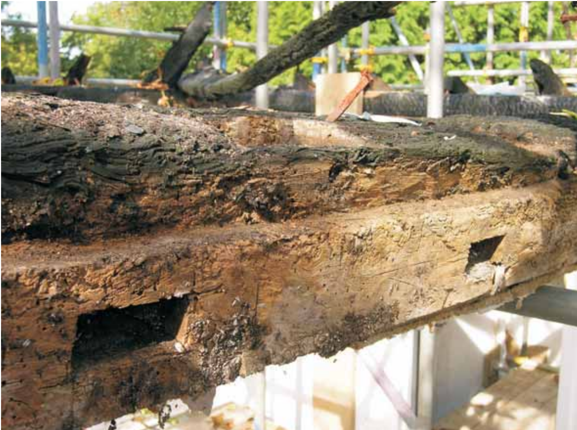
Fig 32 Detail of east face of tie-beam over IF5, looking north-west
