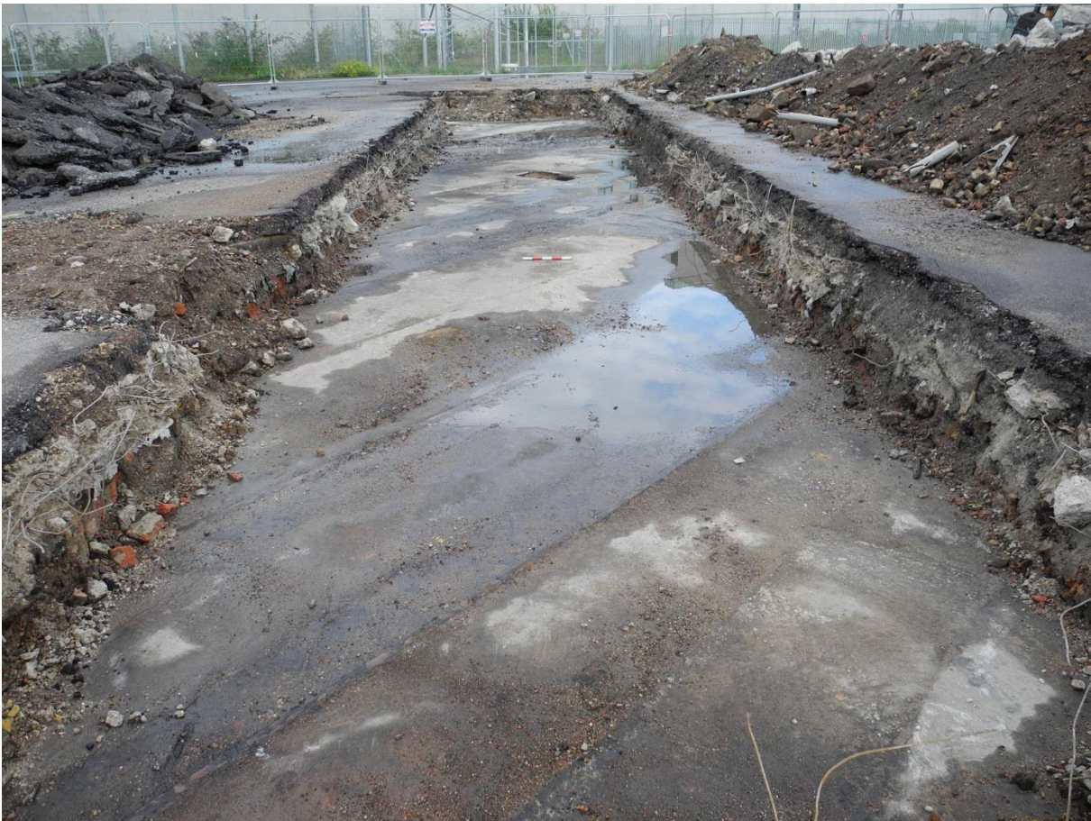
Photo: the railway tracks, Trench 5 looking North West
