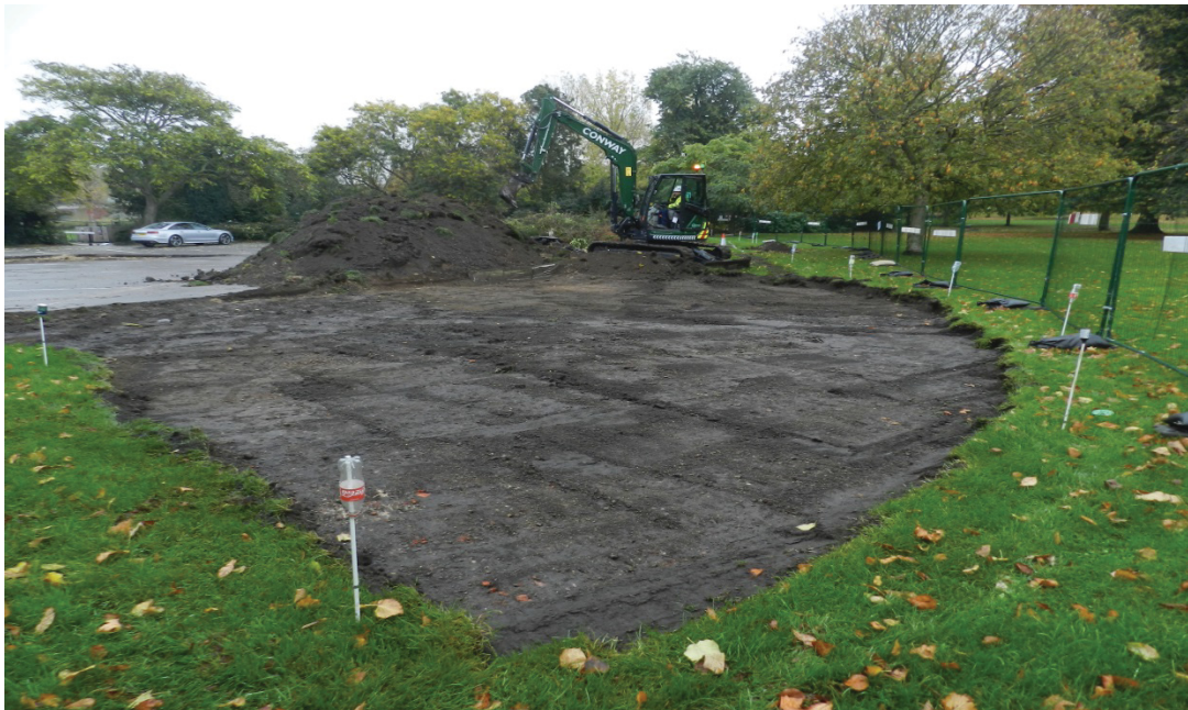
Photo 2 Ground reduction in advance of extending car park, looking North-east
