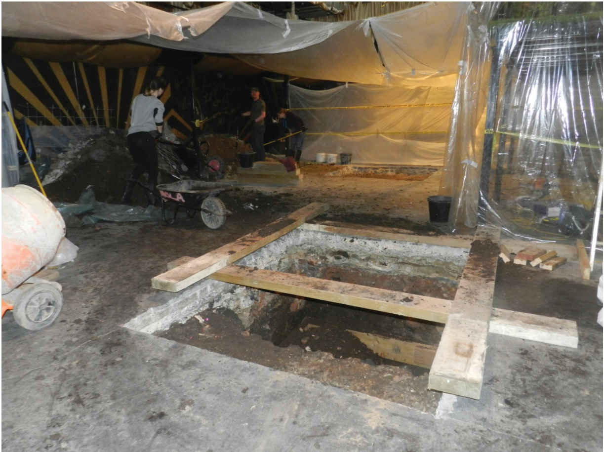
Photo 1 General view of Trench 1 (foreground) and Trench 2 (background), facing north-west
