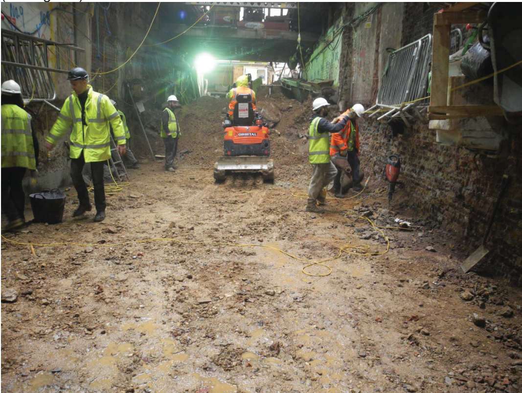
Photo: the site following reduction for the new basement (looking NE)
