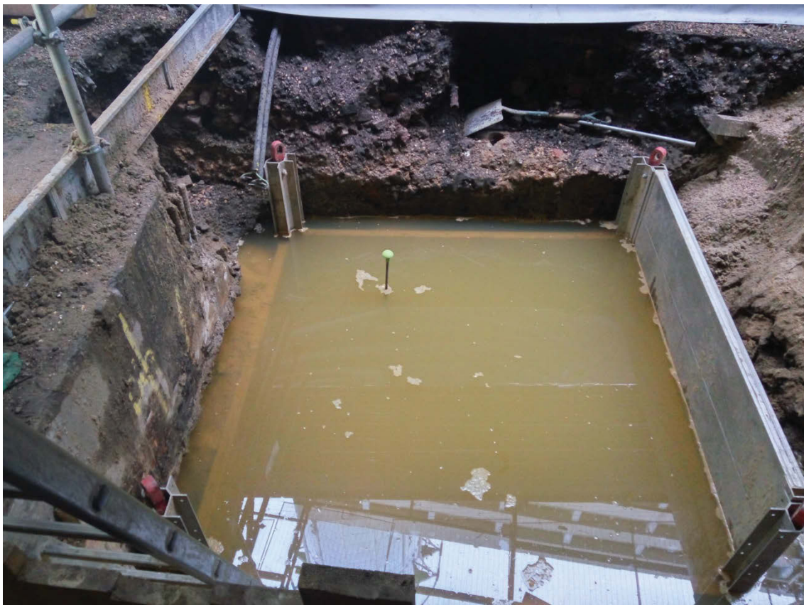
Photo 6 View of Pile probing trench 10 (looking north)
