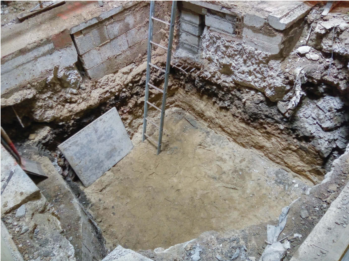
Photo 8 View of Pile probing trench 13 (looking southwest)
