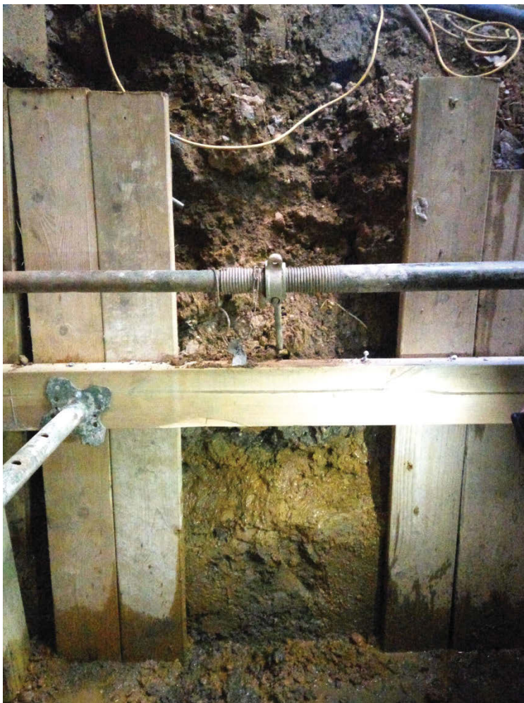
Photo 2 View of Pile probing trench 4 (looking east)
