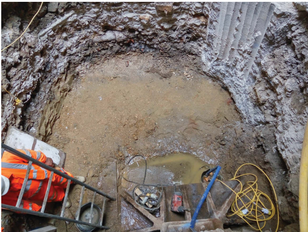
Photo 1 View of Pile probing trench 2 (looking north)
