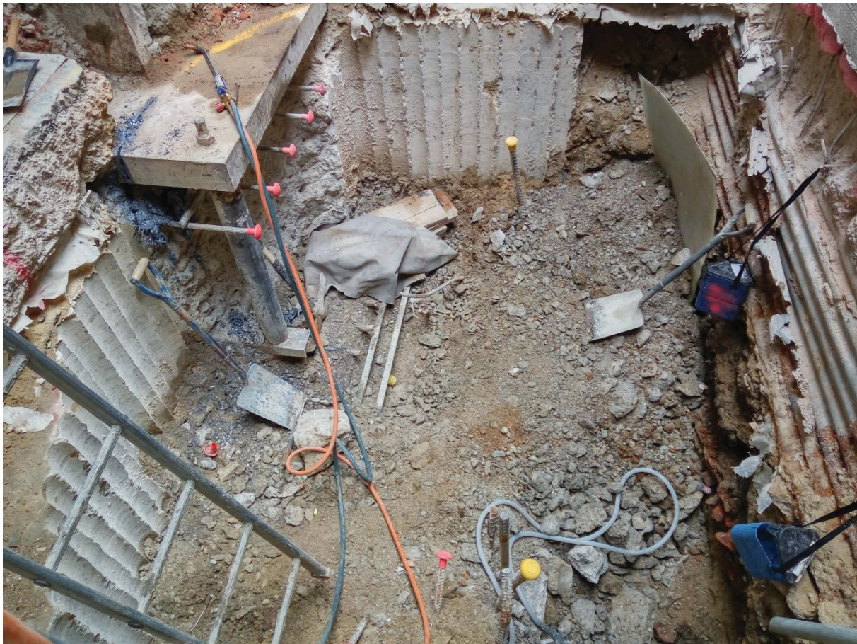
Photo 9 View of Pile probing trench 14 (looking north)
