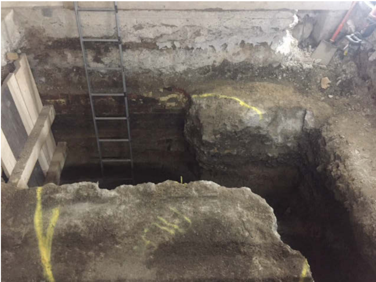
Photo 5 View of Pile probing trench 9 (looking north)
