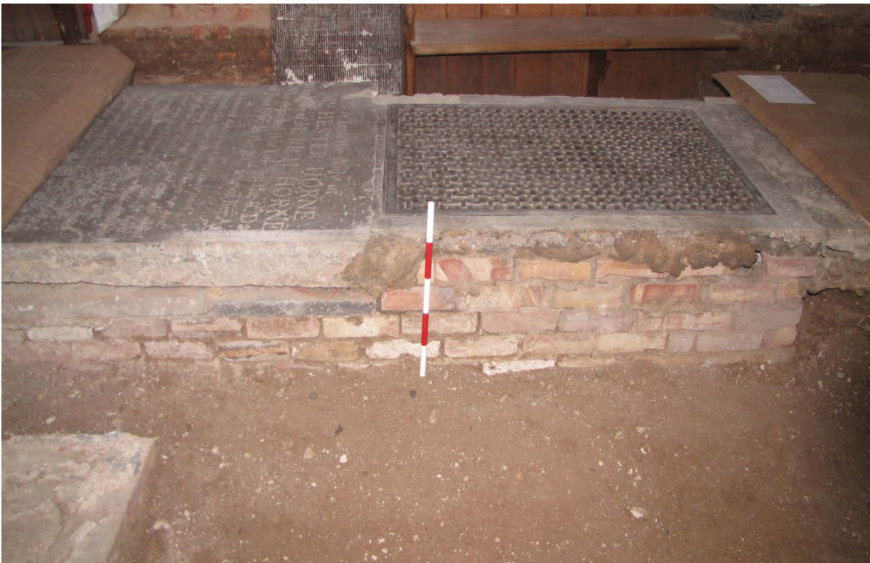
Photo 7 North aisle, Edwardian heating duct [30] with metal grille, looking south
