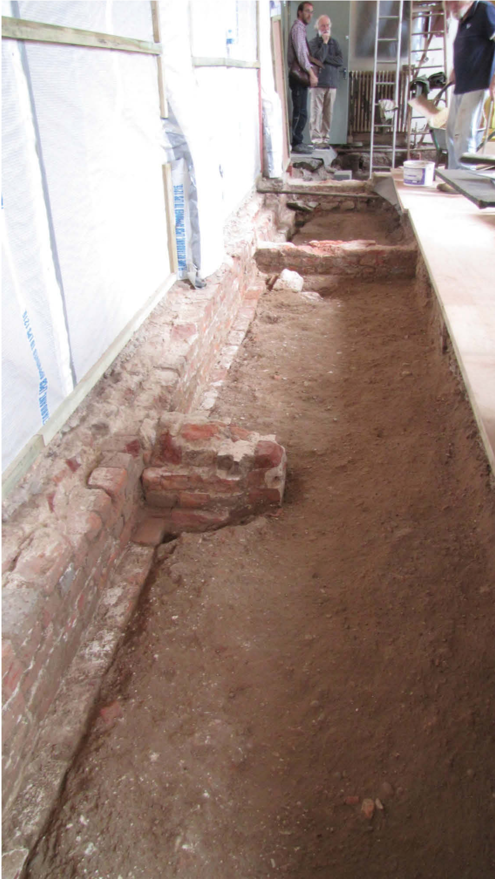
Photo 1 Wall [14] with walls [16] and [18] looking west
