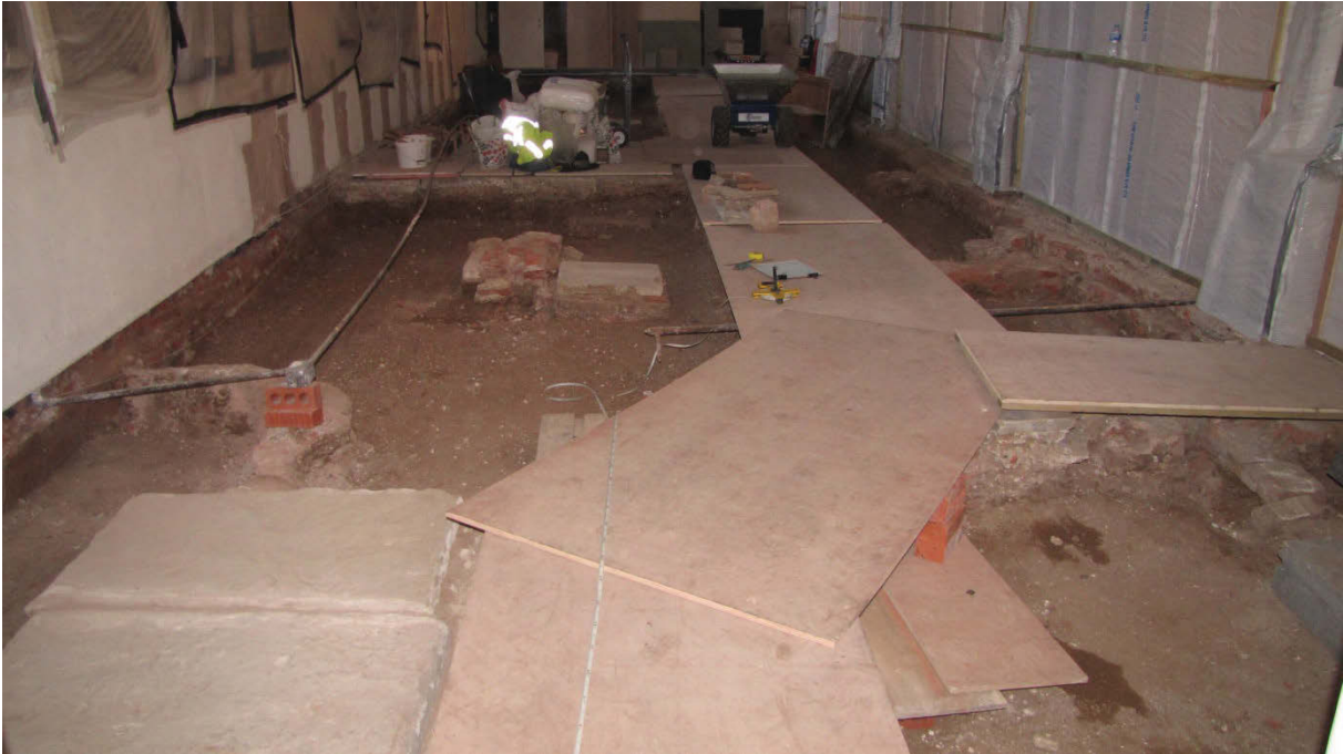
Photo 2 North aisle looking east showing walls [16], [18] and [21] in the middle distance
