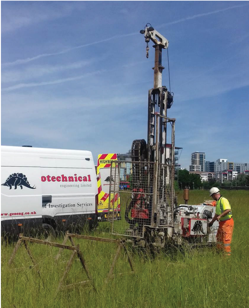
Photograph 1 Drilling rig in position at GA6
