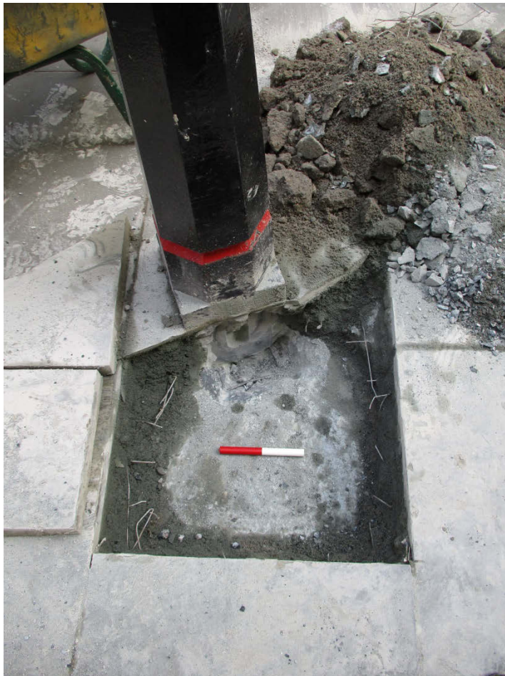
Test hole 6E looking north (0.2m scale)
