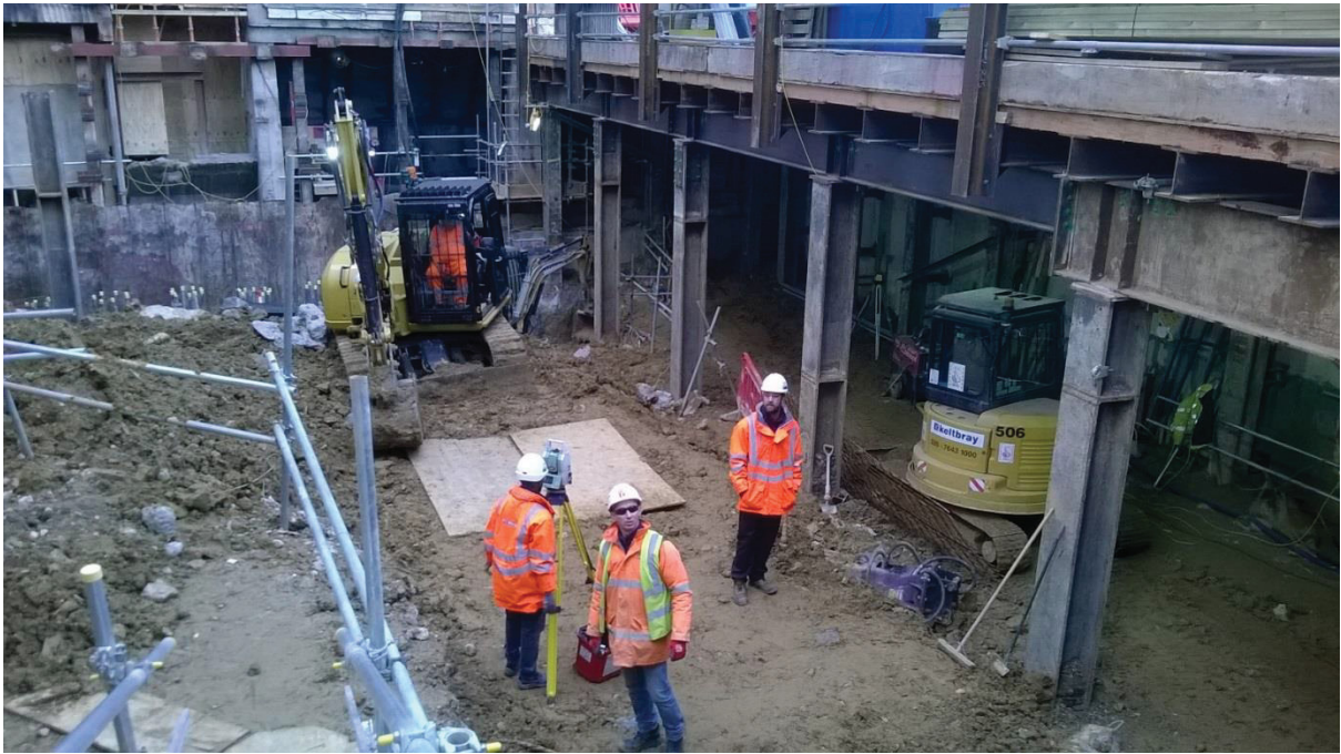
Fig 5 Central area of site looking west during ground reduction
