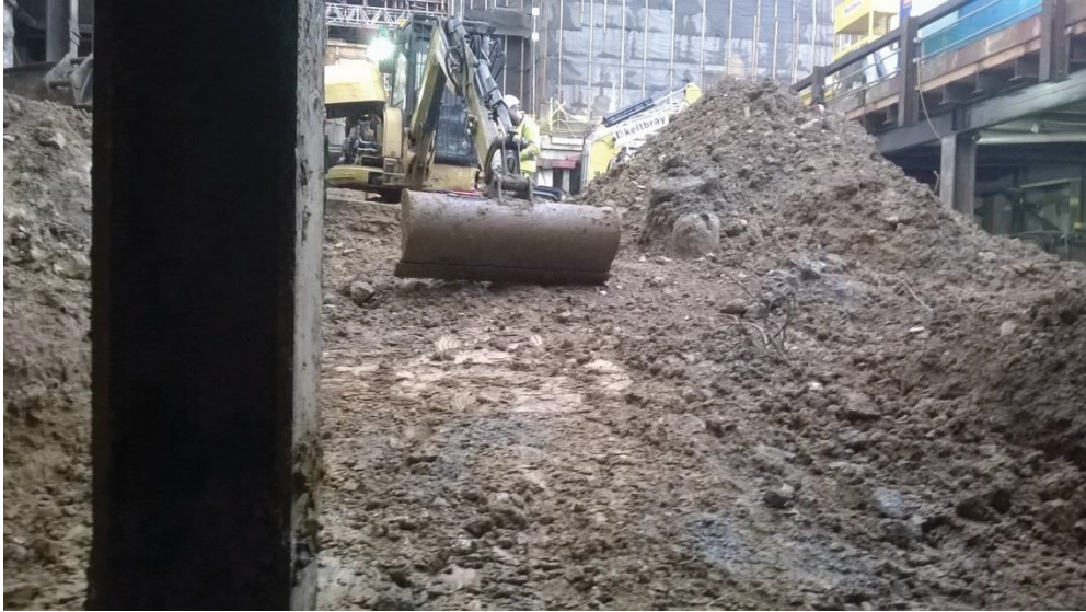
Fig 7 Ground reduction towards south of site looking west
