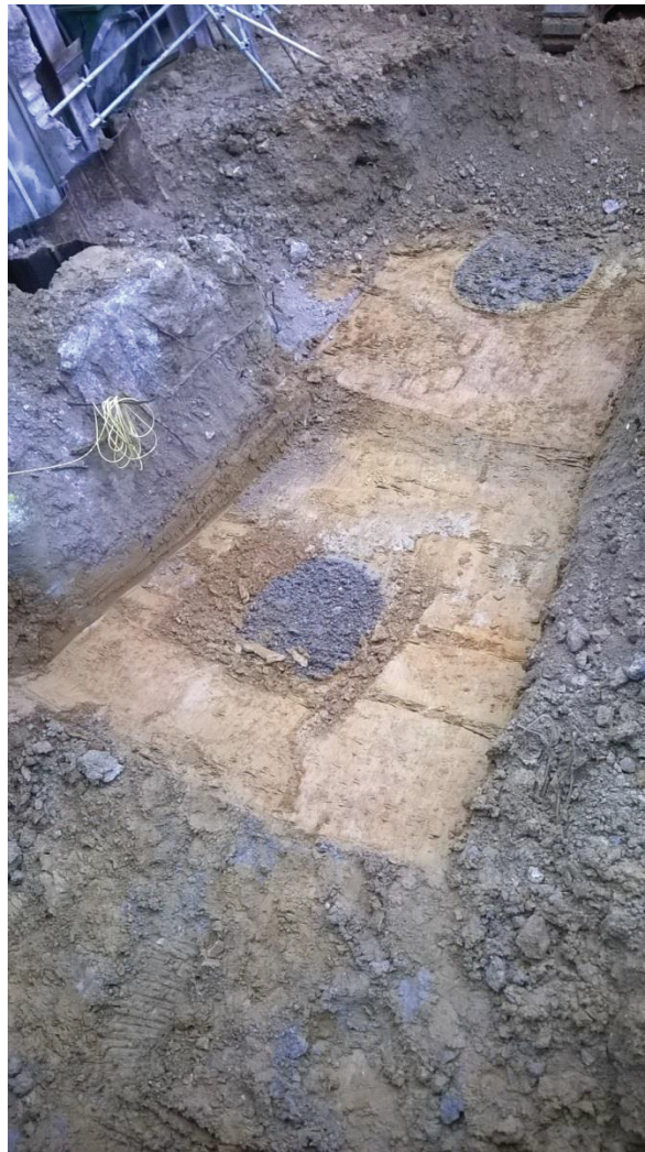
Fig 8 Alluvial deposits beneath redeposited made ground and modern pile holes (from ground level)
