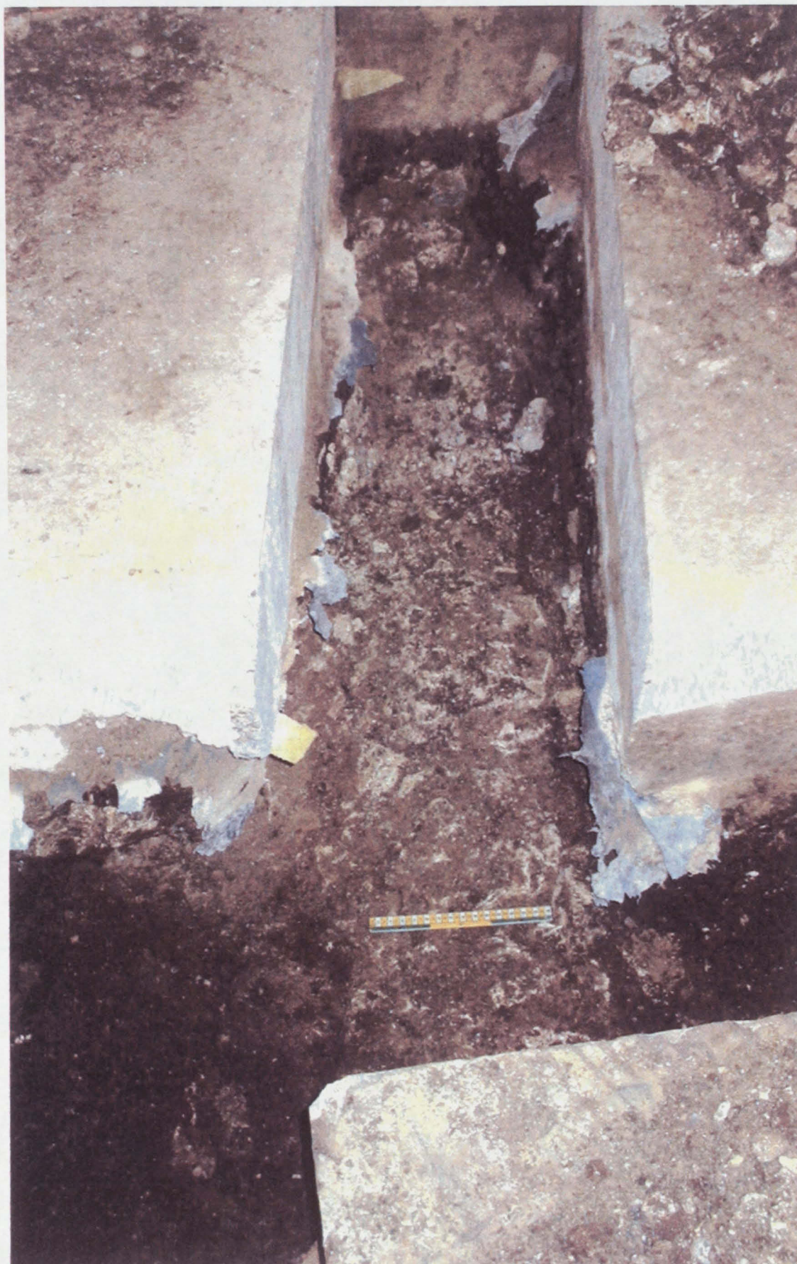
Fig 6 Medieval foundation [9], looking west
