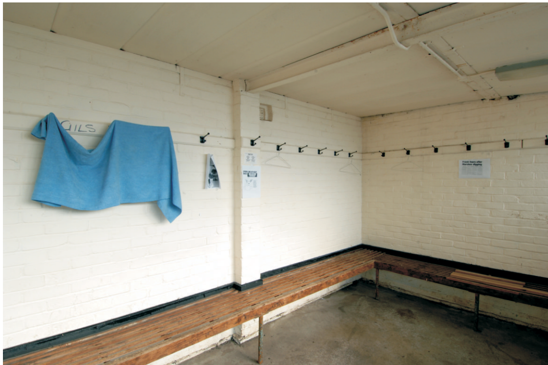
Fig 19 Interior of changing room 15, looking east
