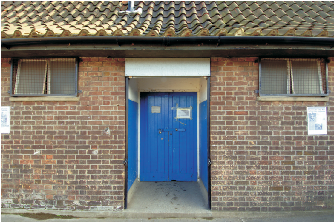
Fig 11 Entrance door to the main range, looking south-east
