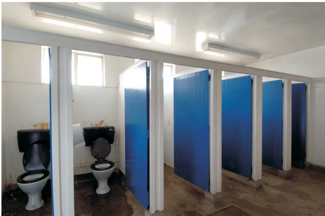
Fig 13 Lavatories in the main range, looking south-east
