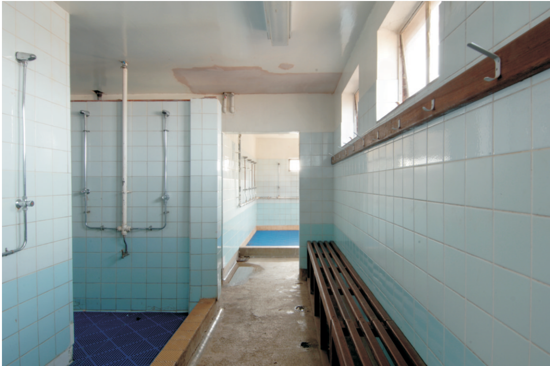
Fig 14 The showers in the main range, looking south-east
