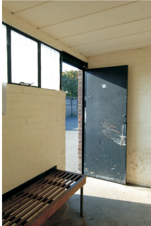
Fig 18 Entrance of changing room 15, looking north-east
