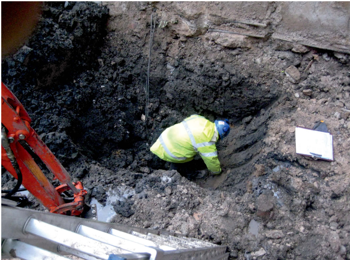
Fig 4 Testpit 10 (view from the north)
