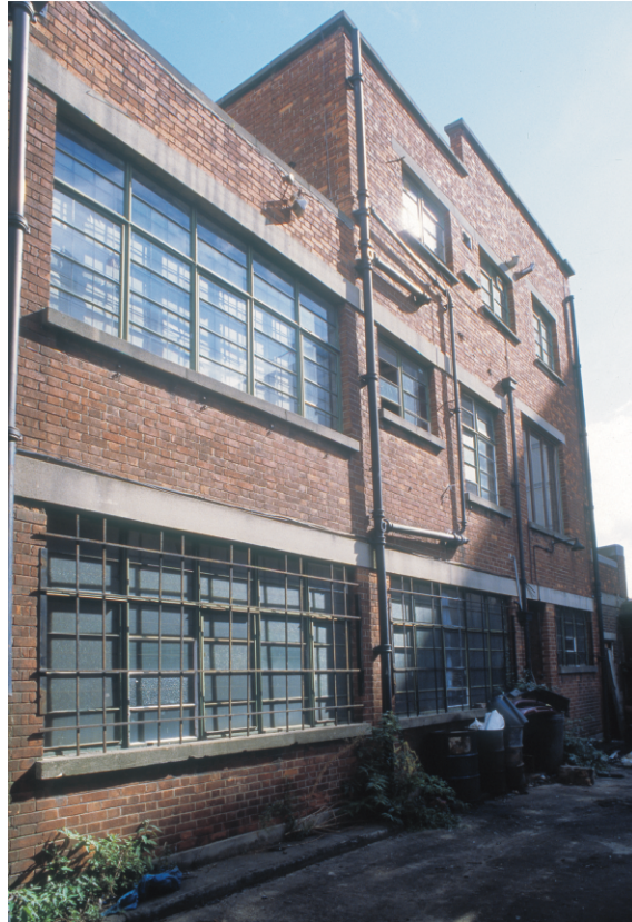
Fig 14 The west facing external elevation, looking south-west
