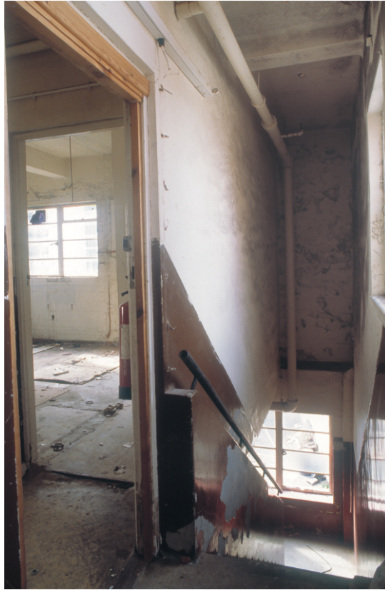
Fig 20 1F4, and the staircase from UG7, looking west
