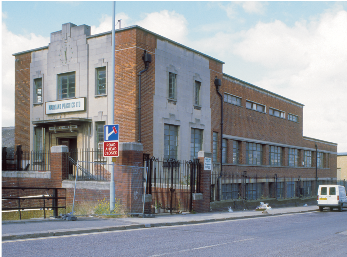
Fig 12 Exterior of 7 Pudding Mill Lane, looking north
