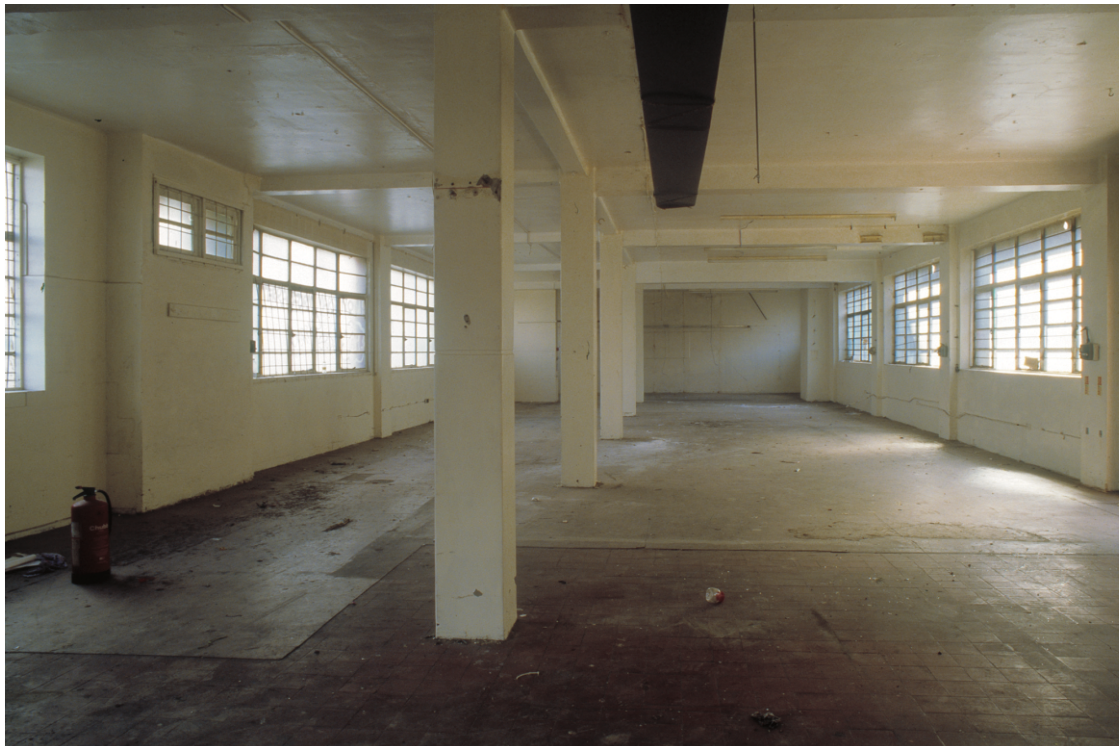
Fig 15 Interior of LG1, looking south
