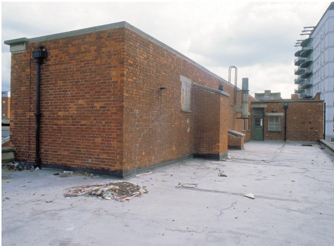
Fig 21 The roof and the exterior of the 1st floor, looking south-east
