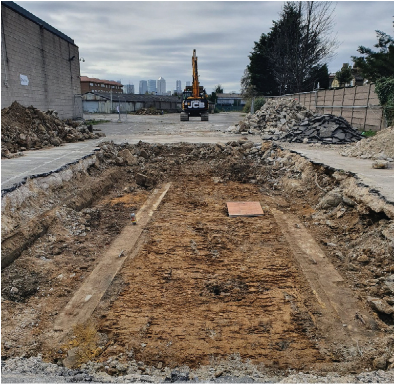
Photo 1 19th century rails cutting through natural brickearth in Trench 1, facing south-west
