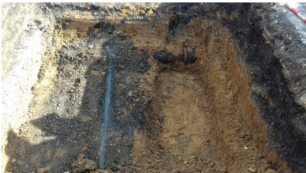
Photo 6 Sondage at north-west end of TR6, facing south-east
