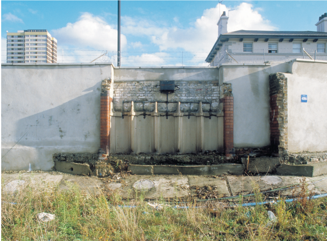
Fig 15 Site of the Men's lavatories on the north side of No. 2 Entrance Gate, looking east
