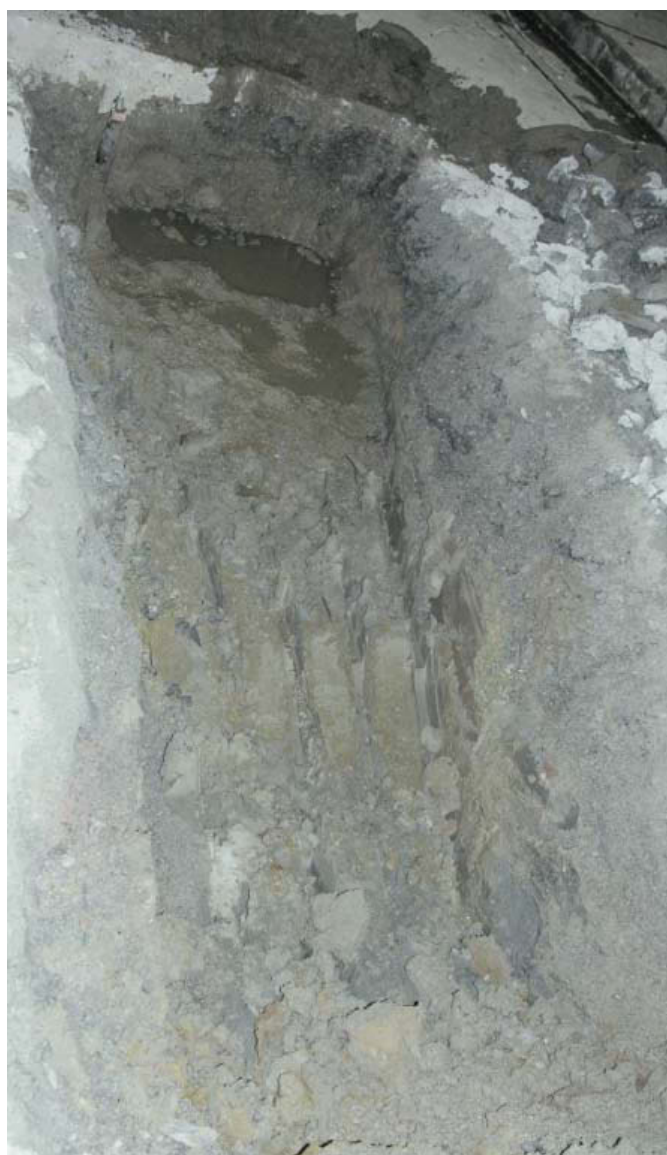
Fig 5 Trial Pit C looking Southwest, during excavation. A toothed bucket was required to excavate into London Clay (to ensure it was not redeposited). It oxidised in contact with the air due to the action of surface water
