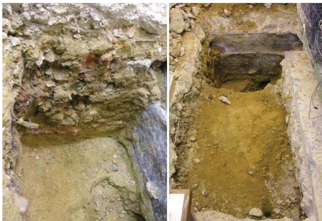
Fig 9 Trial pit 7 looking southwest (left) and northwest (overview right) The natural sand is overlain with clay and concrete from 1950s construction
