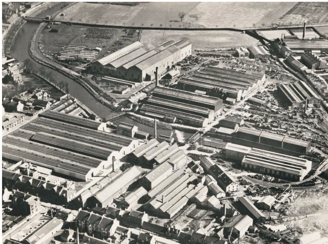
Fig 5 The Glenfield & Kennedy works, Kilmarnock, East Ayrshire (© East Ayrshire Council)
