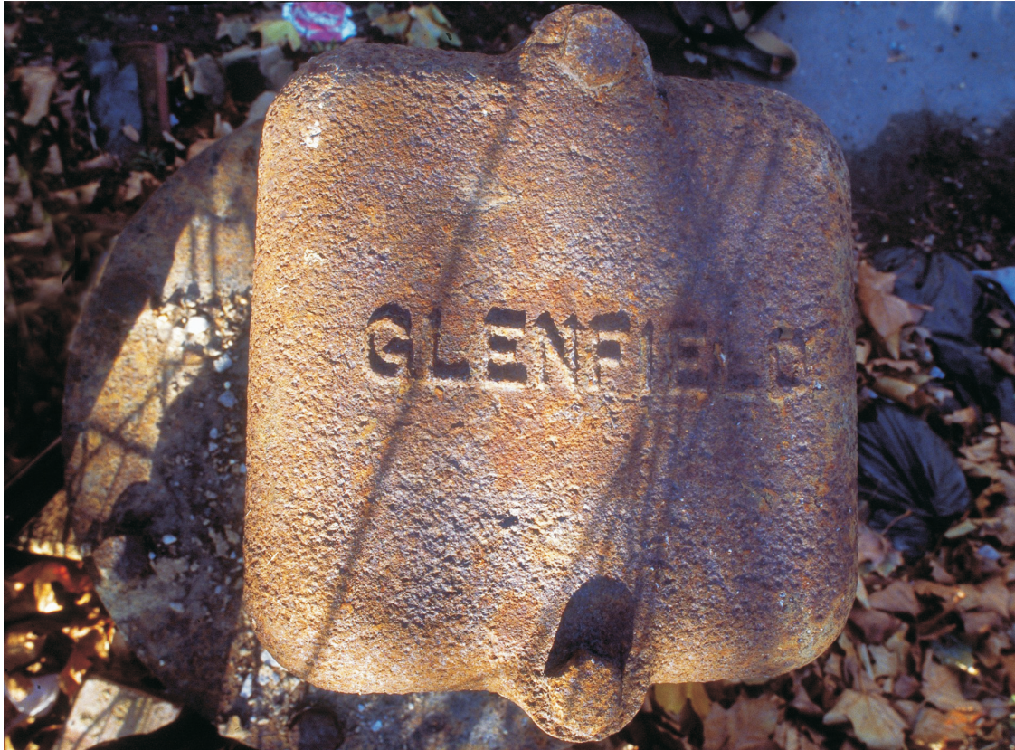
Fig 8 Flanged top plate of the single orifice air valve, with maker's name cast into the fabric
