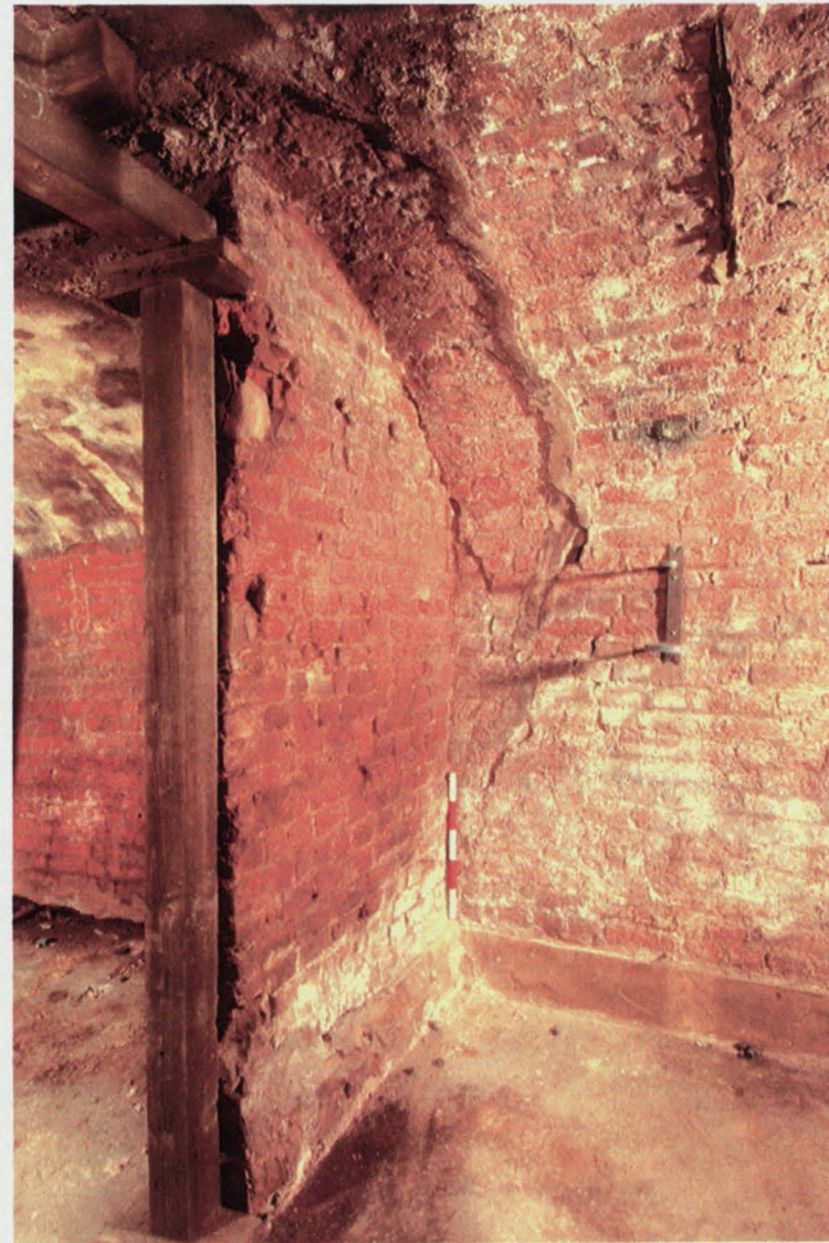
Fig 18 Detail of partition cross-wall of eastern cellar, looking northeast
