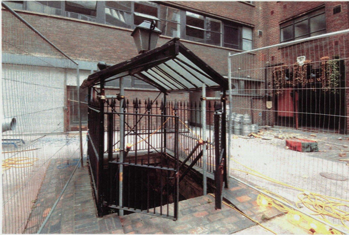
Fig 13 Top of steps to cellars, in Mitre Court, looking northwest
