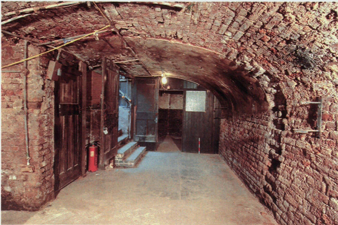
Fig 22 Western cellar, looking south
