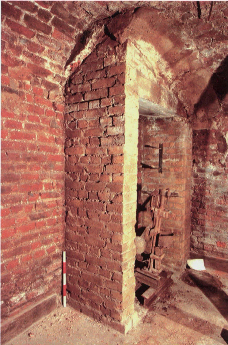
Fig 19 Brick buttresses (with bottling machine) at south end of eastern cellar, looking southwest
