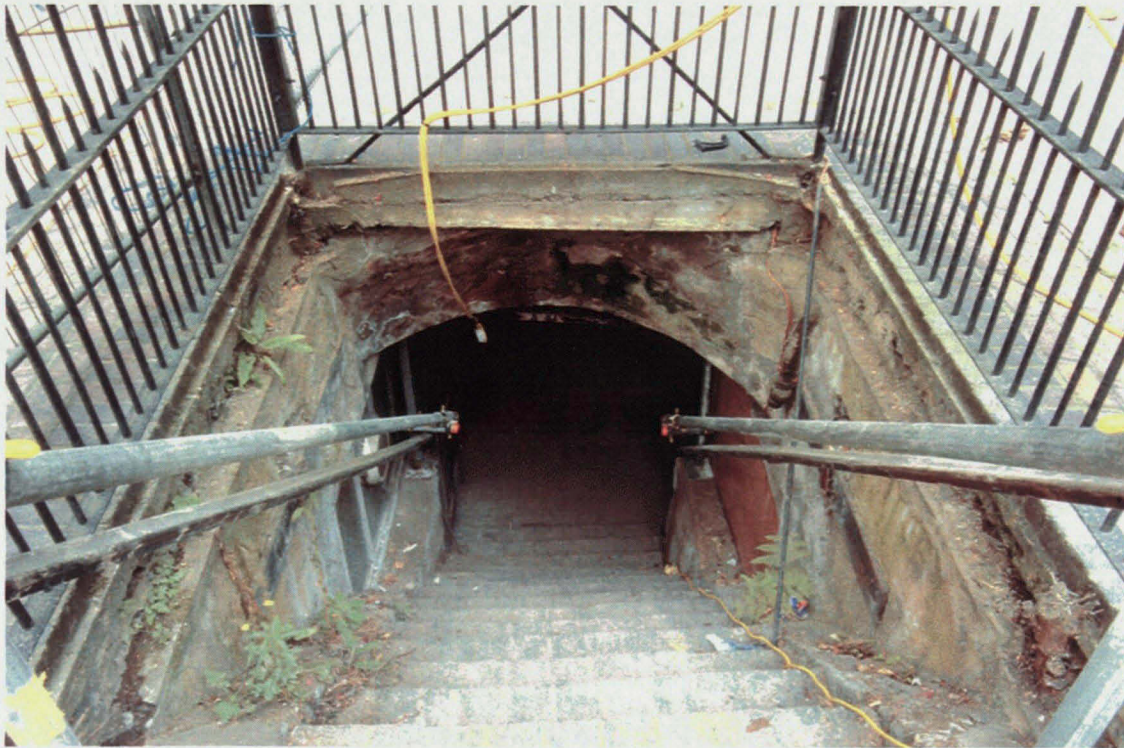
Fig 14 Looking down steps to western cellar from Mitre Court
