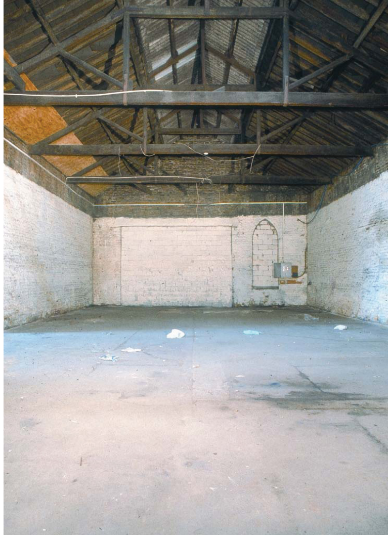
Plate 7 Interior of Unit 6, looking south (MoLAS 374/07/02)
