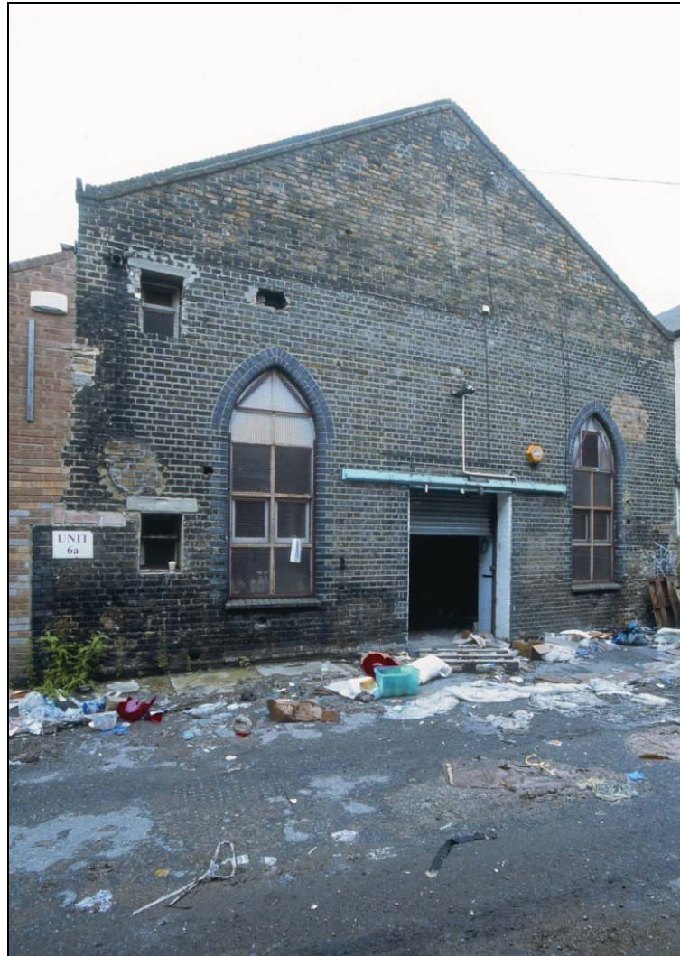
Plate 5 Exterior of Unit 6a, looking west (MoLAS 318/07/017)
