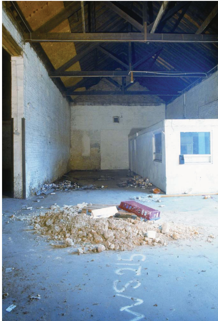
Plate 6 Interior of Unit 5, looking north (MoLAS 374/07/01)
