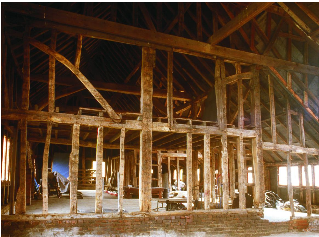
Fig 11 The west gable end of phases 1 and 2 of the barn
