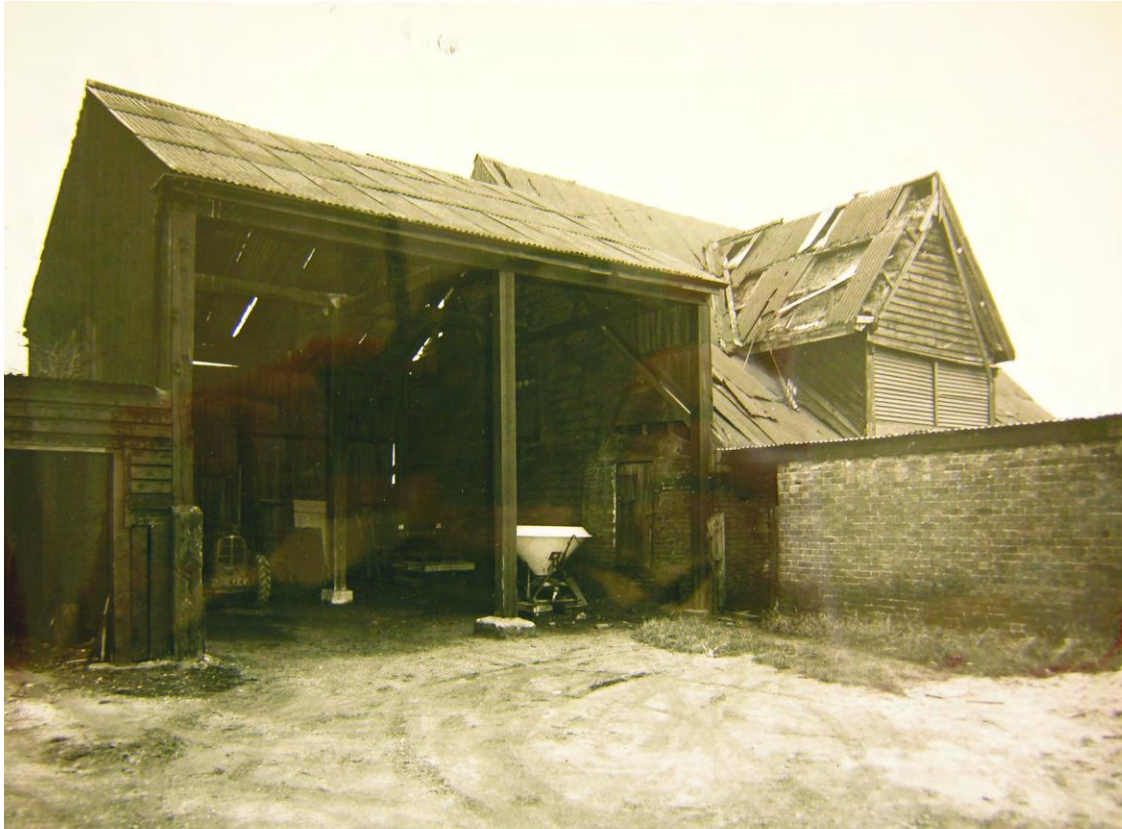
Fig 8 The barn at Albys Farm in the mid 20th century
