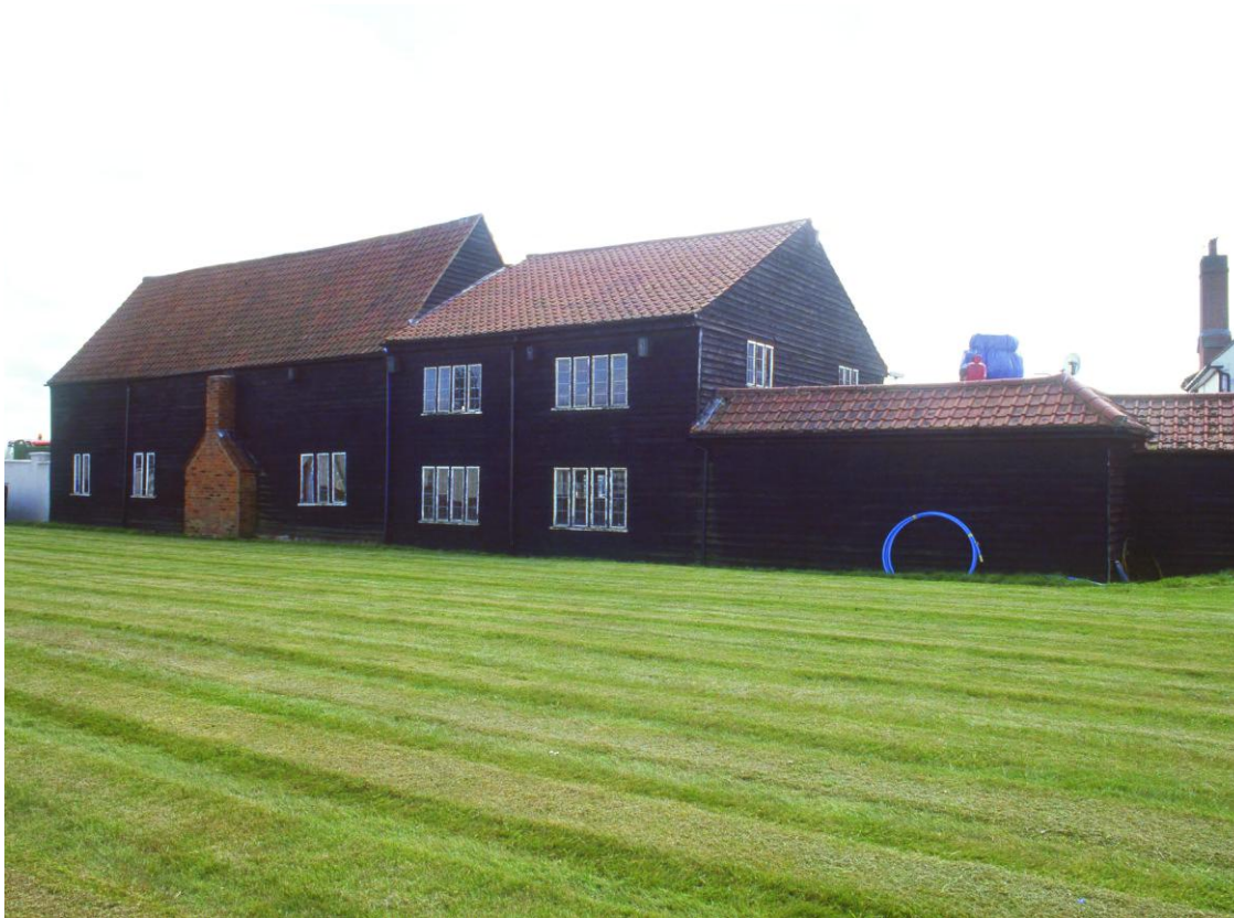
Fig 10 The north-facing external facade of the barn
