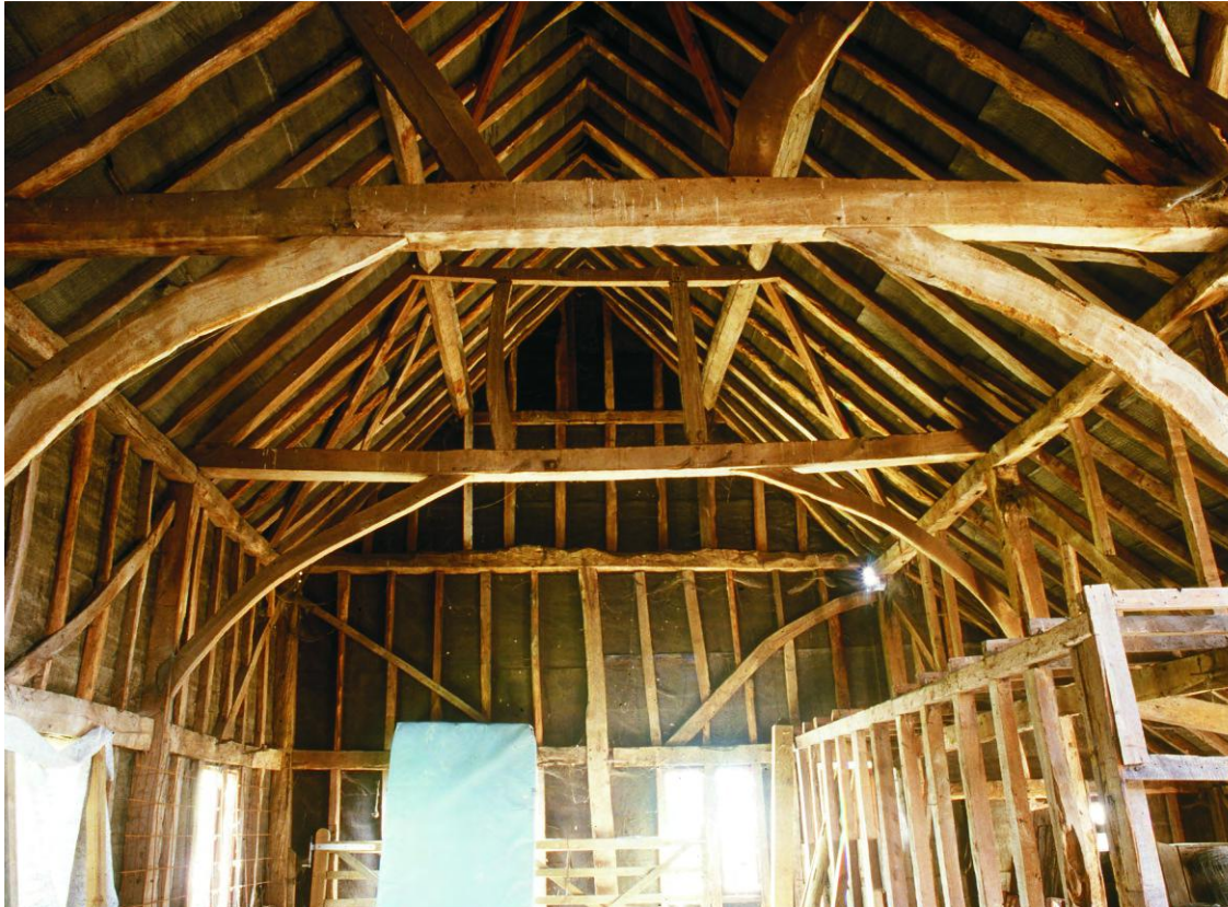
Fig 12 The roof trusses C and D, looking east
