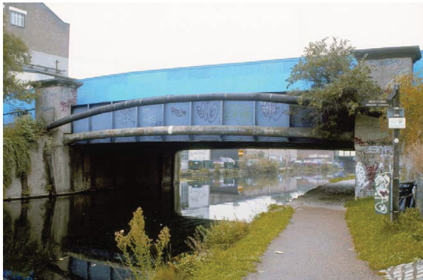
Plate 14 The northern side of White Post Lane Bridge, looking south (40707014)
