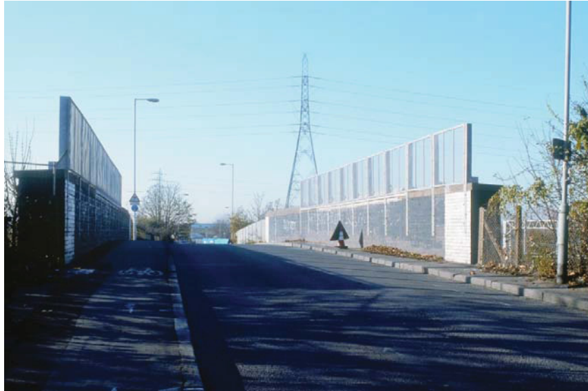
Plate 17 The eastern approach to Temple Mill Lane Bridge, looking west (43707001)
