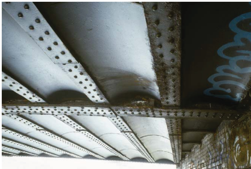
Plate 15 The underside of White Post Lane Bridge, looking south (40707016)
