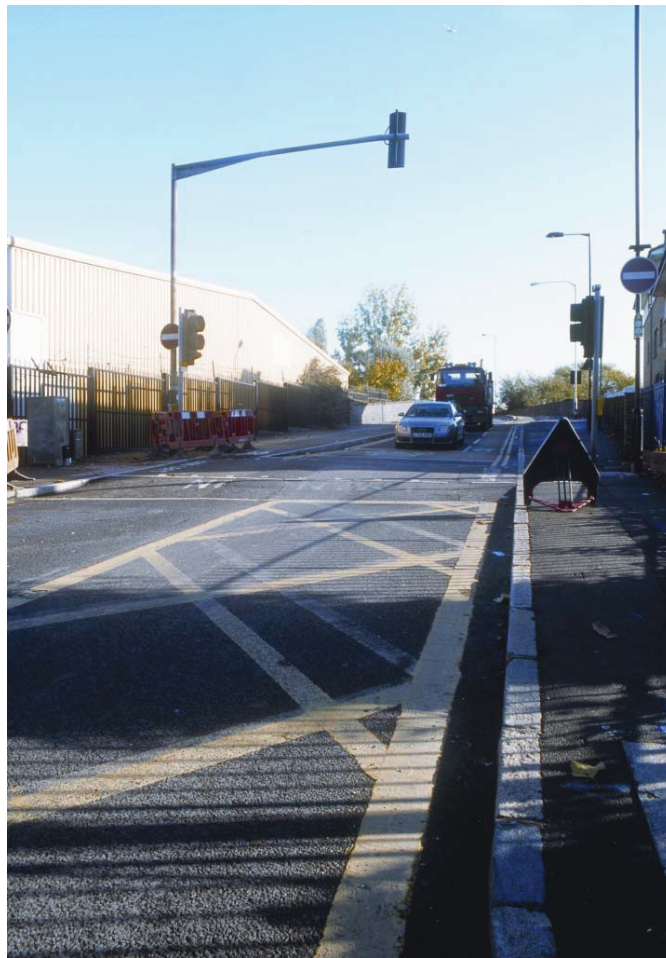
Plate 4 The western approach to the Eastway Bridge, looking east (39507004)
