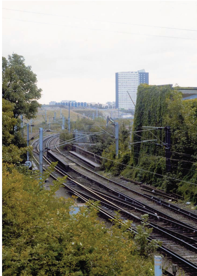
Plate 10 The railway line beneath The Waterden Road Bridge, looking east (34607013)
