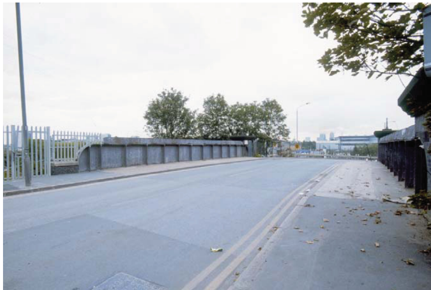
Plate 9 The northern approach to The Waterden Road Bridge, looking south (34607001)
