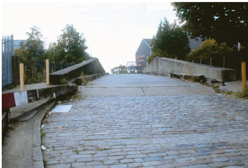
Plate 6 Eastern approach to Bridgewater Road Bridge, looking north-east (34707003)
