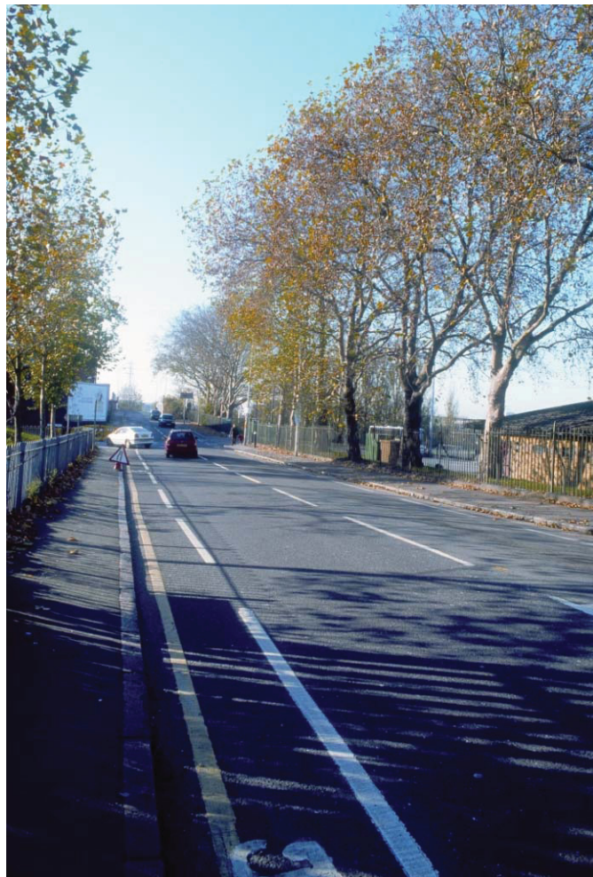
Plate 18 The eastern approach road to Temple Mill Lane Bridge, looking west (43707009)
