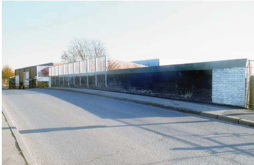
Plate 19 The southern parapet wall of Temple Mill Lane Bridge, looking east (43707003)
