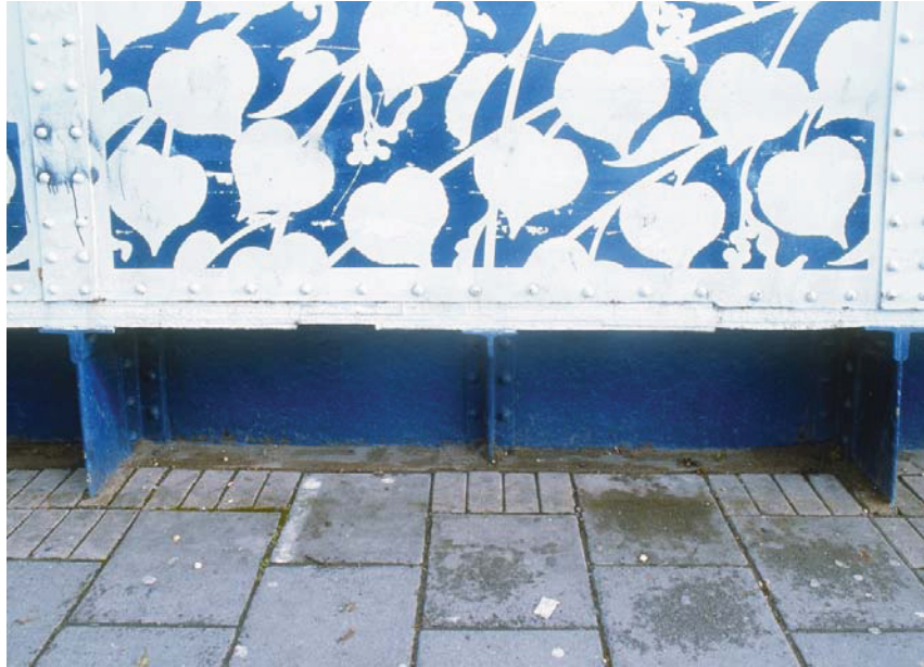
Plate 22 Part of the riveted east parapet wall, looking east (45407004)
