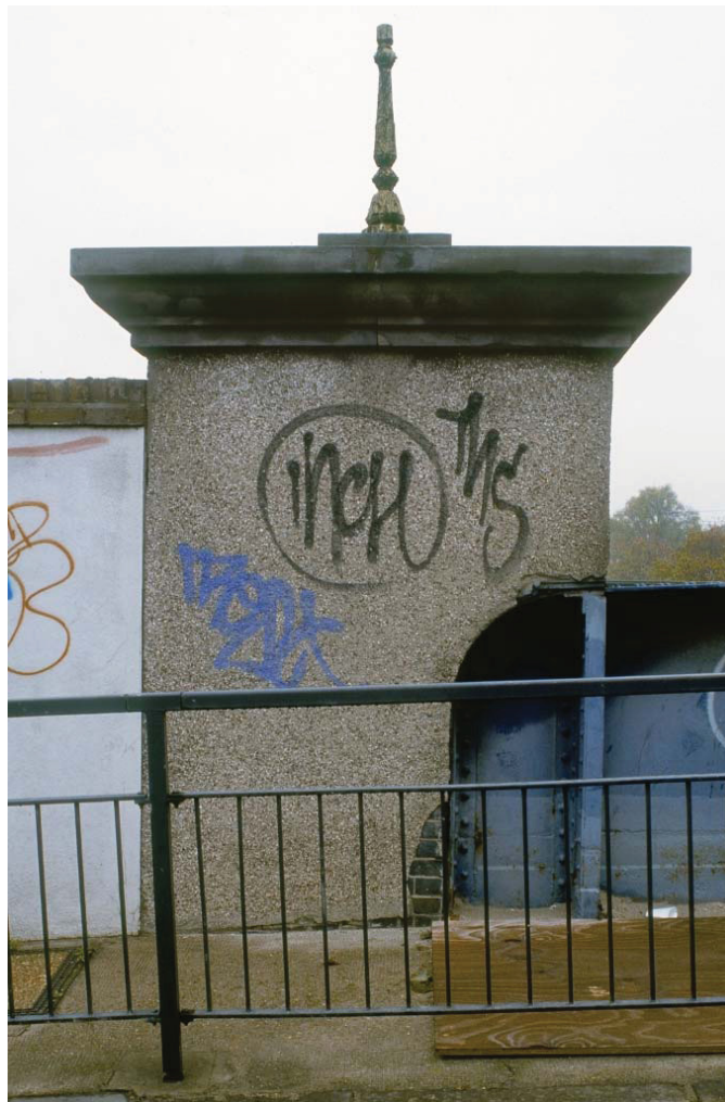
Plate 16 The north-west bridge pier, White Post lane, looking north (40707009)
