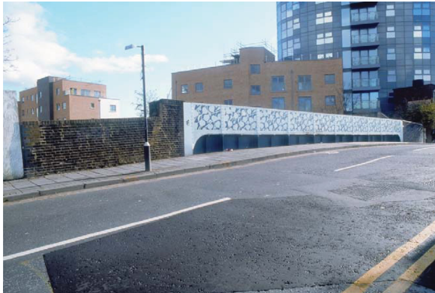
Plate 20 The east parapet wall of Angel Lane Bridge, looking south-east (45407001)
