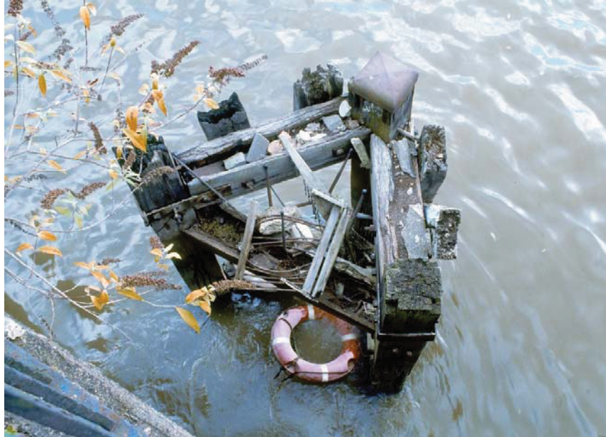
Plate 7 Disused footings of The Bridgewater Road Bridge in the Waterworks River (34707009)
