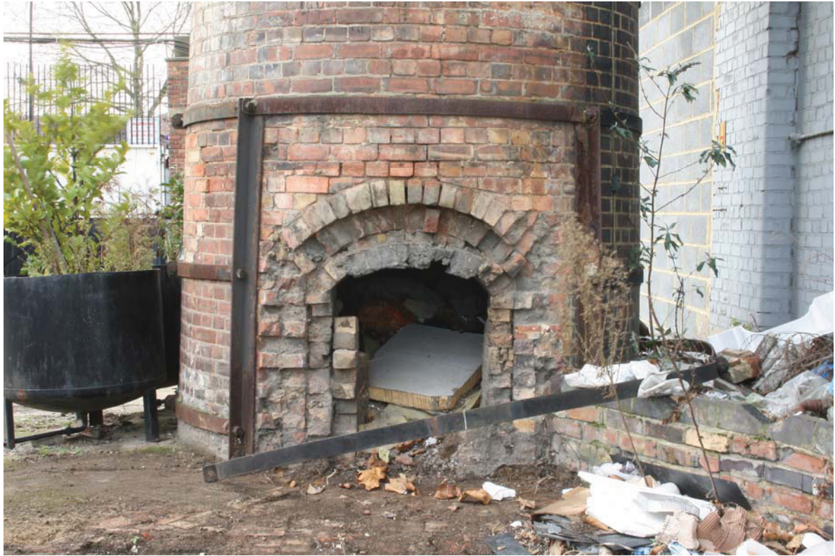
Plate 4 View looking W of the chimney opening (13)
