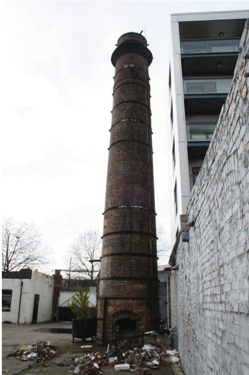
Plate 3 View looking W of the chimney with lightning conductor (21)
