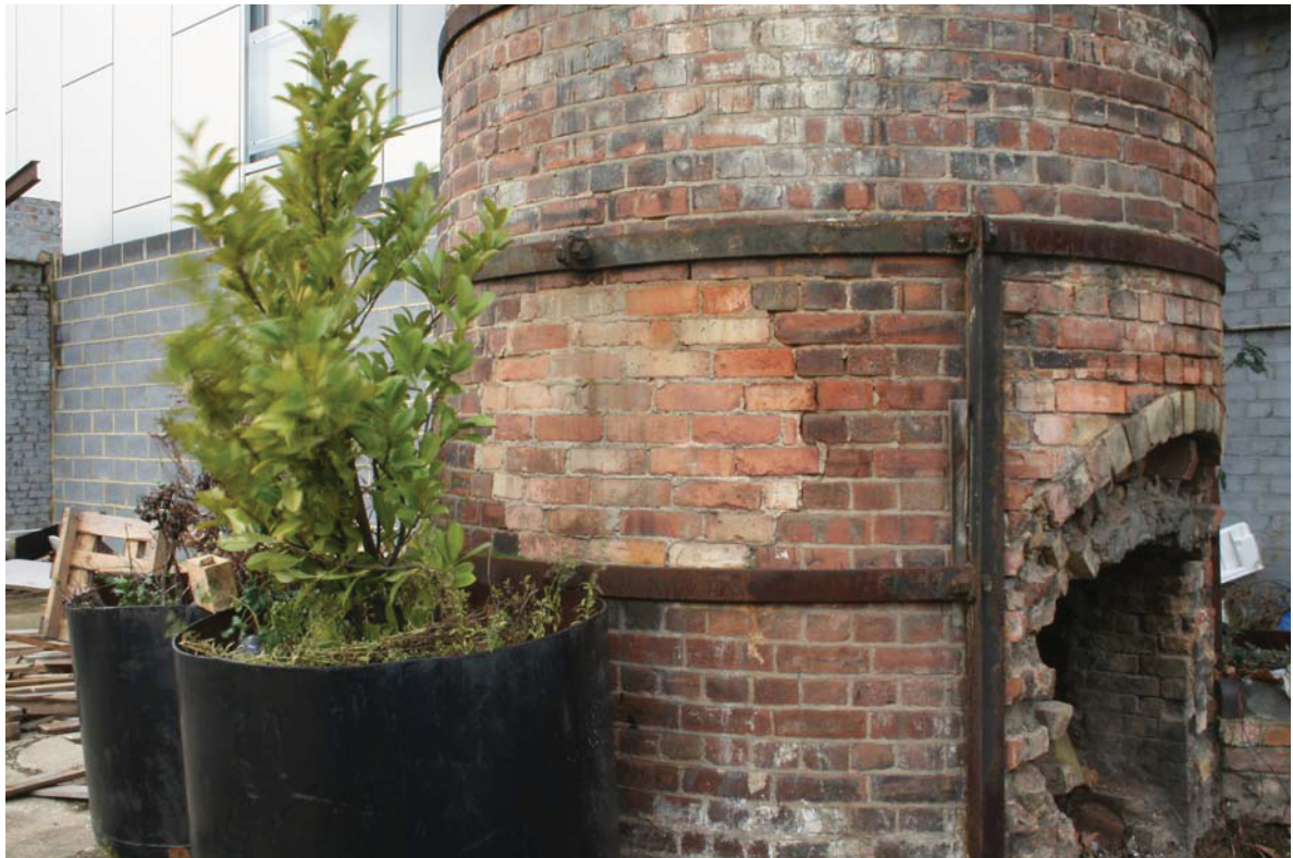
Plate 7 View looking NW of blocked-off inspection window (16)
