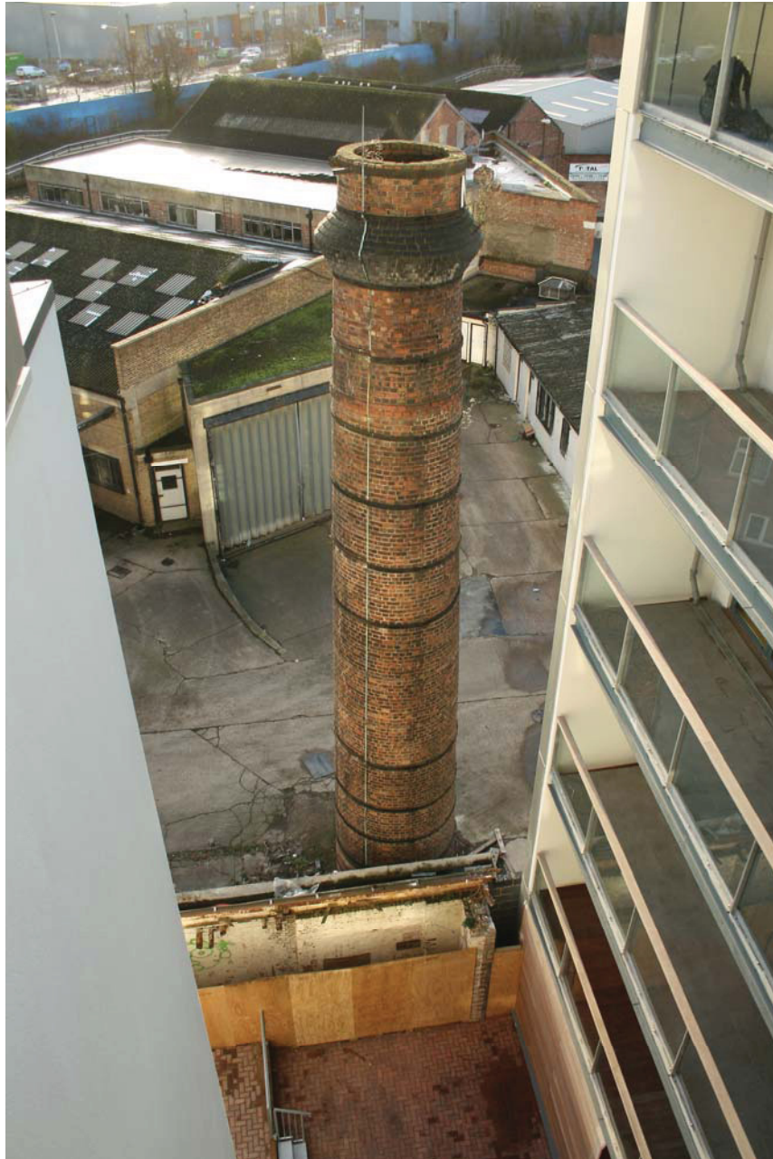
Plate 2 View looking SE of the chimney from the adjoining building (3)
