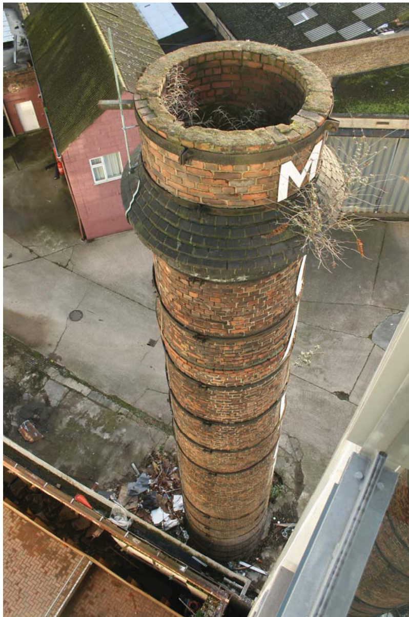
Plate 8 View looking E of the chimney from the adjoining building (2)
