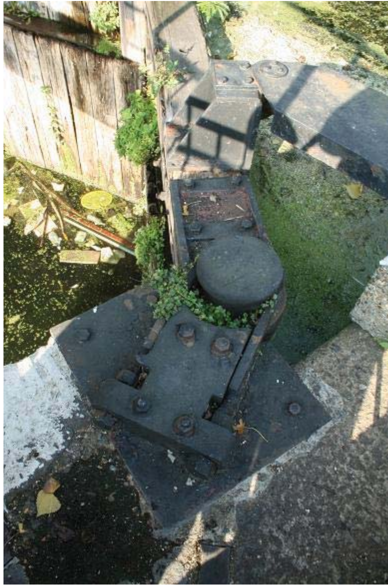
Plate 53 Detailed view of mechanism and hinge of the west chamber's south gate, Old Ford Locks: OL-05007
