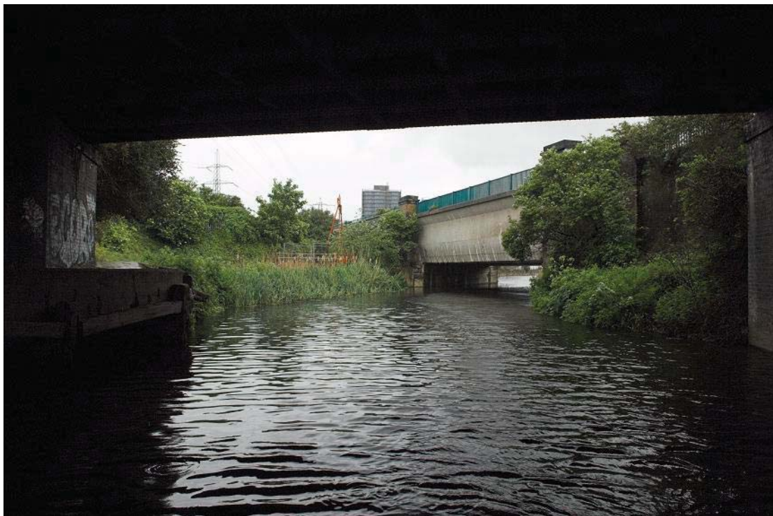
Plate 29 View of mooring area between GNER bridge and Northern Outfall Sewer bridge, City Mill River, looking south-east: OL-01207
