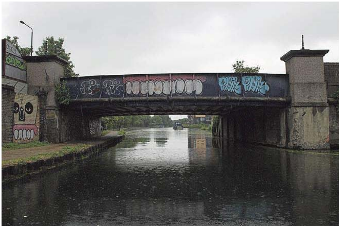
Plate 14 View of White Post Lane bridge spanning the Lea Navigation, looking south: OL-01207
