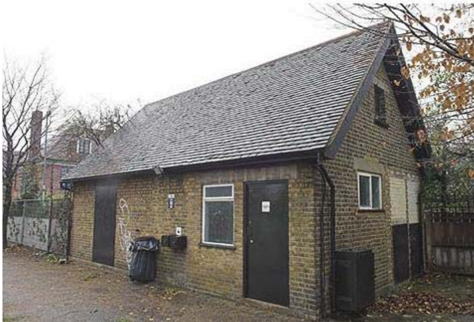
Plate 46 Oblique view of west elevation of stables relating to the Old Ford Lock Houses, looking south-east: OL-07307
