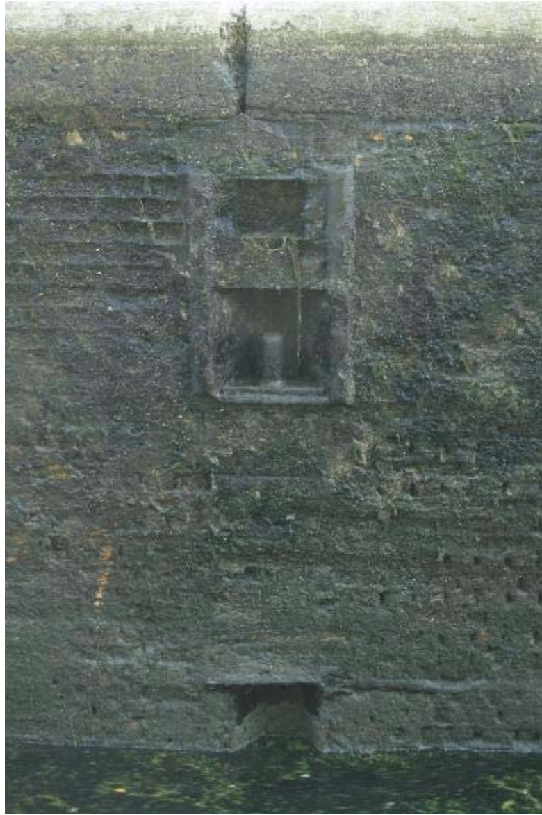
Plate 54 View of mooring hook set into east wall of east chamber, Old Ford Locks, looking east: OL-05007
