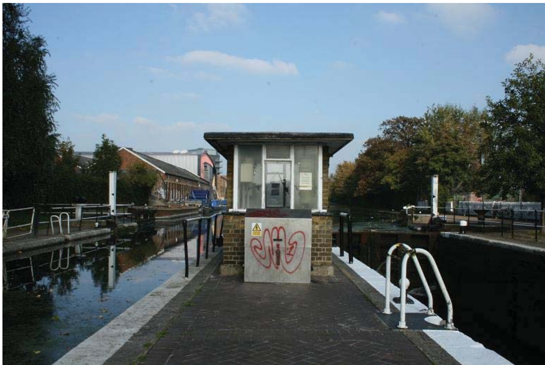
Plate 51 View of central island of Old Ford Locks, showing control booth, looking north: OL-05007
