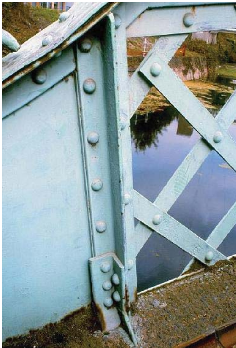
Plate 79 Detailed view of junction between steel panel and lattice on north side of City Mill River Footbridge, looking north: OL-03507
