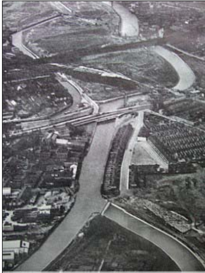
Plate 6 View of the improvements made under the Lea and Back Rivers scheme: Three Mills River and flood channel in foreground, Waterworks River to the right (north of High Street) and City Mill River to the left with Groves Bridge in the centre, 1936 (LD PEM PS 159/0719, courtesy of Newham Local Studies and Archive Library): OL-01207
