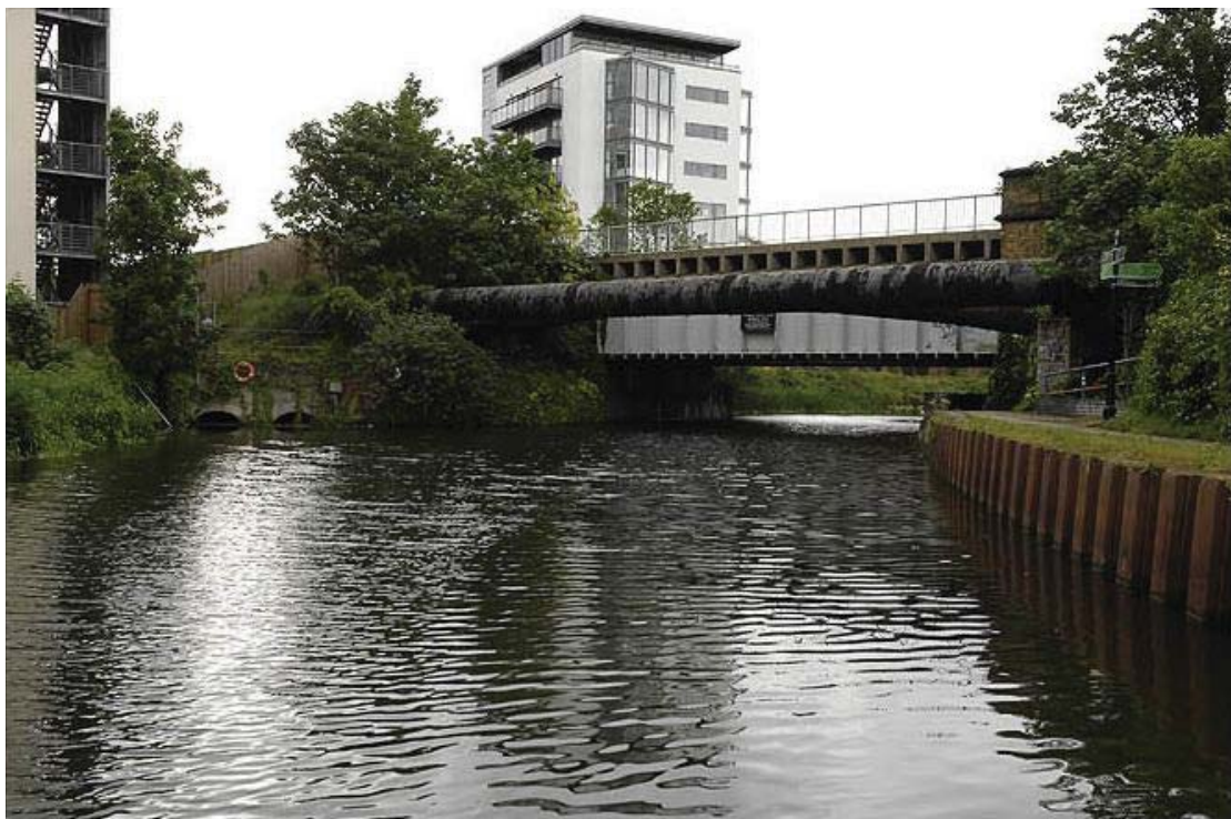
Plate 19 View of Greenway bridge spanning the River Lea with sewage pipes on foreground, looking north-west: OL-01207
