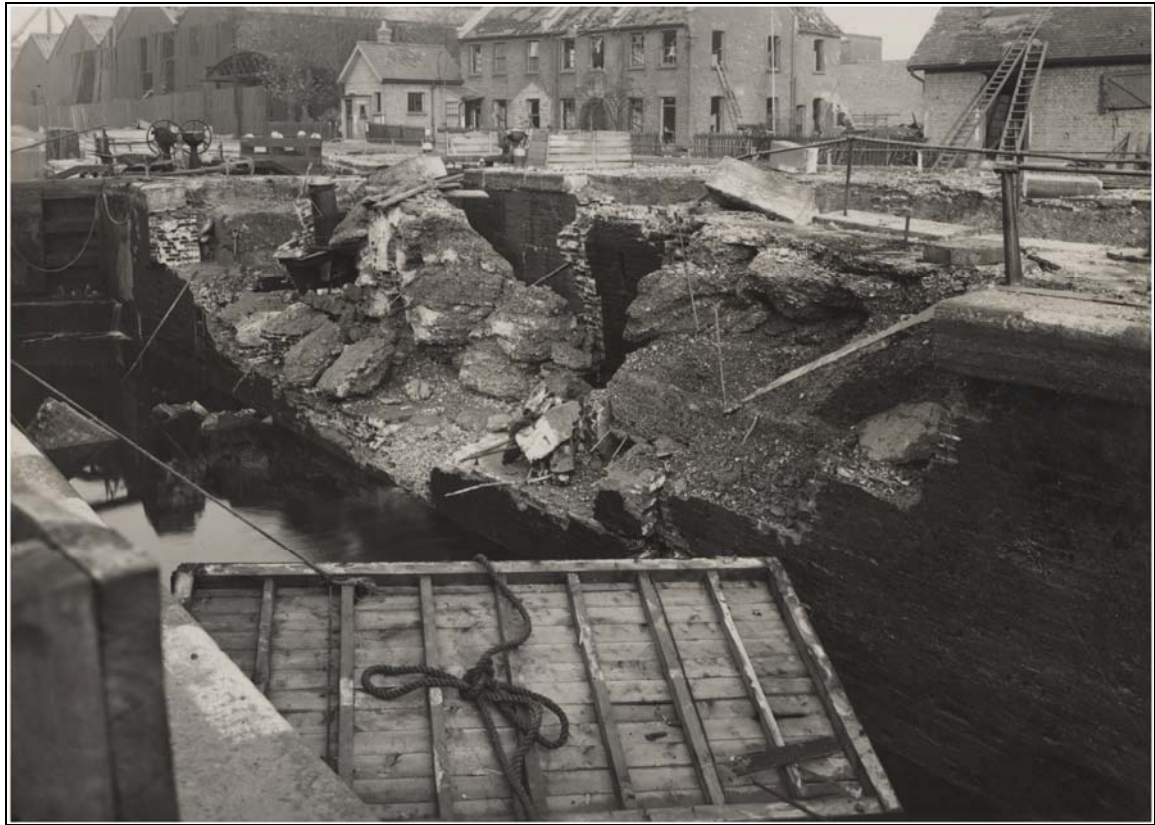
Plate 7 View of bomb damage to central pier at Old Ford Locks, October 1940 (LD PEM PS 159/0976, courtesy of Newham Local Studies and Archive Library): OL- 05007
