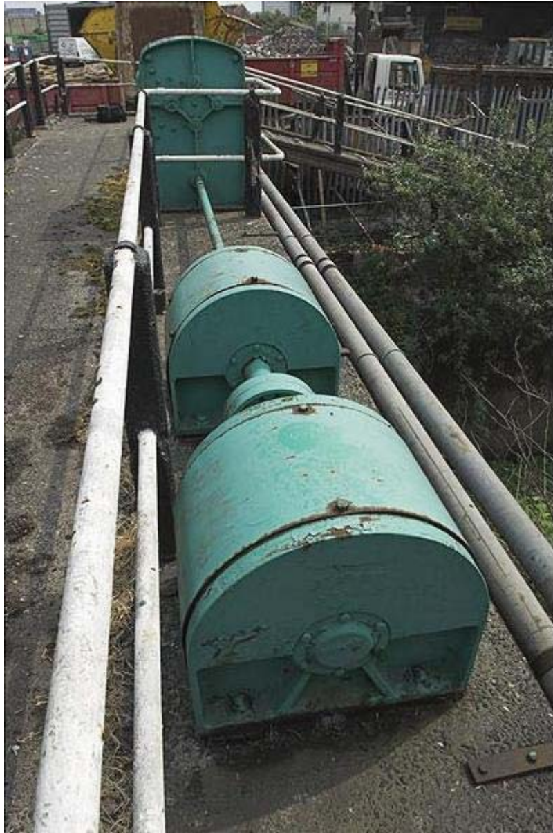
Plate 74 View of original lock mechanisms, Carpenter's Lock, looking east: OL-03007
