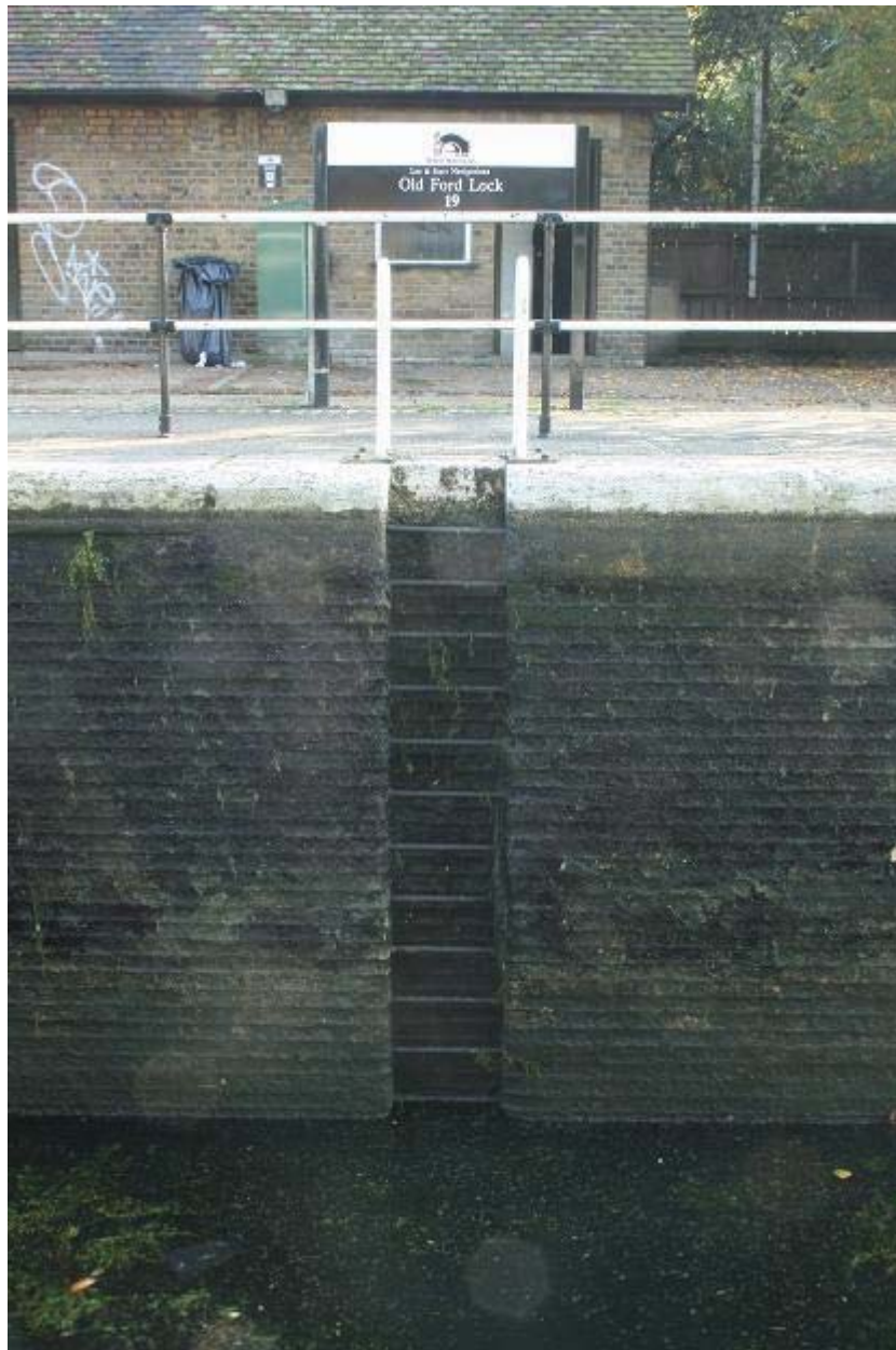
Plate 55 View of ladder set into the recess on the east wall of the east chamber, Old Ford Locks, looking east: OL-05007
