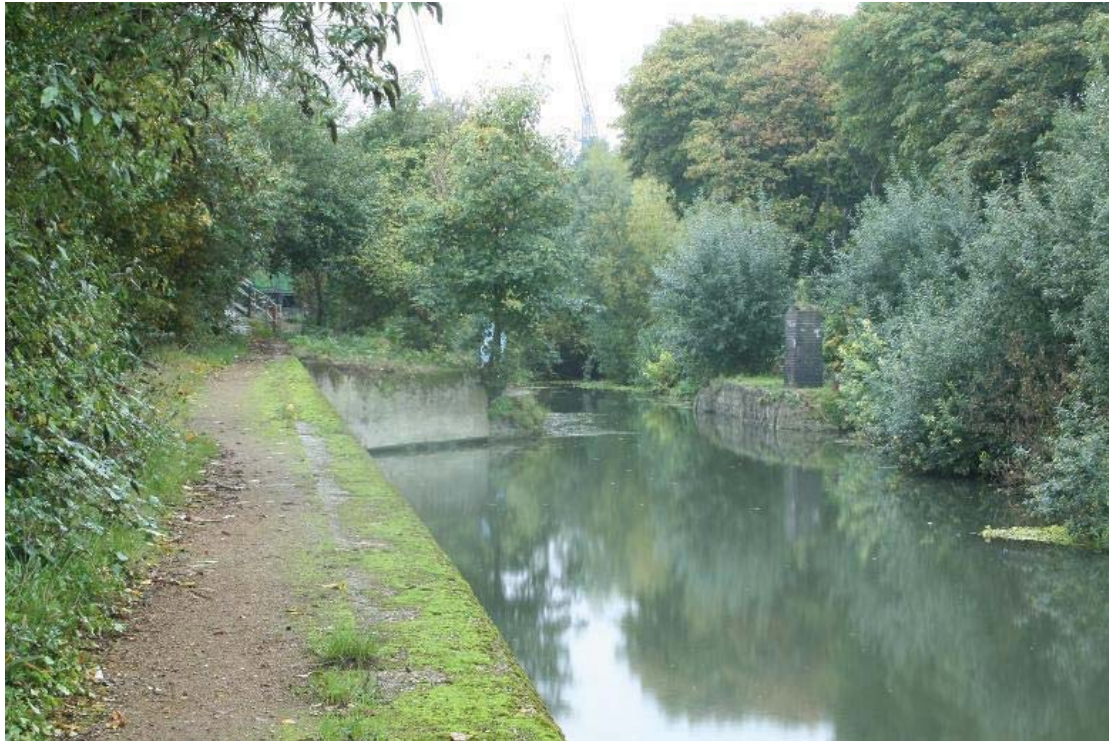
Plate 59 View of Pudding Mill Lock, showing eastern towpath and footbridge in background, looking south-west: OL-05407
