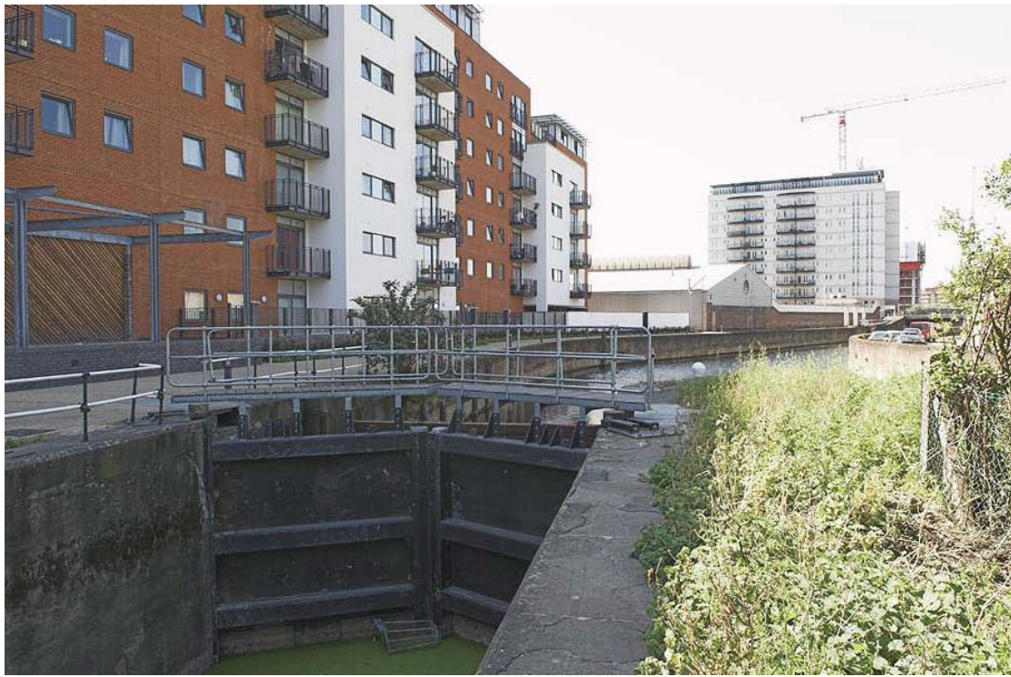
Plate 66 View of south gate of Marshgate Lane Lock, looking south-west: OL-07407
