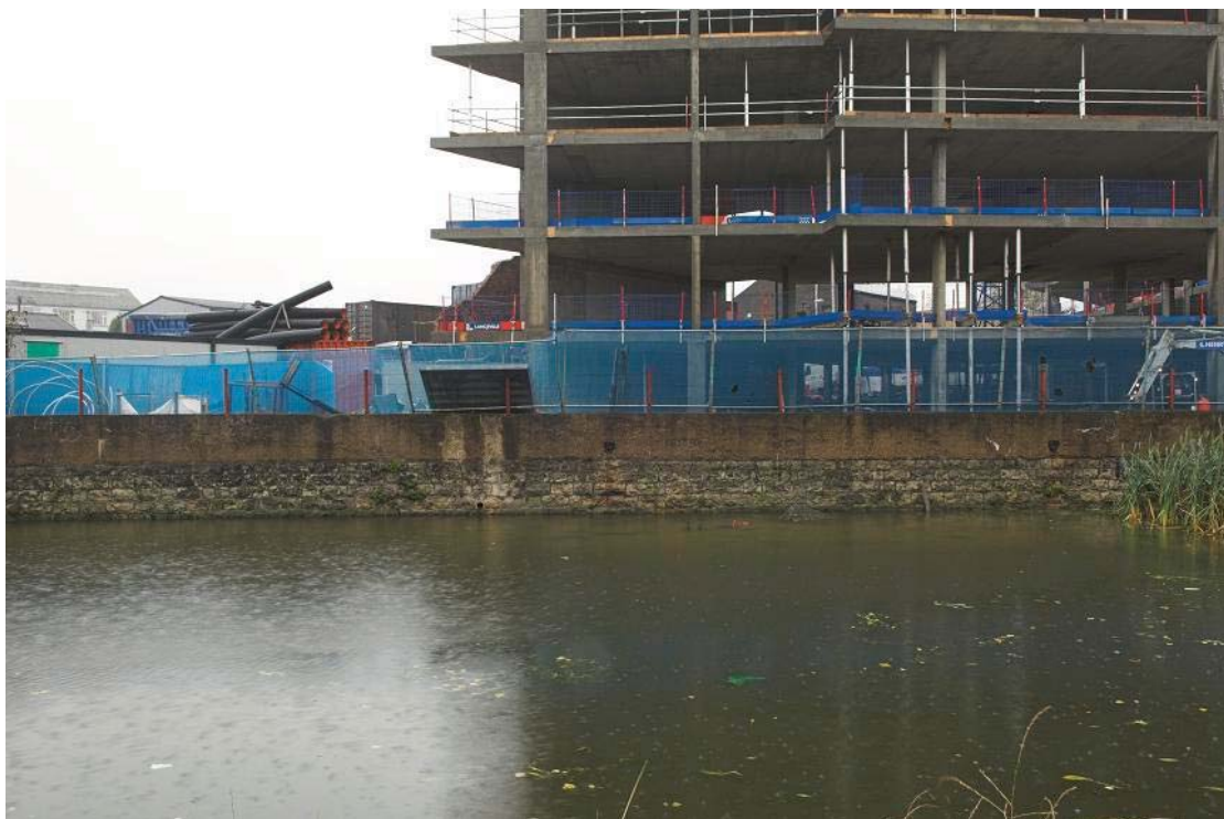
Plate 69 View of continuation of stone and brick riverbank wall, looking west- southwest: OL-07207
