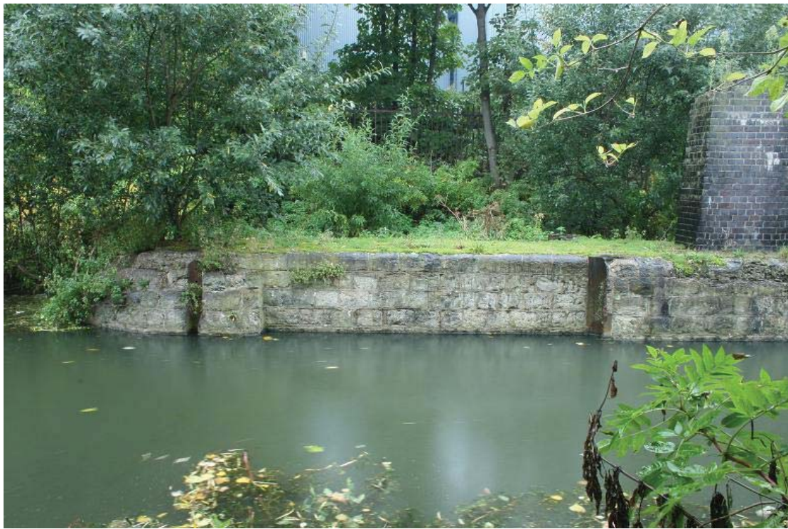
Plate 63 View of lock gate recess on east side of central island, Pudding Mill Lock, looking north-west: OL-05407
