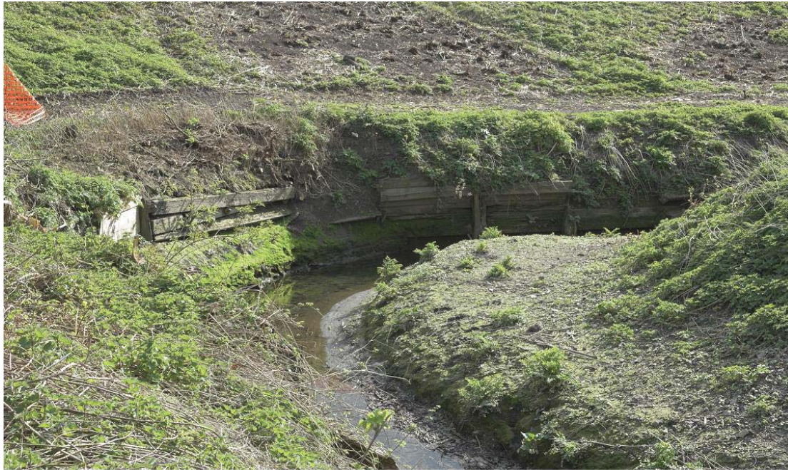
Plate 24 View of curve of Potter's Ditch with timber revetment, looking south-east: OL-02007
