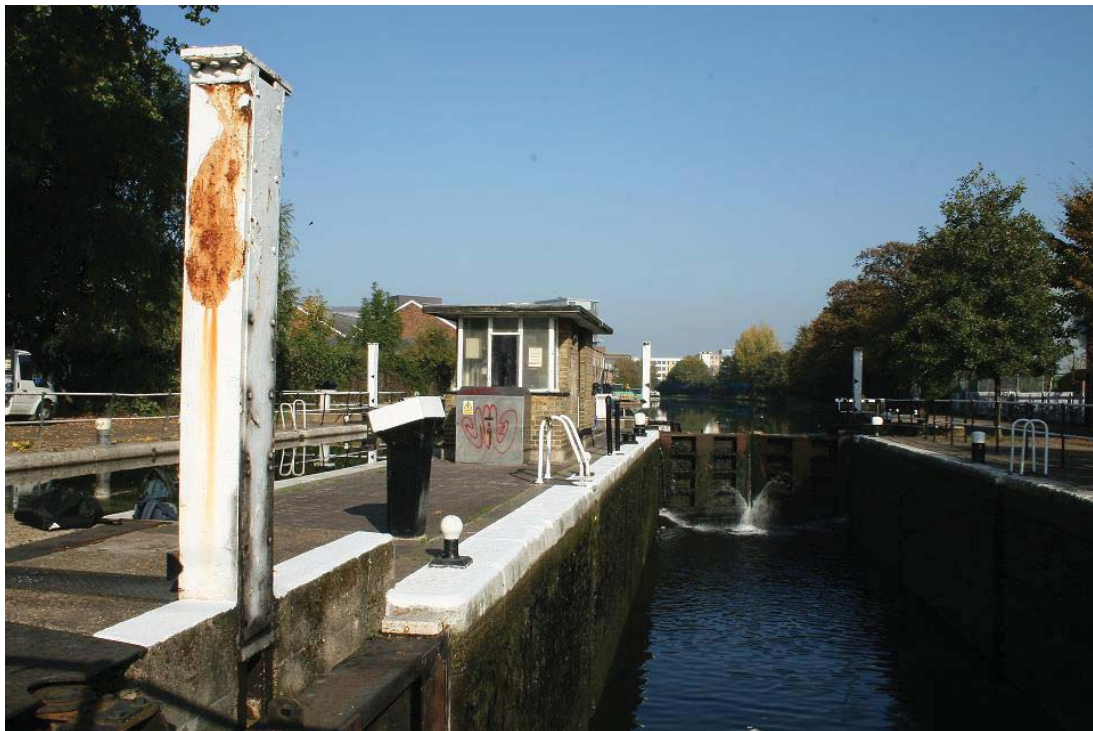
Plate 47 View of central island of Old Ford Locks with clough in foreground, looking north-west: OL-05007
