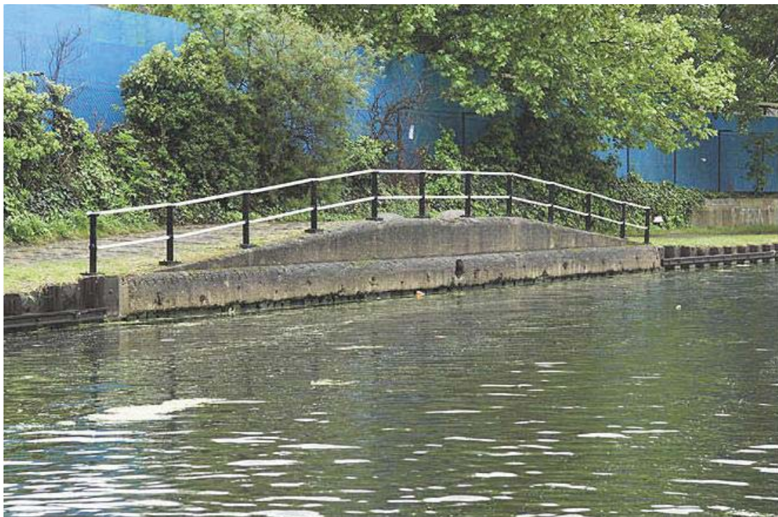
Plate 16 View of first tipping wharf on eastern bank of the Lea Navigation, looking south-east: OL-01207
