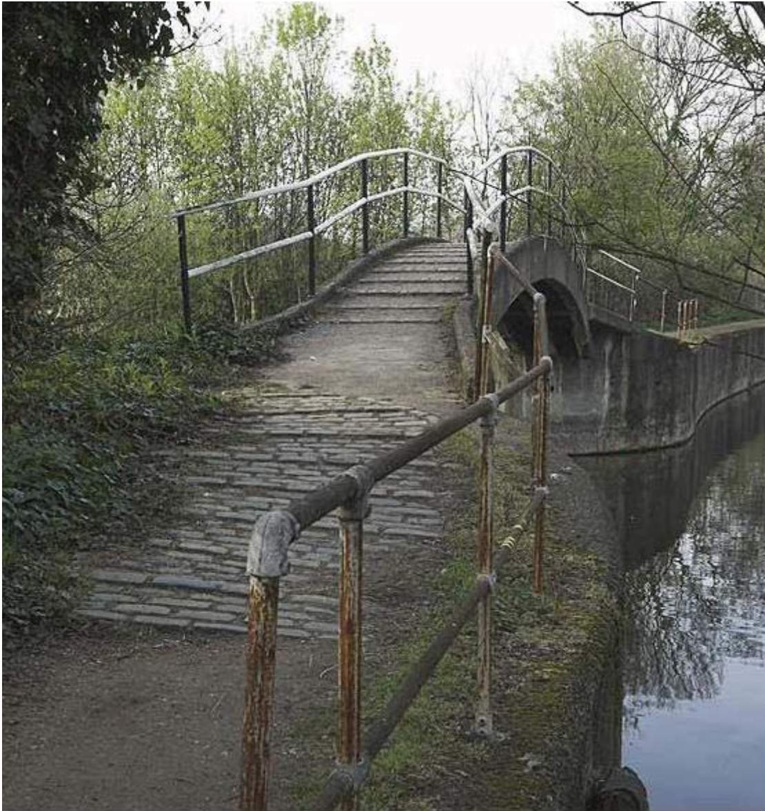
Plate 34 View of northern side of Pudding Mill River footbridge spanning the River Lea, looking south-west: OL-01207
