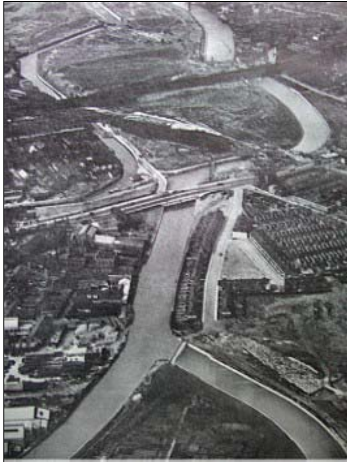
Plate 6 View of the improvements made under the Lea and Back Rivers scheme: Three Mills River and flood channel in foreground, Waterworks River to the right (north of High Street) and City Mill River to the left with Groves Bridge in the centre, 1936 (LD PEM PS 159/0719, courtesy of Newham Local Studies and Archive Library): OL-01207
