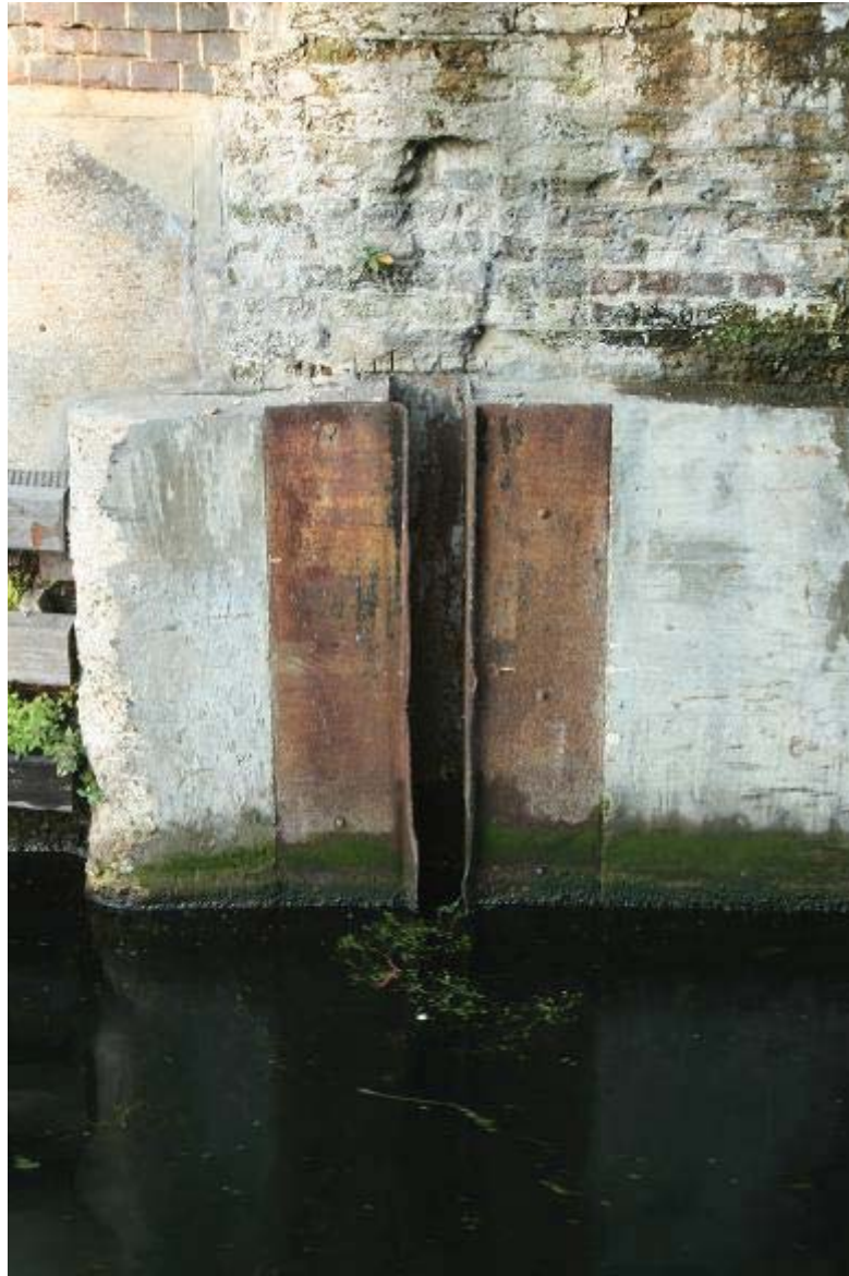
Plate 56 View of stock groove on east chamber, Old Ford Locks, looking west: OL- 05007
