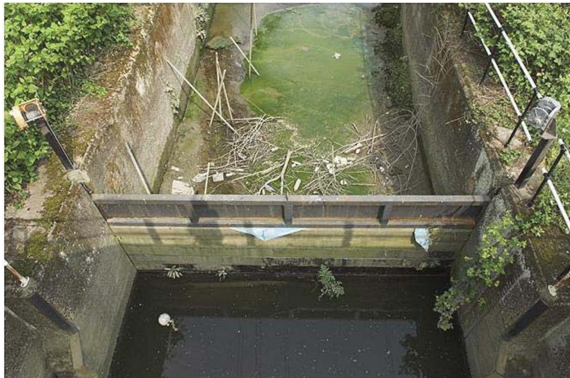
Plate 76 View of modern tide gate with associated machinery, Carpenter's Lock, looking north-east: OL-03007
