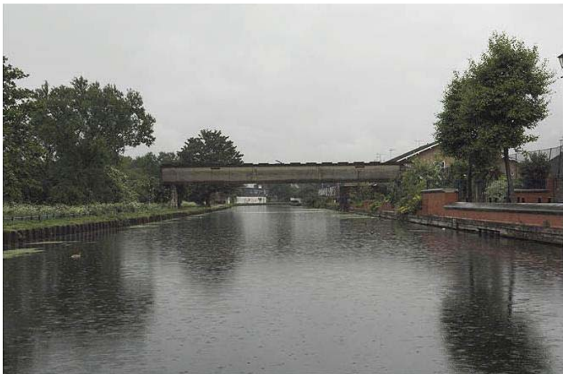
Plate 12 View of Lea Navigation and covered footbridge, looking south: OL-01207
