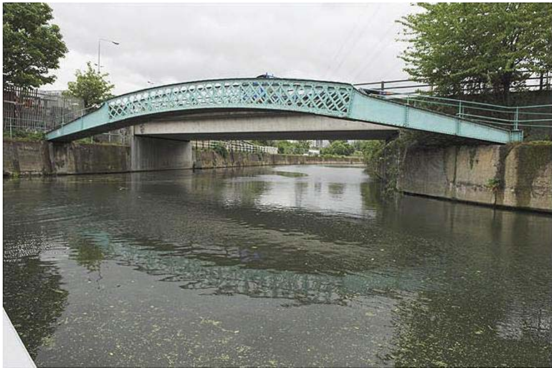
Plate 26 View of City Mill River footbridge with Marshgate Lane road bridge in background, looking north-east: OL-03507
