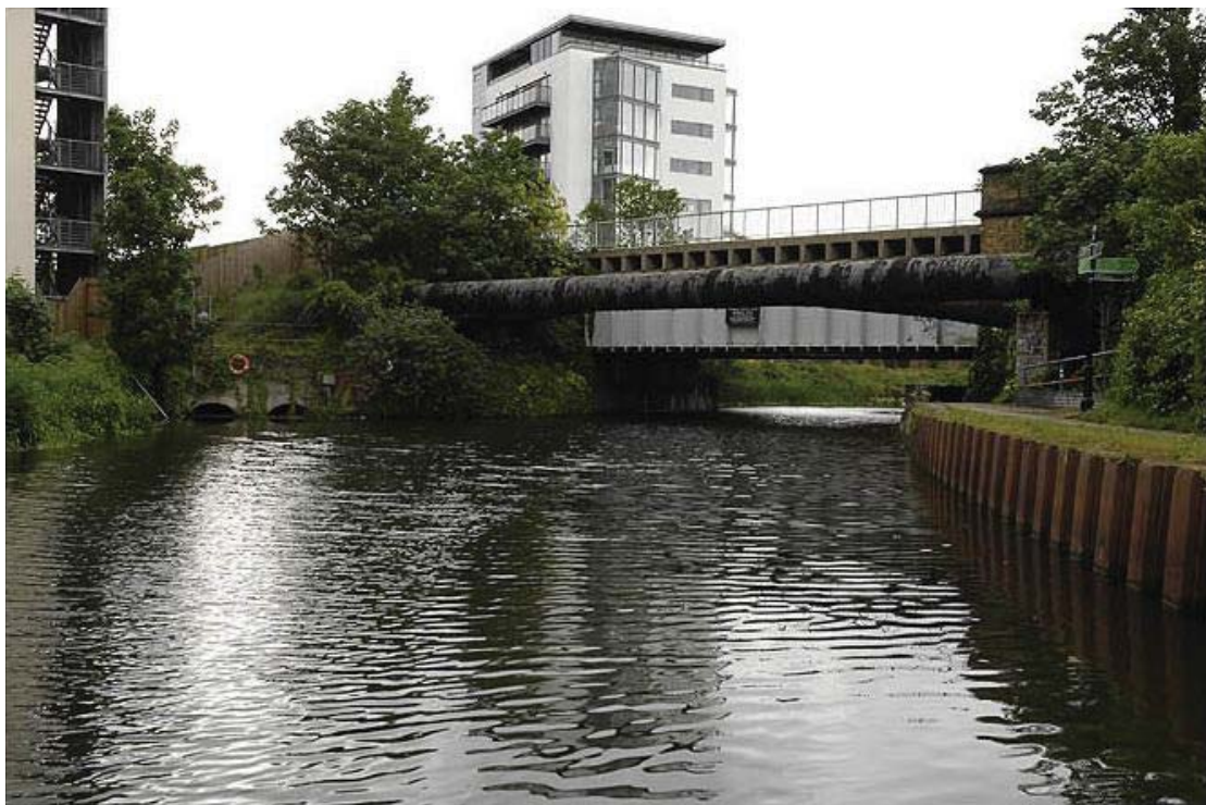
Plate 19 View of Greenway bridge spanning the River Lea with sewage pipes on foreground, looking north-west: OL-01207
