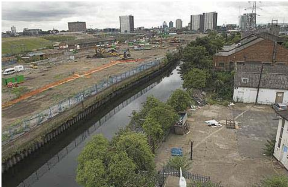
Plate 40 View of the Waterworks River from Marshgate Lane road bridge, looking south-east: OL-01207
