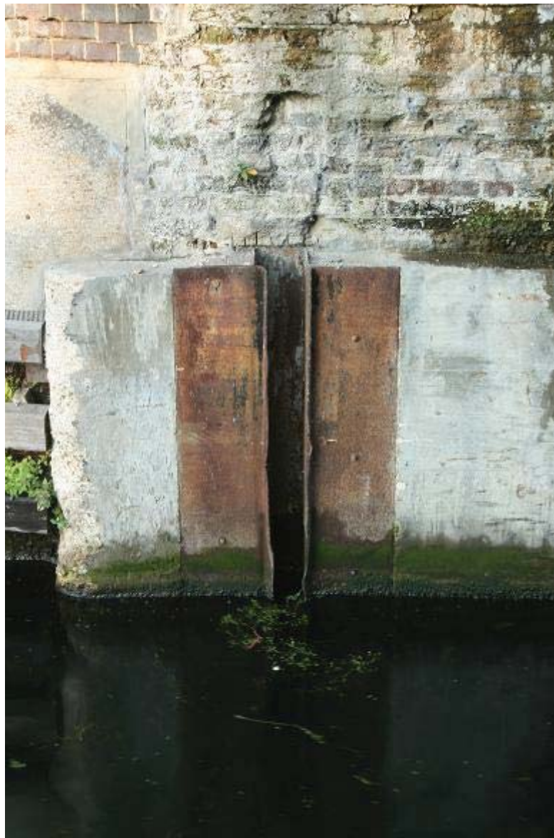
Plate 56 View of stock groove on east chamber, Old Ford Locks, looking west: OL- 05007
