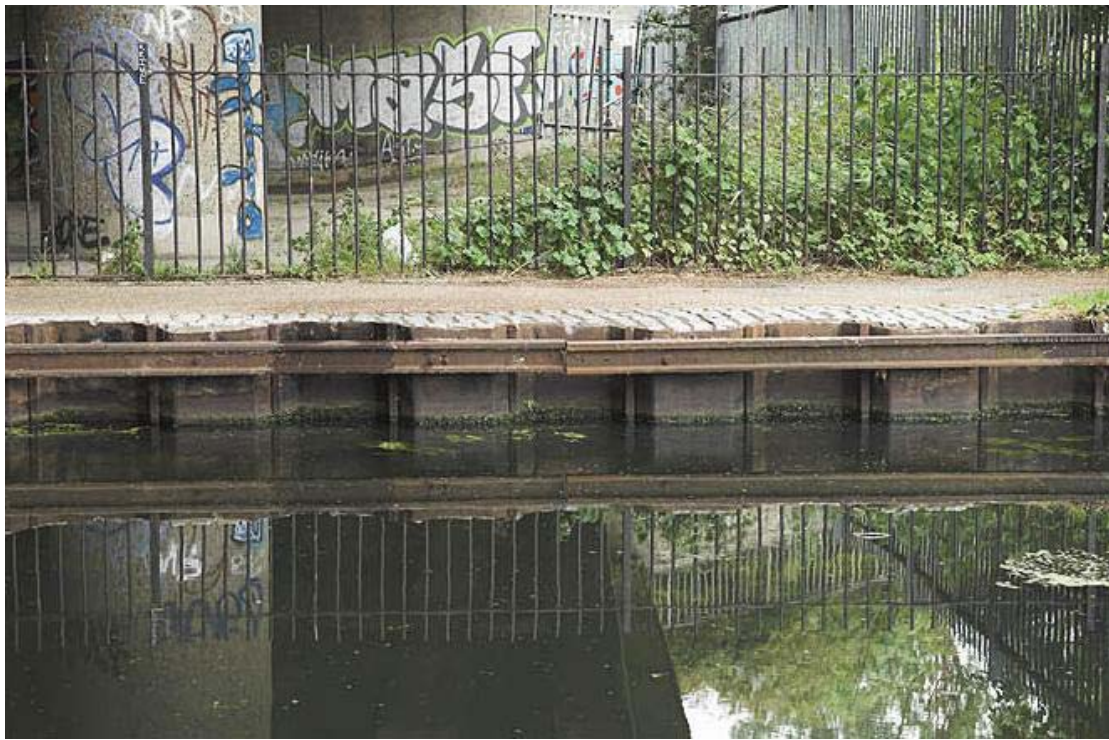
Plate 15 View of Lea Navigation's east bank showing Larsen camp sheeting with metal bracketing and cobbled capping: OL-01207
