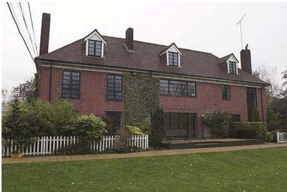
Plate 41 Oblique view of south elevation of Old Ford Lock Houses, looking north-northeast: OL-07307
