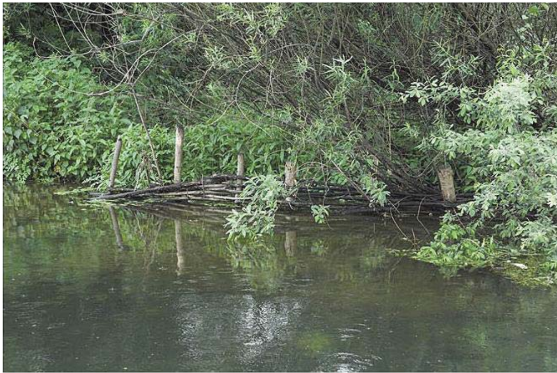
Plate 20 View of wattling on the west bank of the River Lea, looking west: OL-01207
