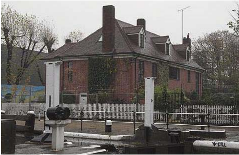
Plate 44 View of west elevation of Old Ford Lock Houses with Old Ford Locks in foreground, looking east: OL-07307
