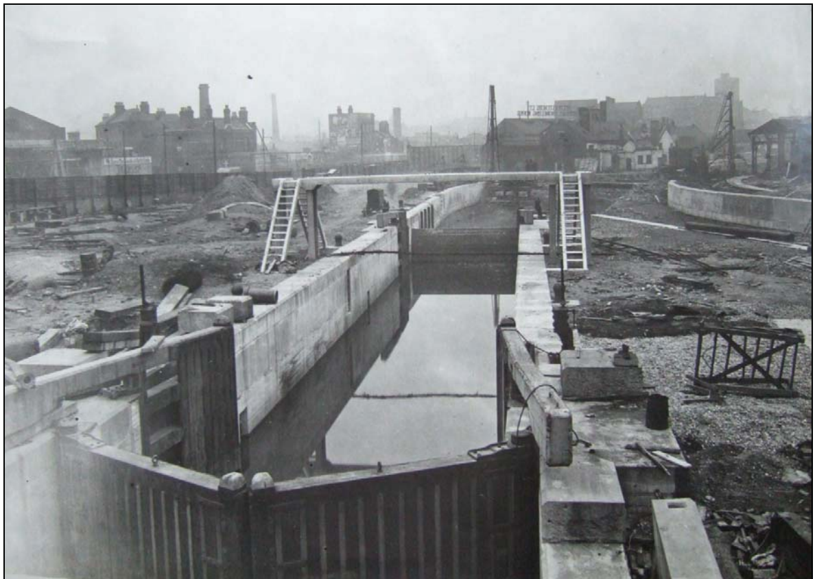
Plate 3 Setting out of the flood channel (sloping poles show position of the future concrete revetments), May 1930: OL-01207
