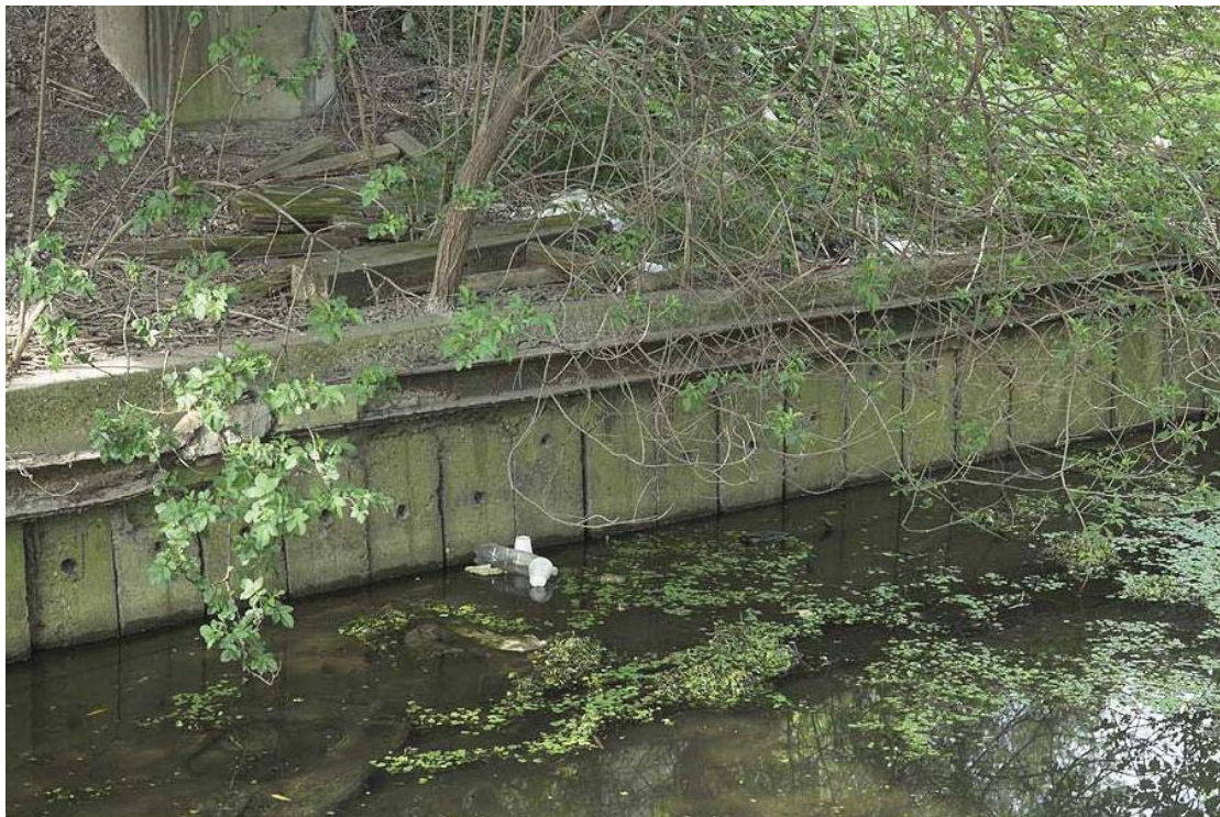
Plate 37 View of concrete pile west bank of Pudding Mill River, looking south-west: OL-01207
