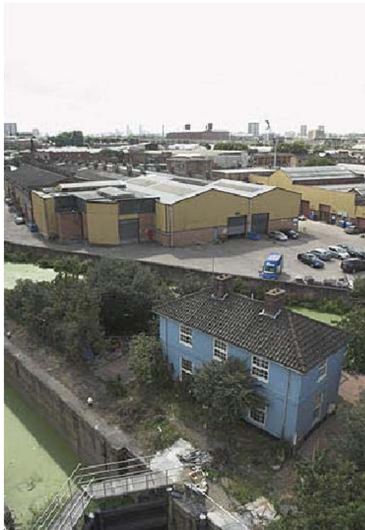
Plate 65 View of Marshgate Lane Lock House, looking south-west: OL-07407
