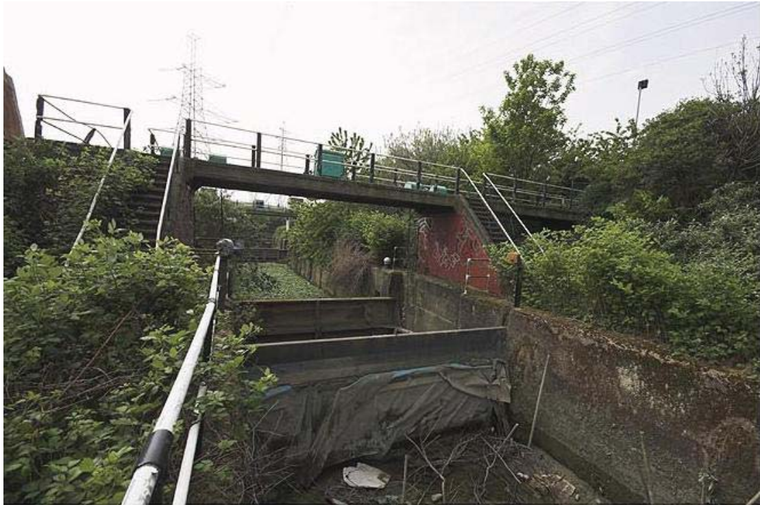
Plate 78 View of north end of Carpenter's Lock, looking south: OL-03007
