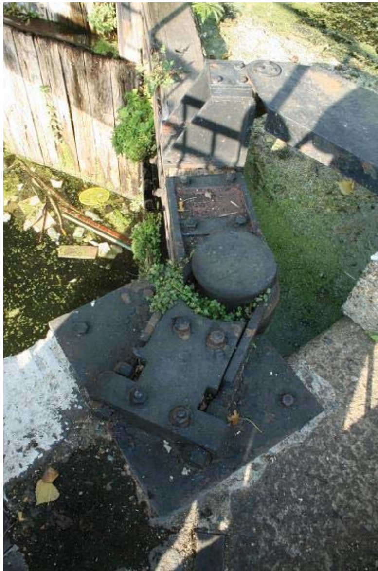
Plate 53 Detailed view of mechanism and hinge of the west chamber's south gate, Old Ford Locks: OL-05007
