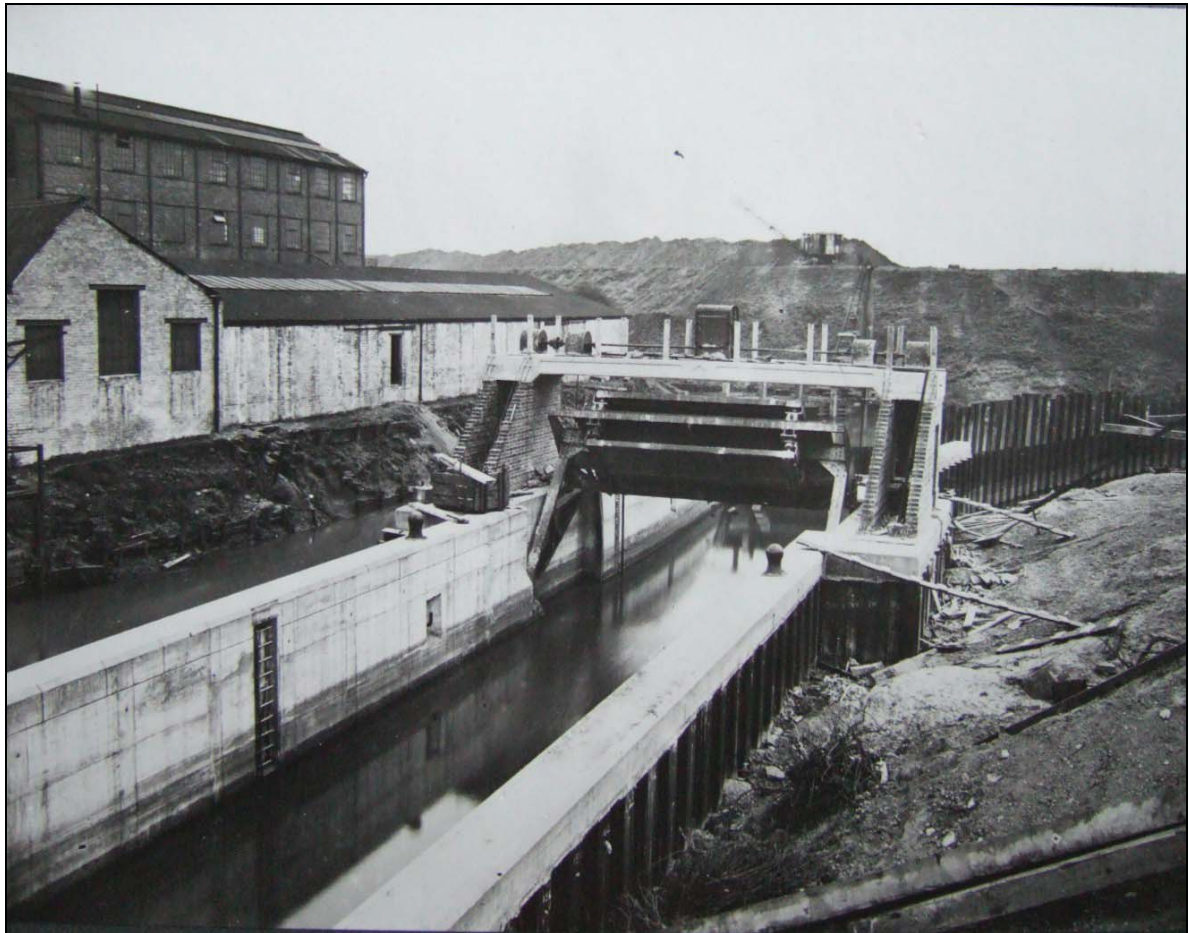
Plate 5 View of new lock near Carpenter's Road bridge (Carpenter's Lock), 1934 (LD PEM PS 159/0818, courtesy of Newham Local Studies and Archive Library): OL-03007
