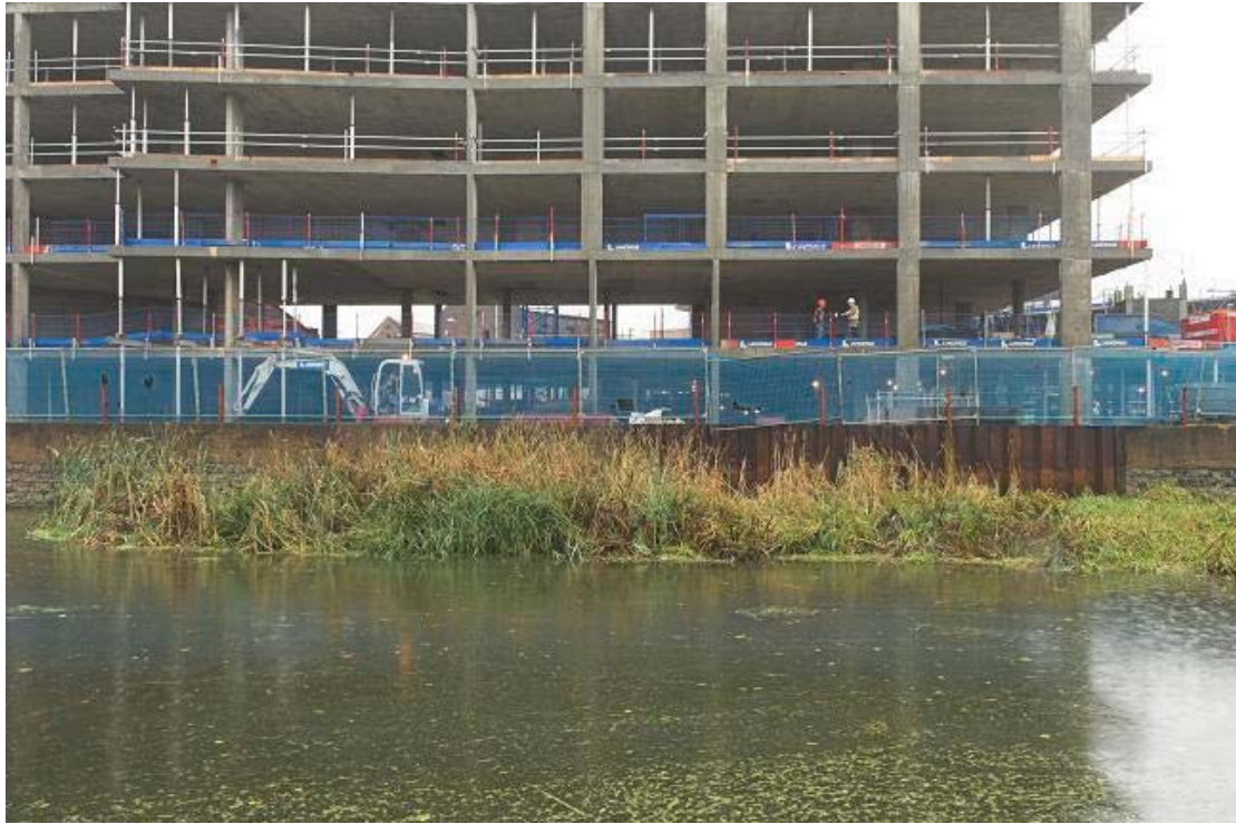
Plate 68 View of possible wharf entrance, stone and brick riverbank wall, looking southwest: OL-07207
