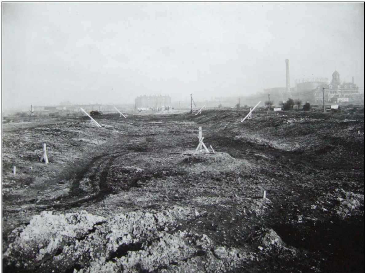
Plate 3 Setting out of the flood channel (sloping poles show position of the future concrete revetments), May 1930: OL-01207
