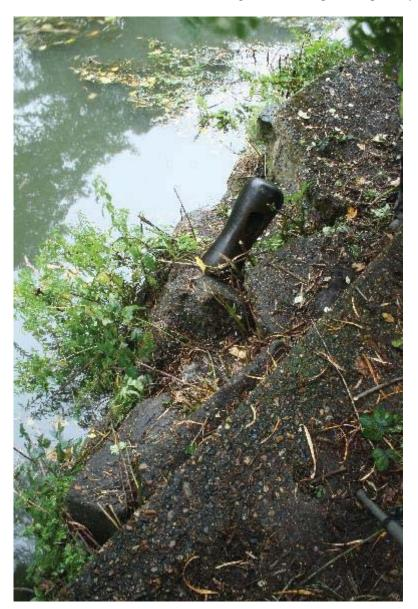
Plate 61 Detailed view of damaged eastern wing wall with metal mooring post, Pudding Mill River, looking north-northwest: OL-05407
