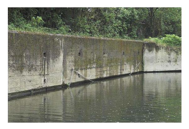
Plate 21 View of the east bank of the River Lea showing imprints of timber shuttering and sockets for mooring rings, looking south-west: OL-01207
