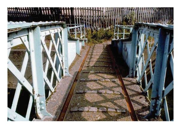
Plate 83 Detailed view showing granite set risers and inset open ceramic drainpipes, City Mill River Footbridge, looking north-east: OL-03507
