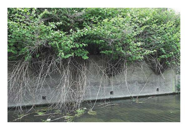
Plate 27 View of west bank of City Mill River with row of drainage holes immediately above waterline, looking west: OL-01207
