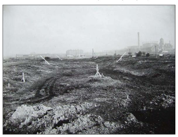
Plate 3 Setting out of the flood channel (sloping poles show position of the future concrete revetments), May 1930: OL-01207
