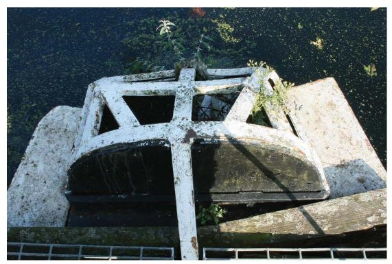
Plate 49 Detailed view of navigation lamp on northern tip of Old Ford Locks dolphin, looking north: OL-05007
